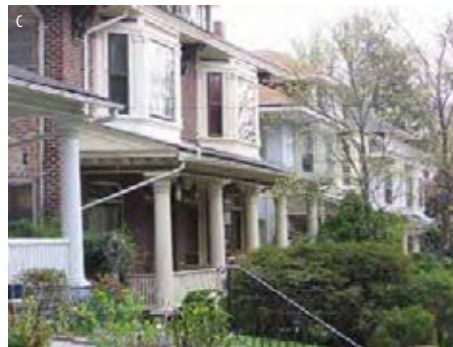
A Burrows Farmhouse, Verplank Street, NW B Naylor Court alley building, NW C Porch fronts, ???Location?
