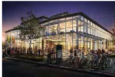
A Capital Bike Share Station B The Lumber Shed, 301 Water Street SE, before and proposed rendering of adaptive reuse
