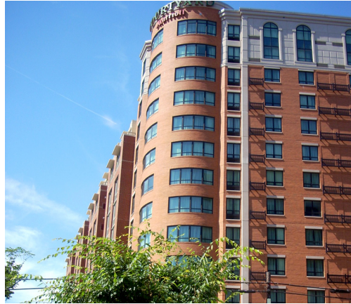
Courtyard Marriott, 140 L Street, SE
