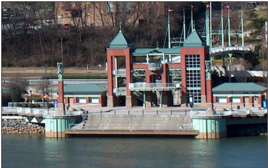
Example of boathouse in Knoxville, TN
