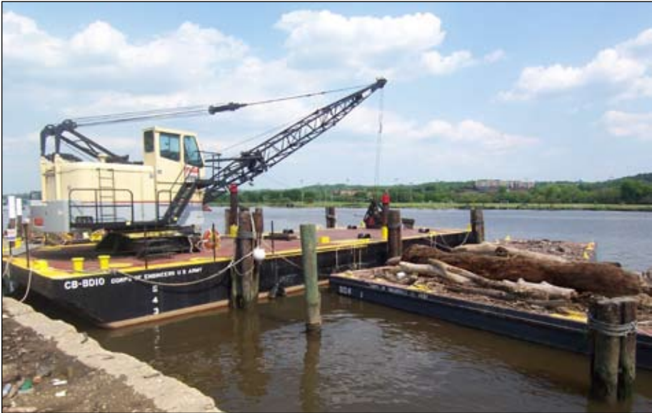
USACE debris removal facility
