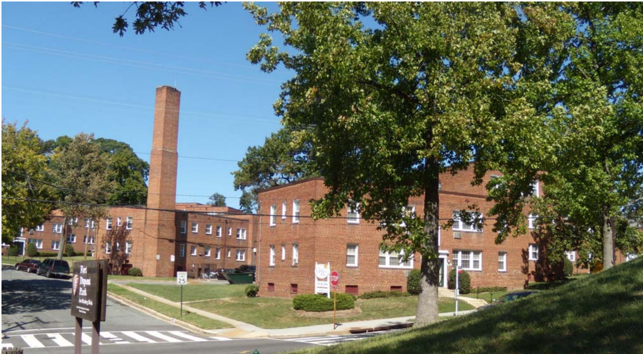
Multi-family residential uses located on the north side of Ely Street SE
