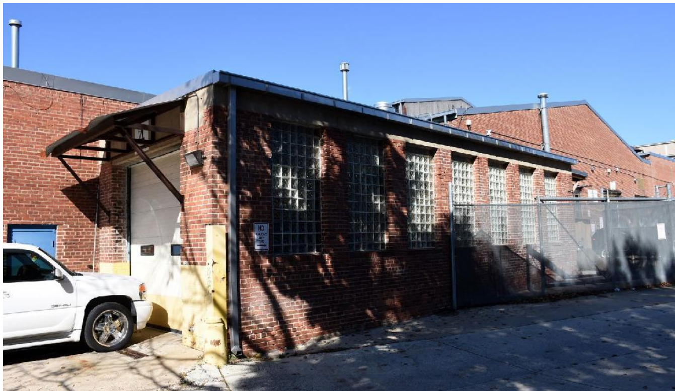
13. South addition – south façade facing alley showing glass block infill.
