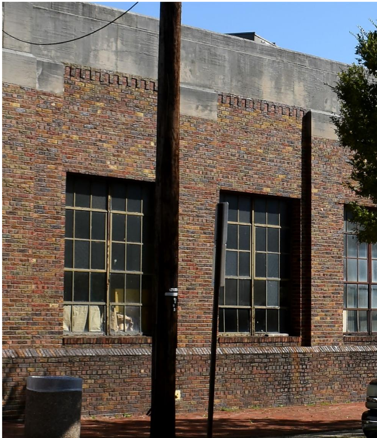
6. West (44 th Street) façade – window apertures showing steel sashes.
