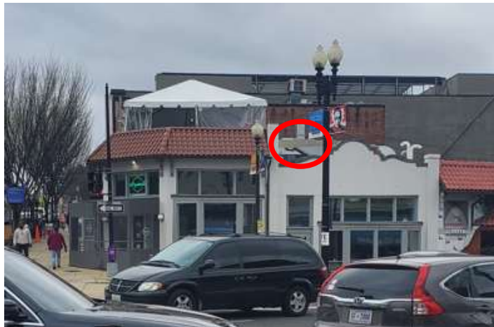
Approved stair towers circled in red with restaurant equipment in front
