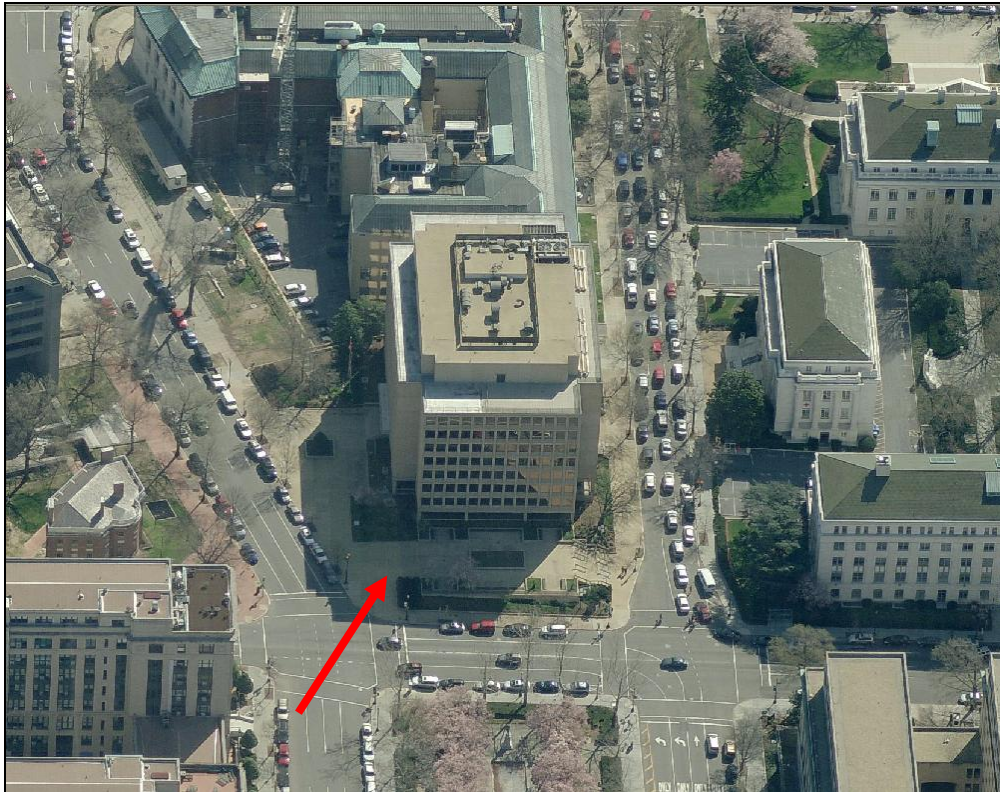
Aerial view of the site looking east across 18 th Street
