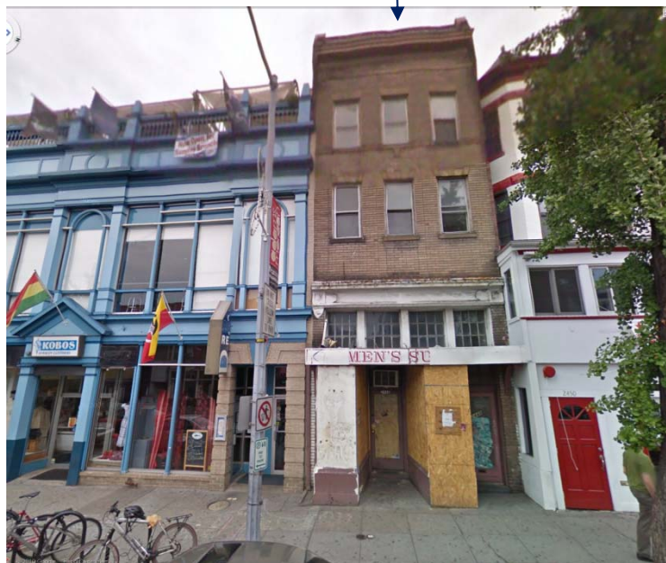
Zoning and vicinity map, with photo of existing condition - 2448 18 th St NW.
