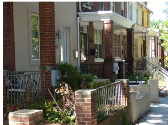
Adjacent residential uses on Euclid Street NW
