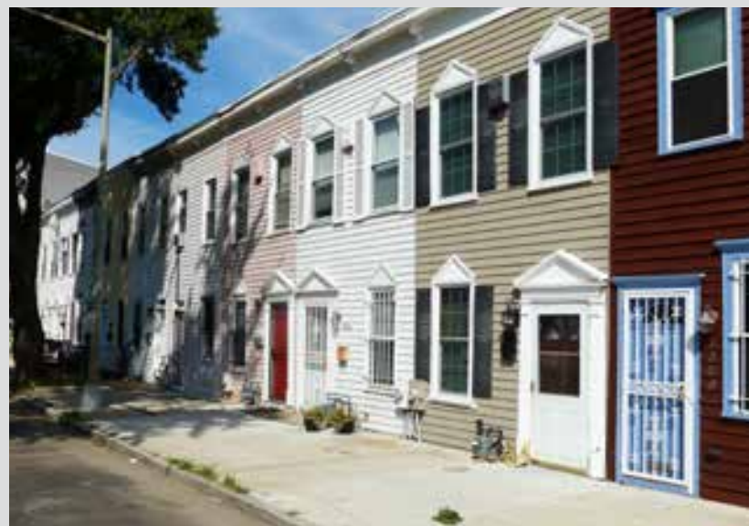
Early frame houses in Rosedale
