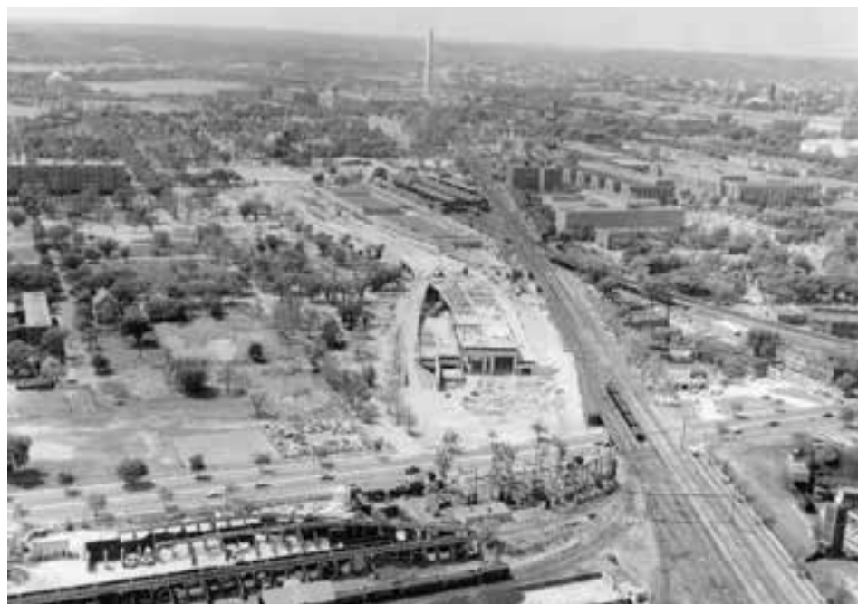
New freeway begins to rise on cleared land in Southwest District Department of Transportation
