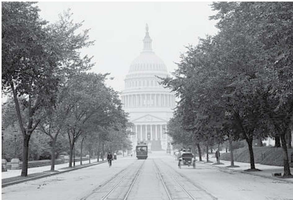
Streetcar along East Capitol Street, showing underground electrical conduit installed in 1884 Library of Congress
