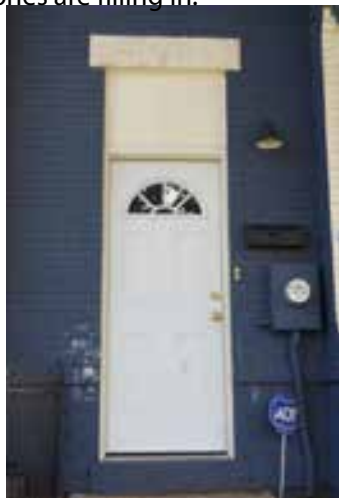
Transom window filled in with solid panel
