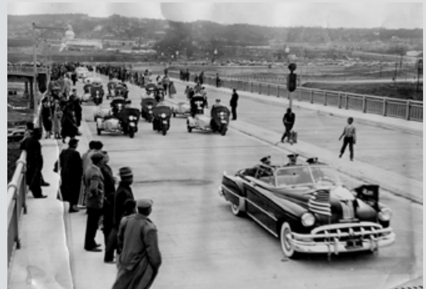
Opening of the Douglass Memorial Bridge connecting Southwest across the Anacostia River, courtesy DDOT
