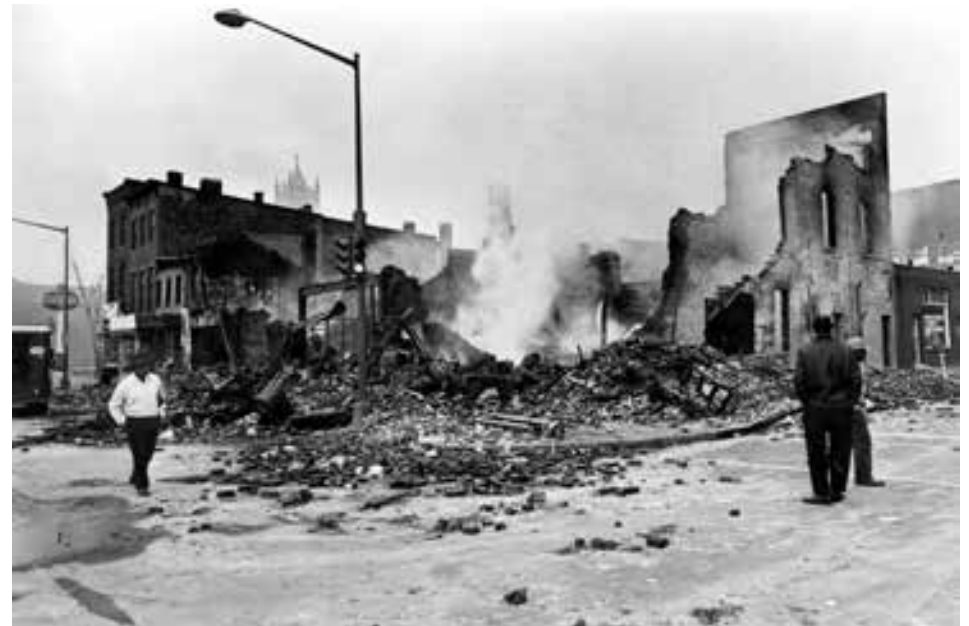
Burned out buildings at 7th Street NW
