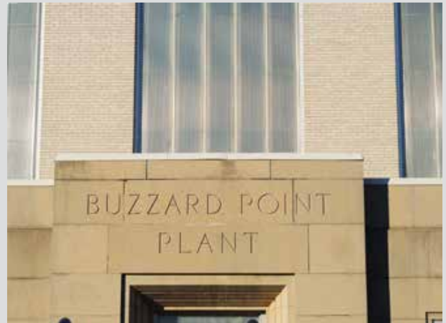
Buzzard Point Power Plant, courtesy H. Wetzel
