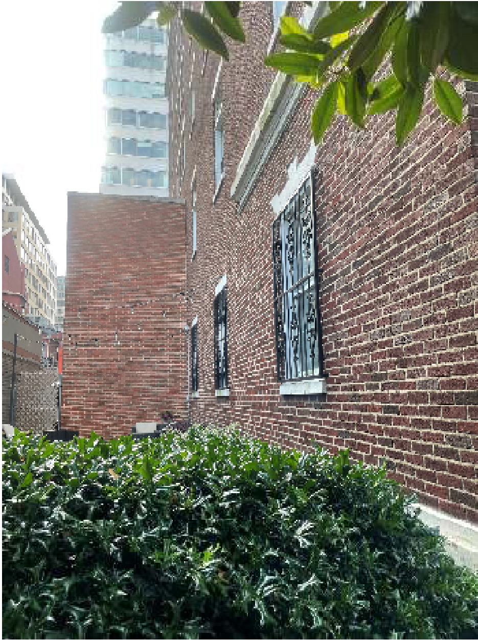
Photo 04: North elevation looking east
