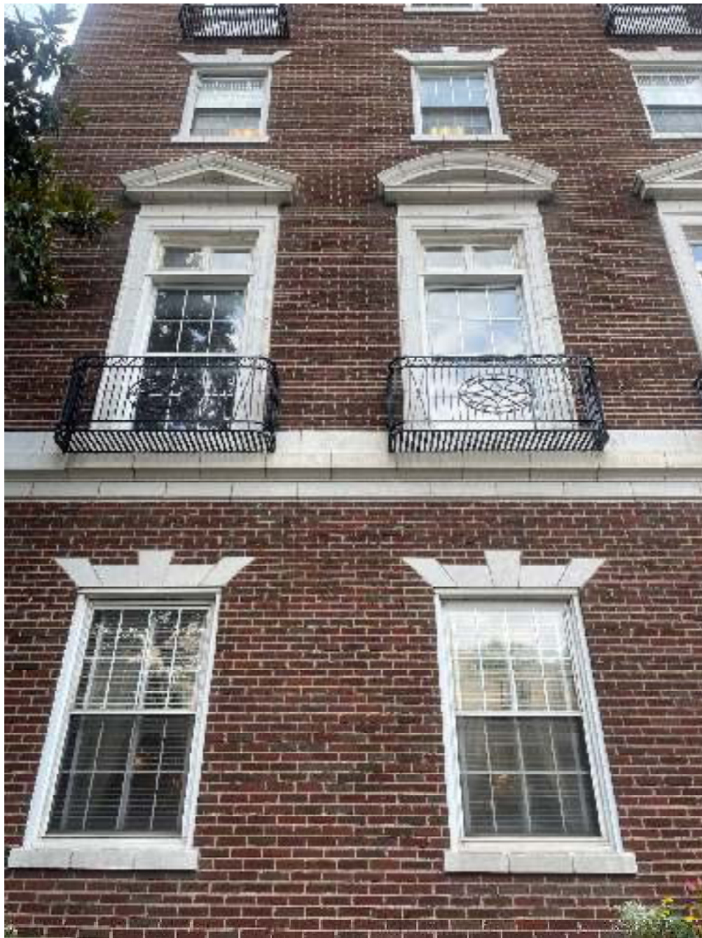
Photo: 10: Close up of windows on façade (west elevation) looking west
