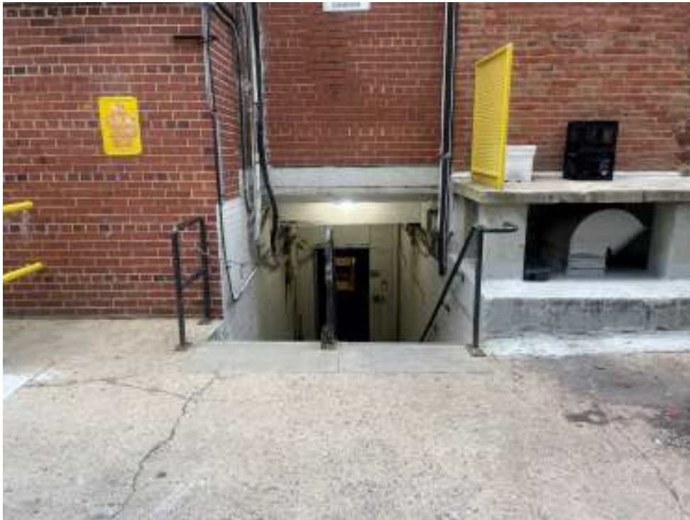
Figure 07: Basement egress door on east (rear) elevation looking west
