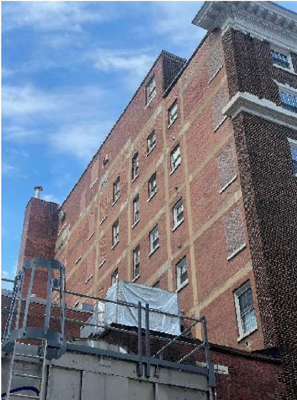
Photo 05: East (rear) elevation looking southwest
