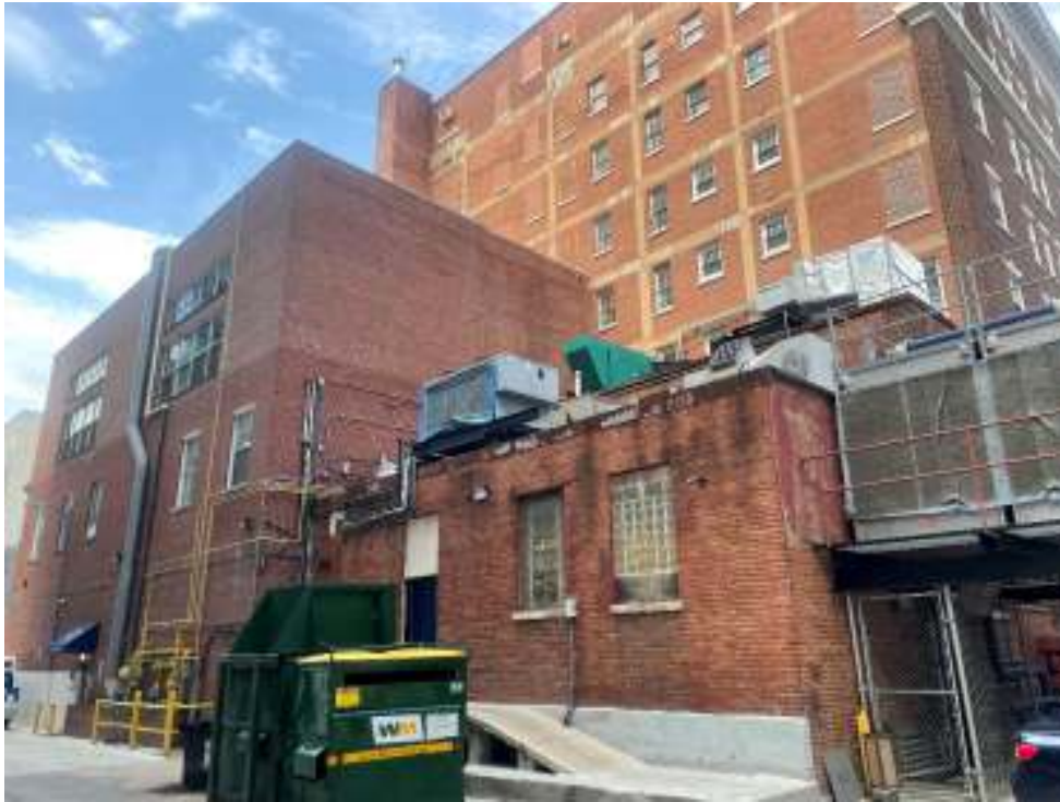
Figure 06: East (rear) elevation looking southwest
