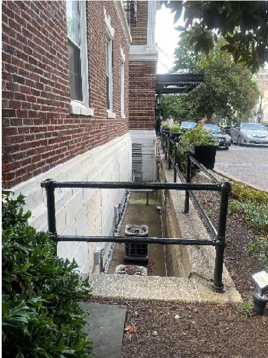
Figure 08: Areaway in front of building, looking south
