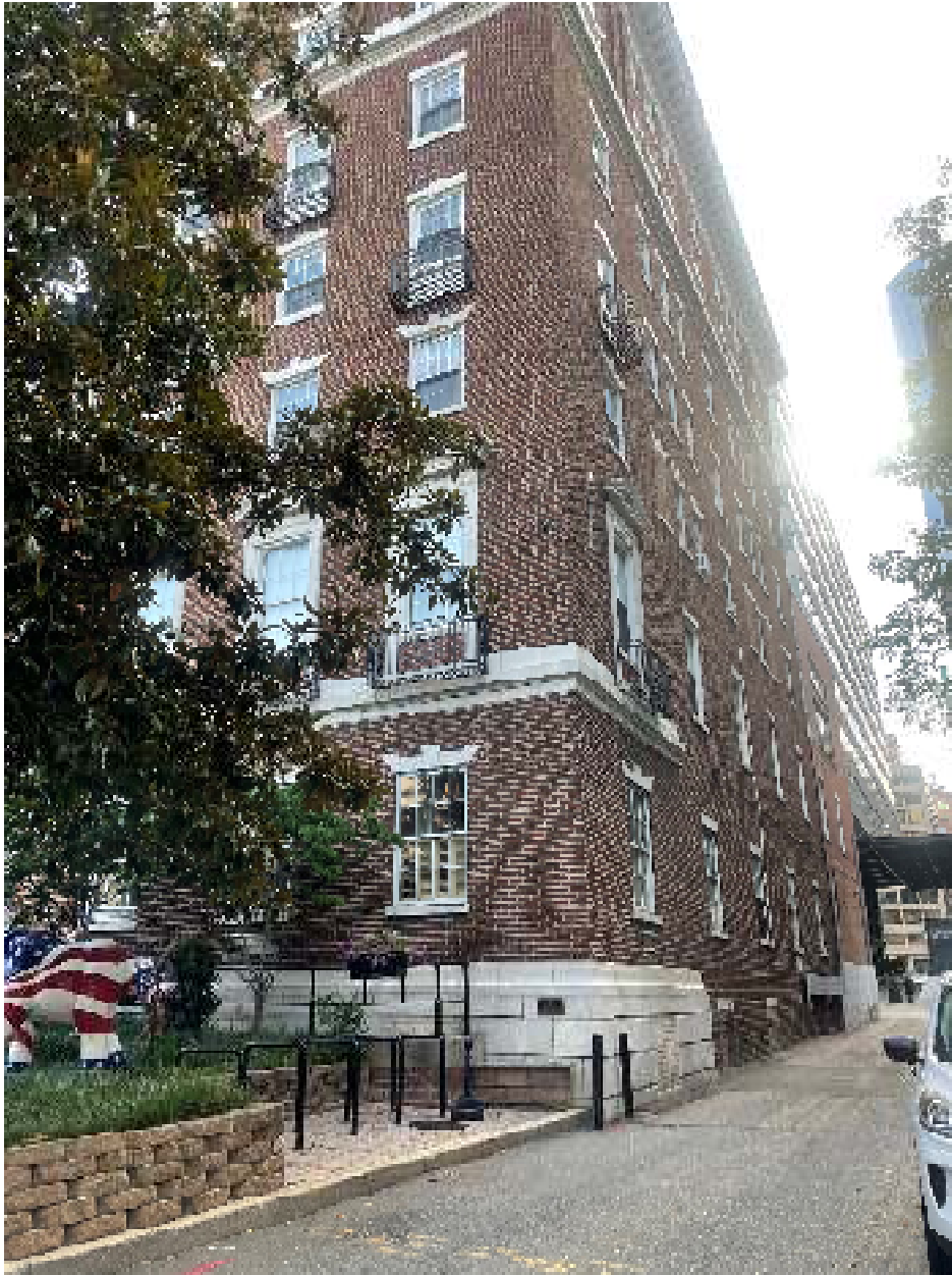
Photo 02: South and west elevation, looking northeast
