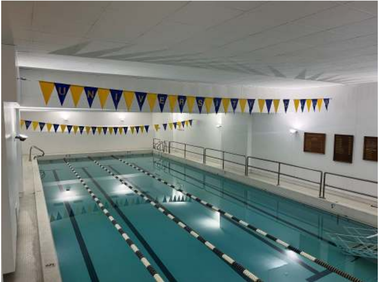
Photo 21: View of pool at basement level looking east
