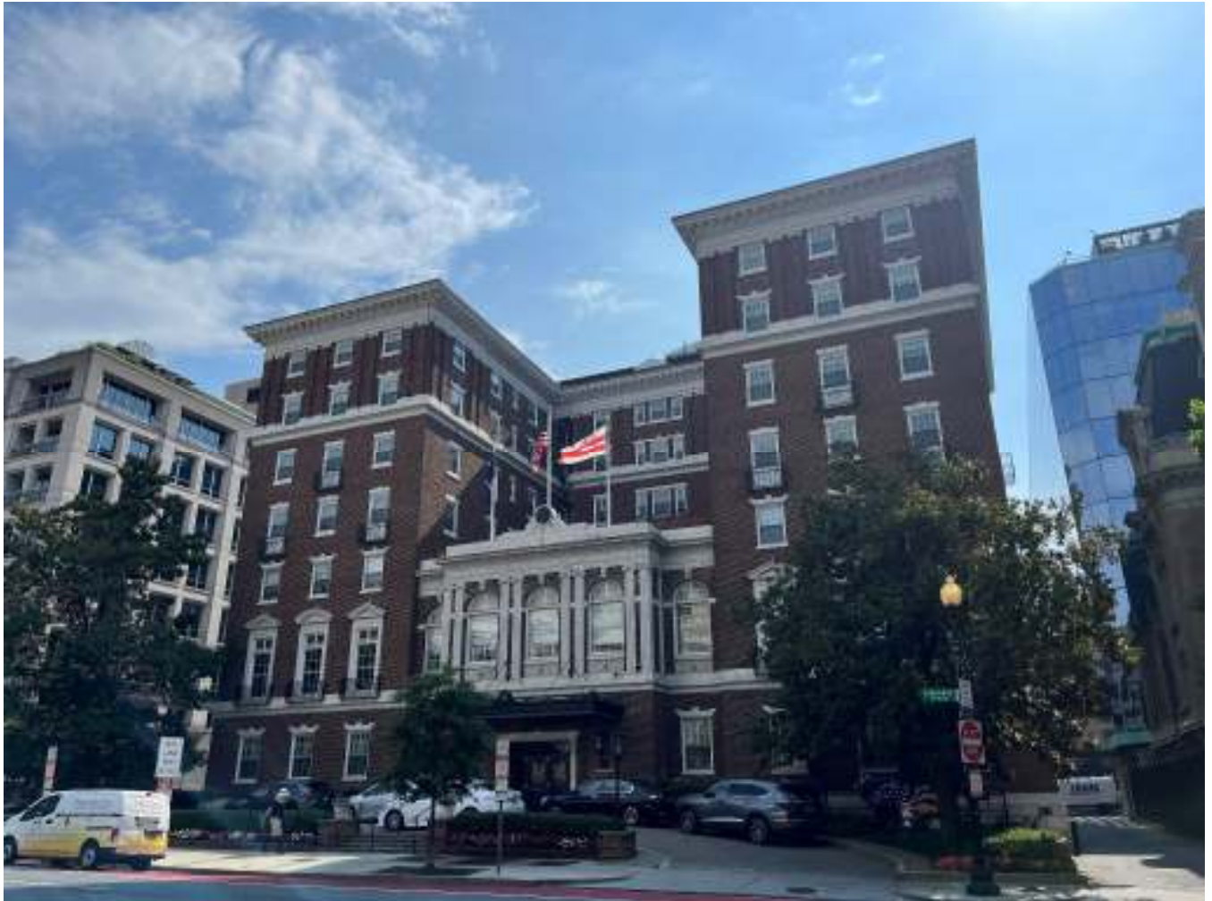
Photo 01: Façade (west elevation), looking northeast
