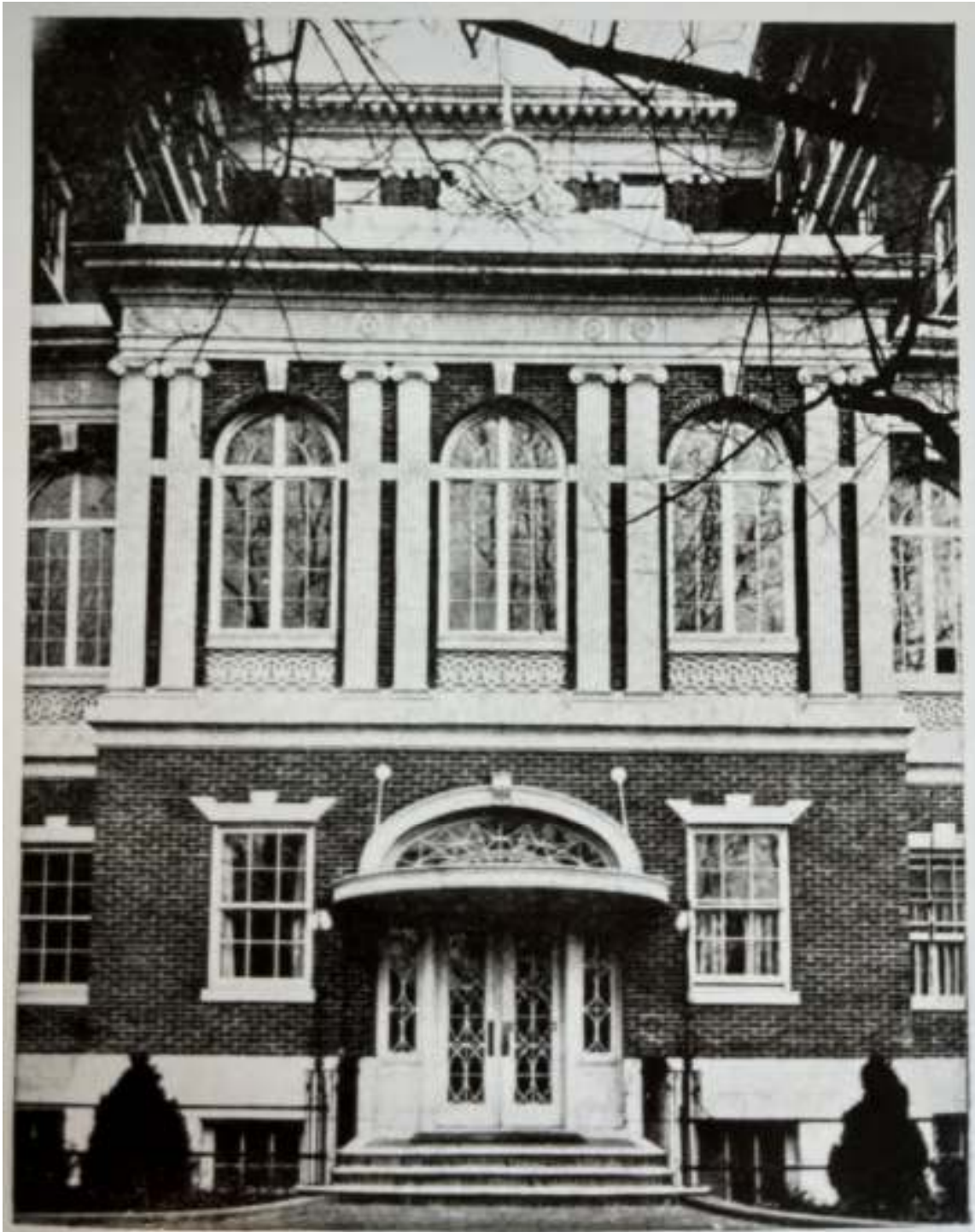
Figure 10: Undated view of detail on terra cotta on façade of 1135 Sixteenth Street NW, looking W. DC History Center .
