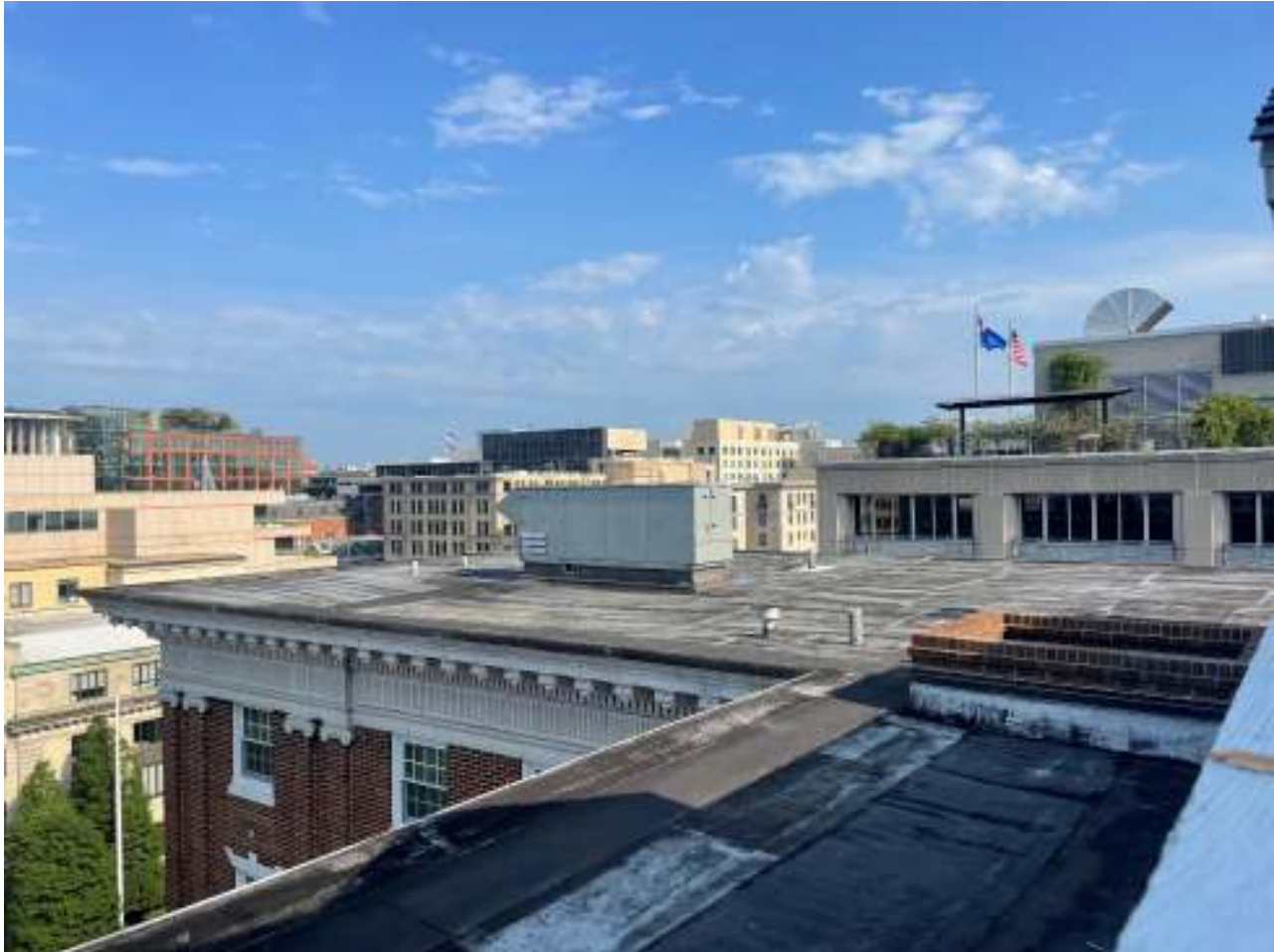
Photo 21: View of rooftop looking northwest
