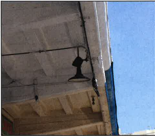
Existing light fixtures and locations at 5th Street.
