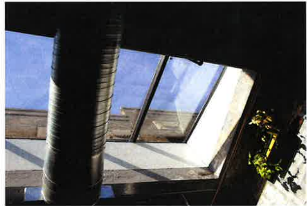
Example of re-opened skylight.
