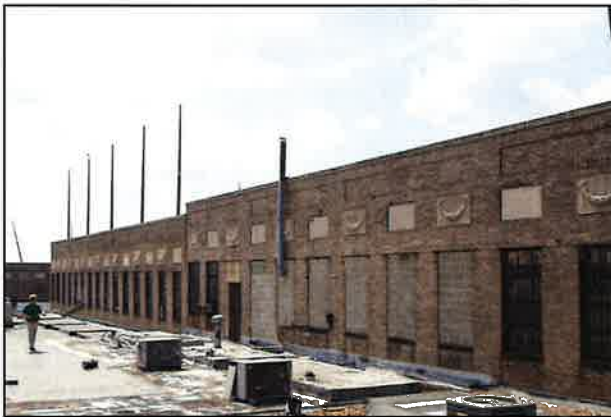
Existing cornice conditions.
