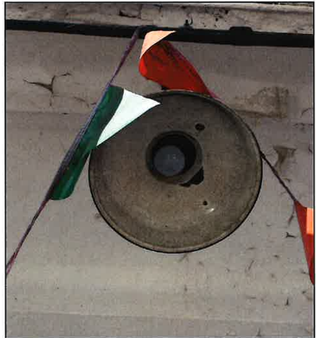
Existing light fixture at 5th Street.
