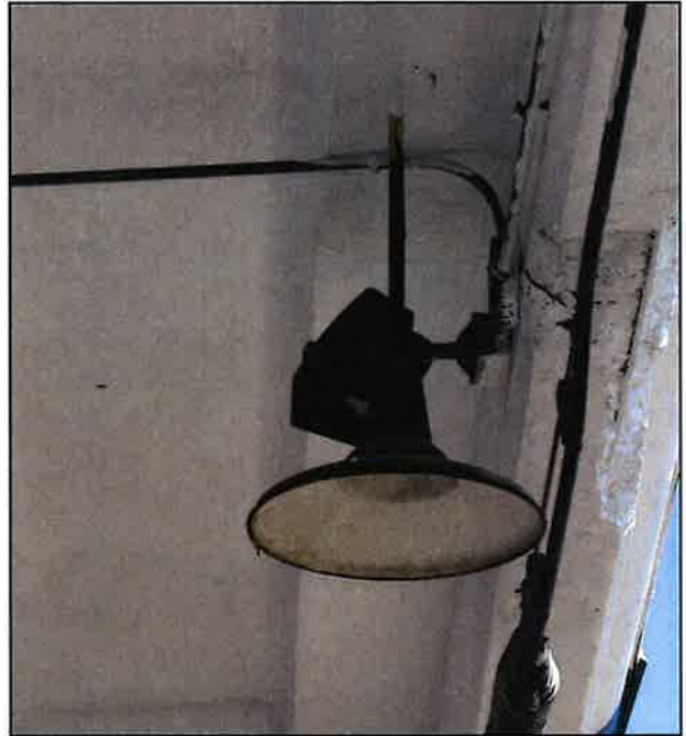
Existing light fixture at 5th Street.
