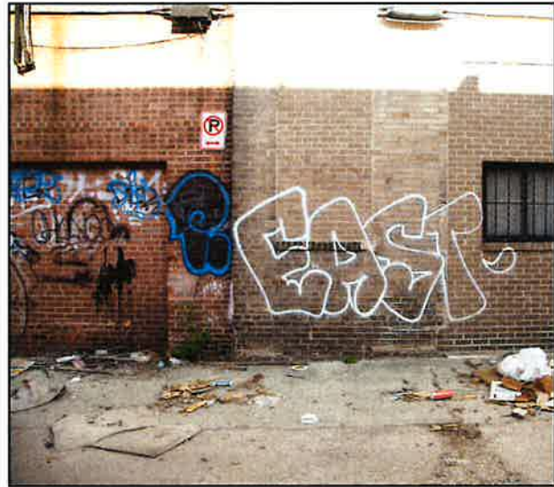
Existing typical masonry wall.
