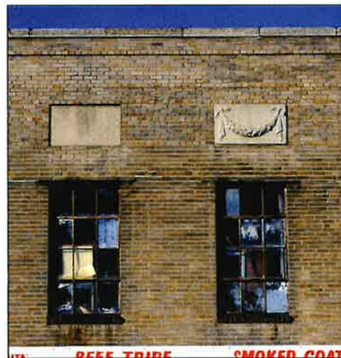
Existing original window detail.
