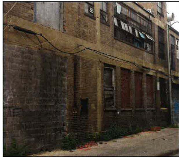
Existing typical wall at rear alley.
