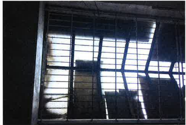
Image of original skylight.
