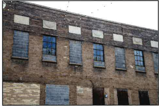
Existing window and panel conditions.
