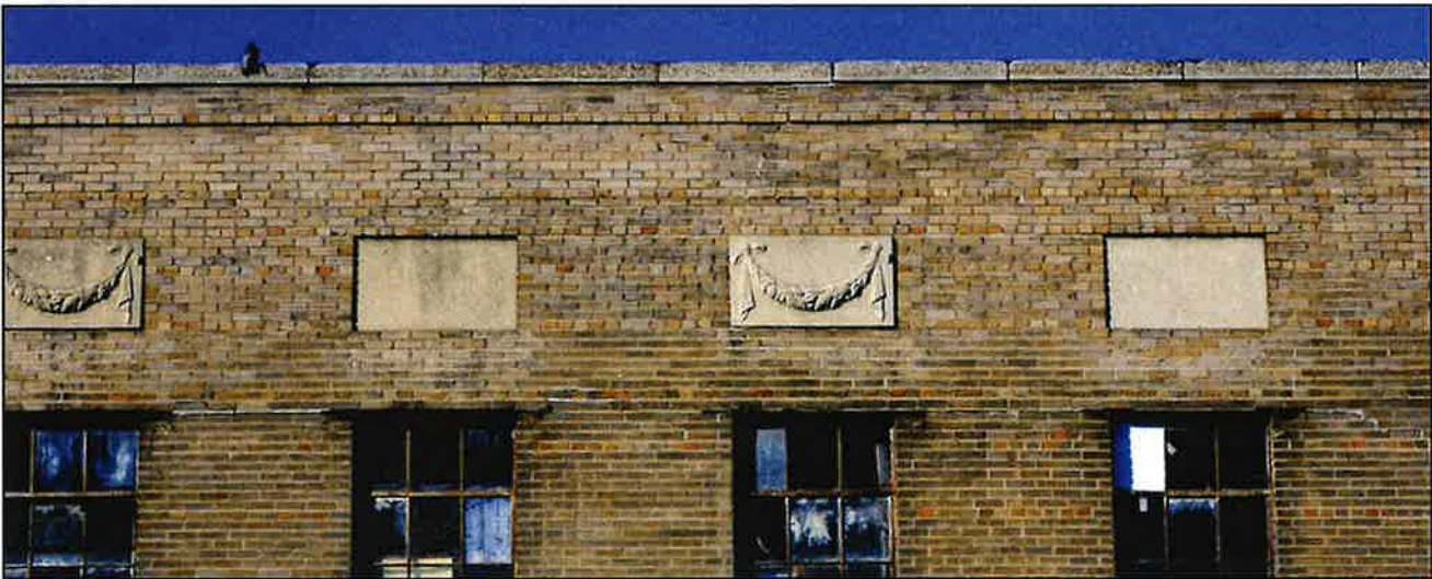
Existing window and panel conditions.
