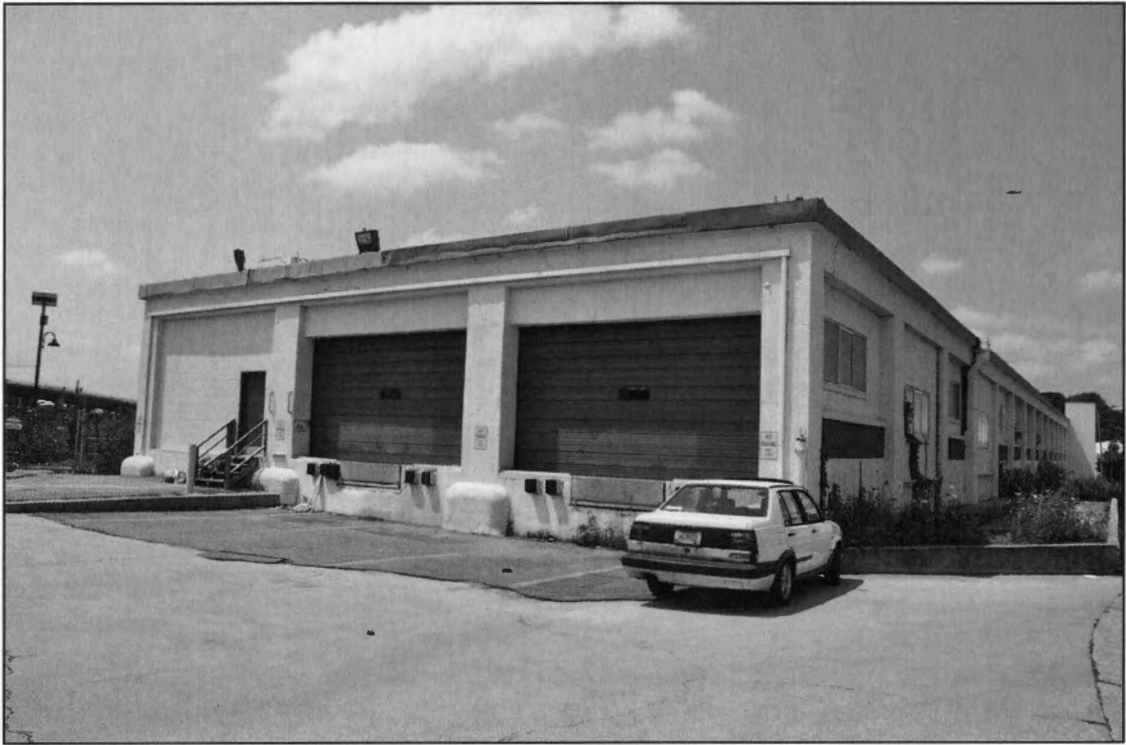
PHOTO 5: View Northeast Elevation and Loading Dock, Looking South
