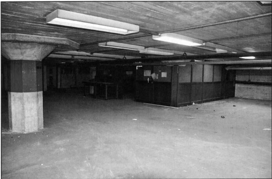
PHOTO 10: Basement, View of Storage Area
