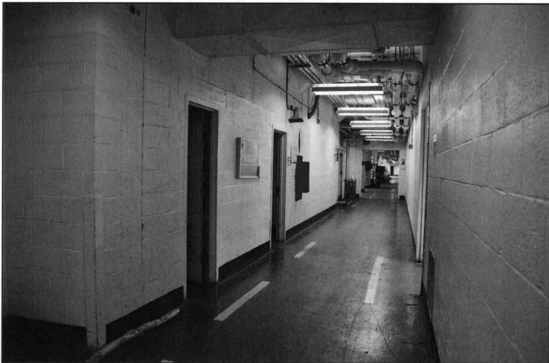
PHOTO 17: First Floor, Western Portion of Building, Corridor Adjacent to Cafeteria, Looking Southeast
