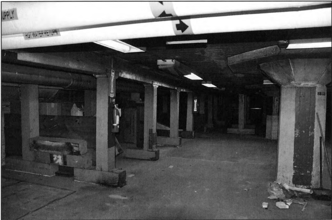
PHOTO 9: Basement, View of Storage Area, Wooden Supports
