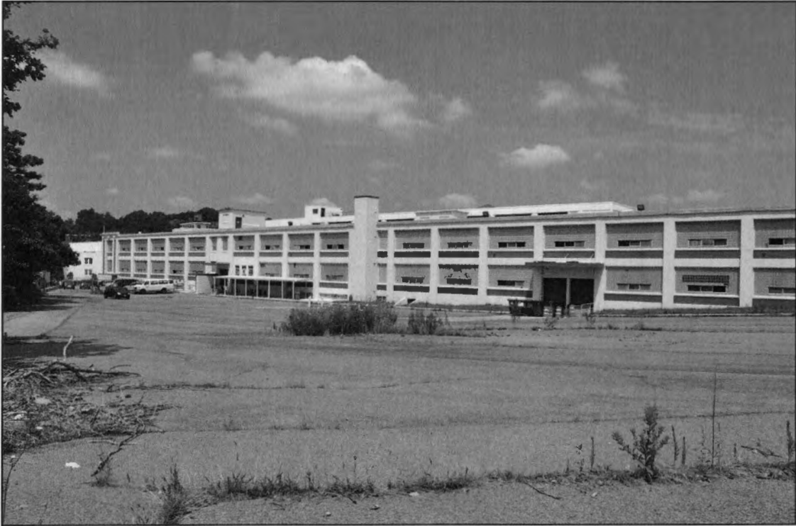
PHOTO 7: View of Southeast Elevation, Looking Northwest
