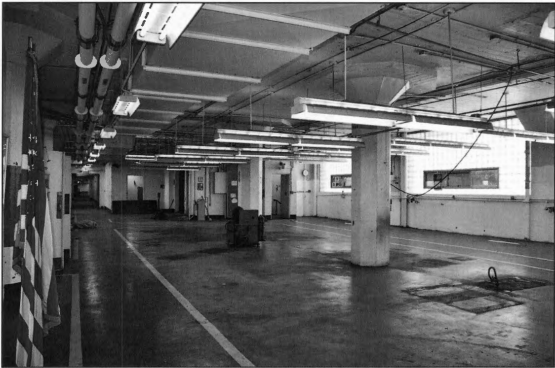
PHOTO 13: First Floor, Tool and Die Area, Looking East
