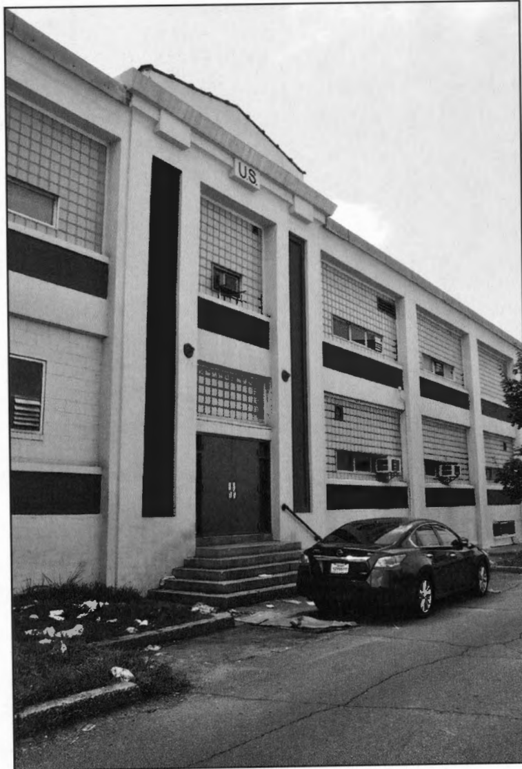
PHOTO 4: View of Original Main Entrance on Northwest Elevation, Looking Southwest
