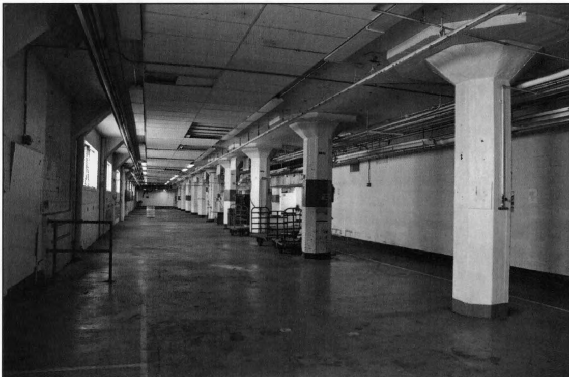
PHOTO 18: First Floor, View of Manufacturing and Storage Areas Looking Southeast Toward Press Room
