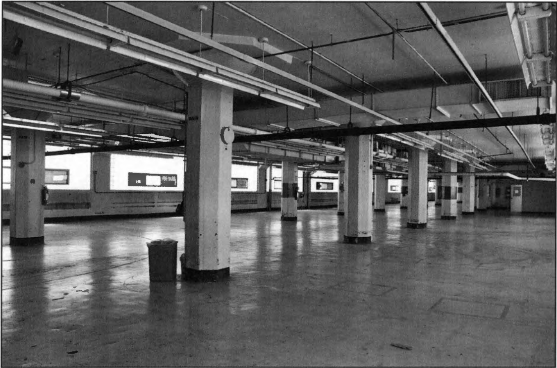
PHOTO 24: Second Floor, Key/Lock Manufacturing Area, Looking Southwest
