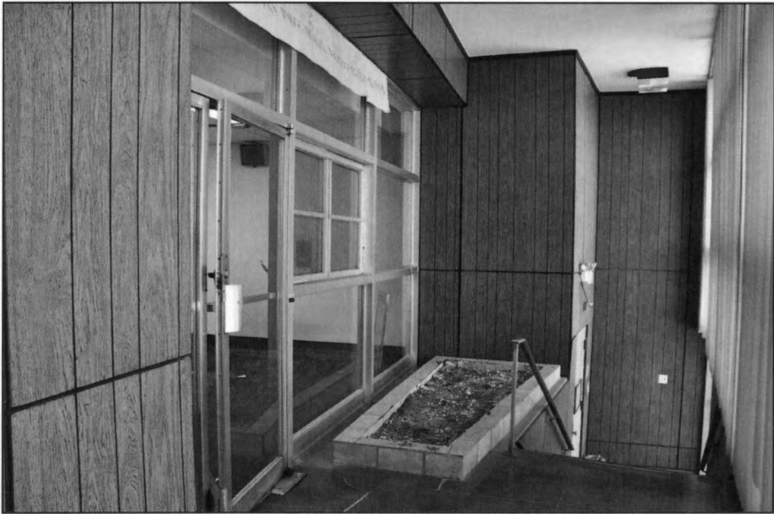
PHOTO 11: First Floor, Entrance Vestibule (ca. 1965) Looking South
