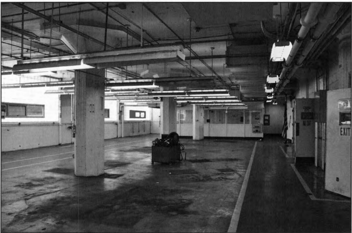
PHOTO 14: First Floor, Tool and Die Area, Looking West
