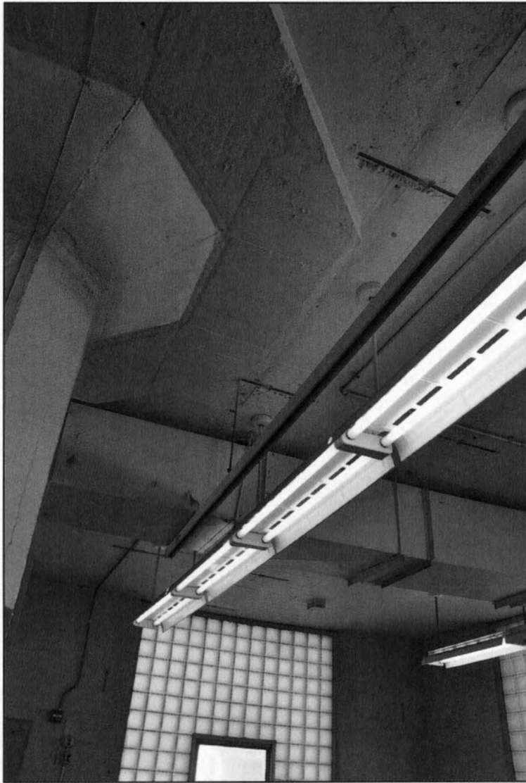
PHOTO 27: Second Floor, Lock Shop Area Ceiling Showing Original Keyways
