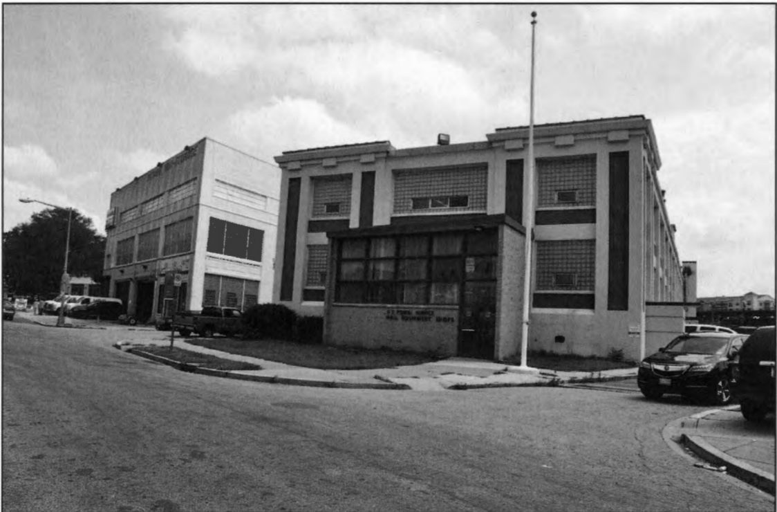
PHOTO 2: View of Southwest Elevation, Looking Northeast
