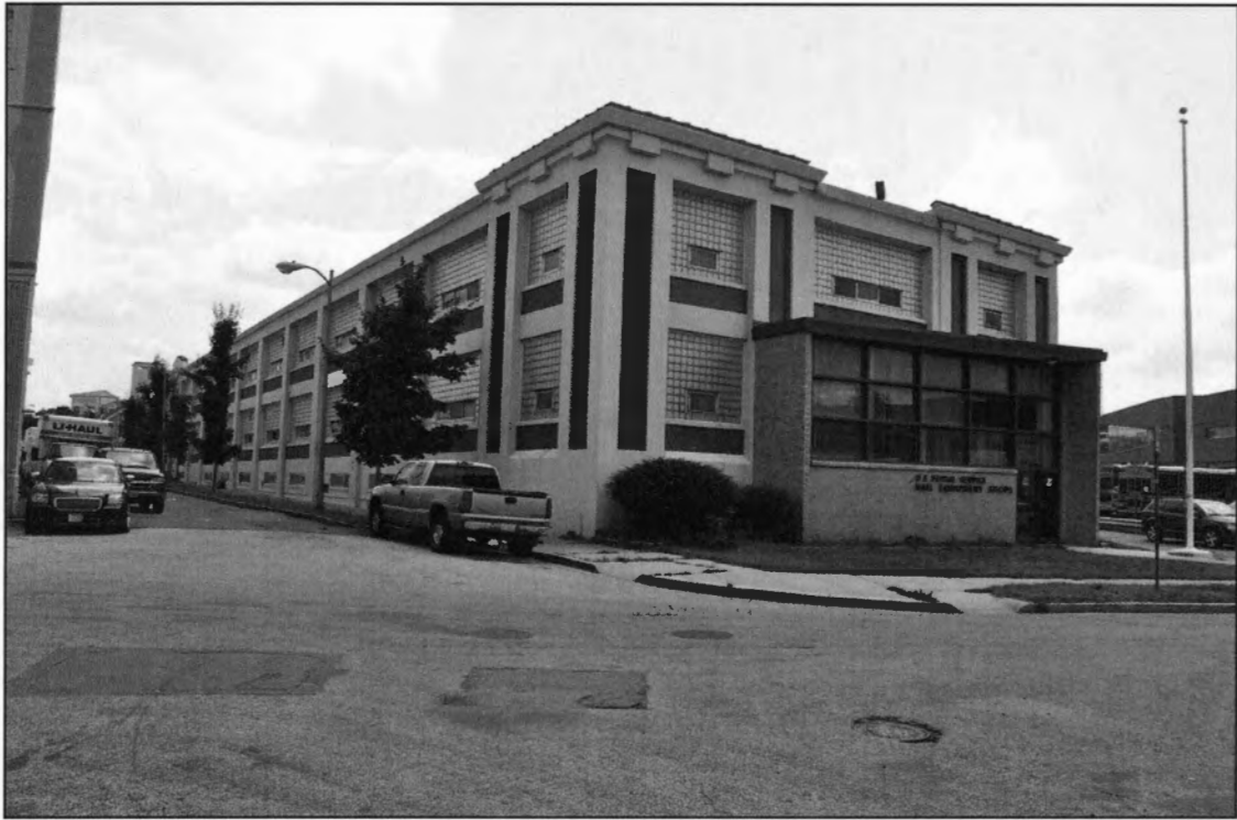
PHOTO 1: View of USPS Mail Equipment Shops, West Corner Looking East
