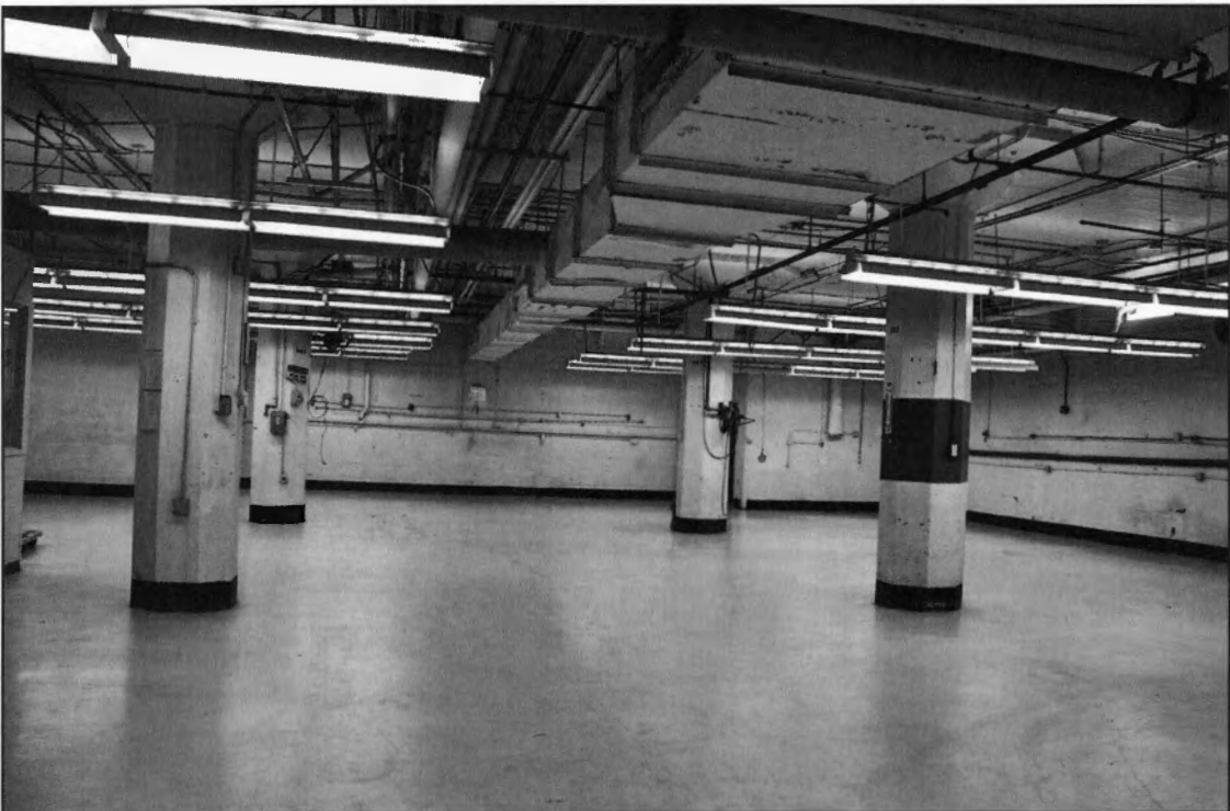
PHOTO 8: Basement, View of Maintenance Area
