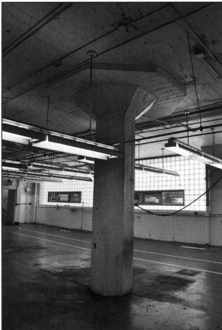
PHOTO 15: First Floor, Detail of Column
