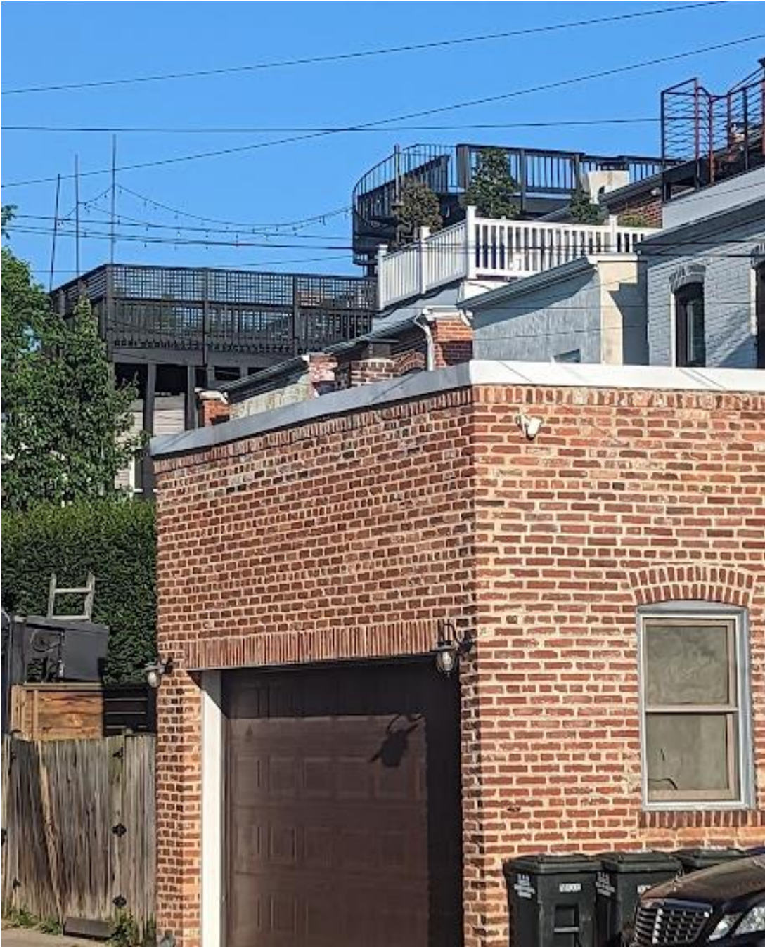
2: Existing Neighboring Roof Deck with Spiral Staircase
