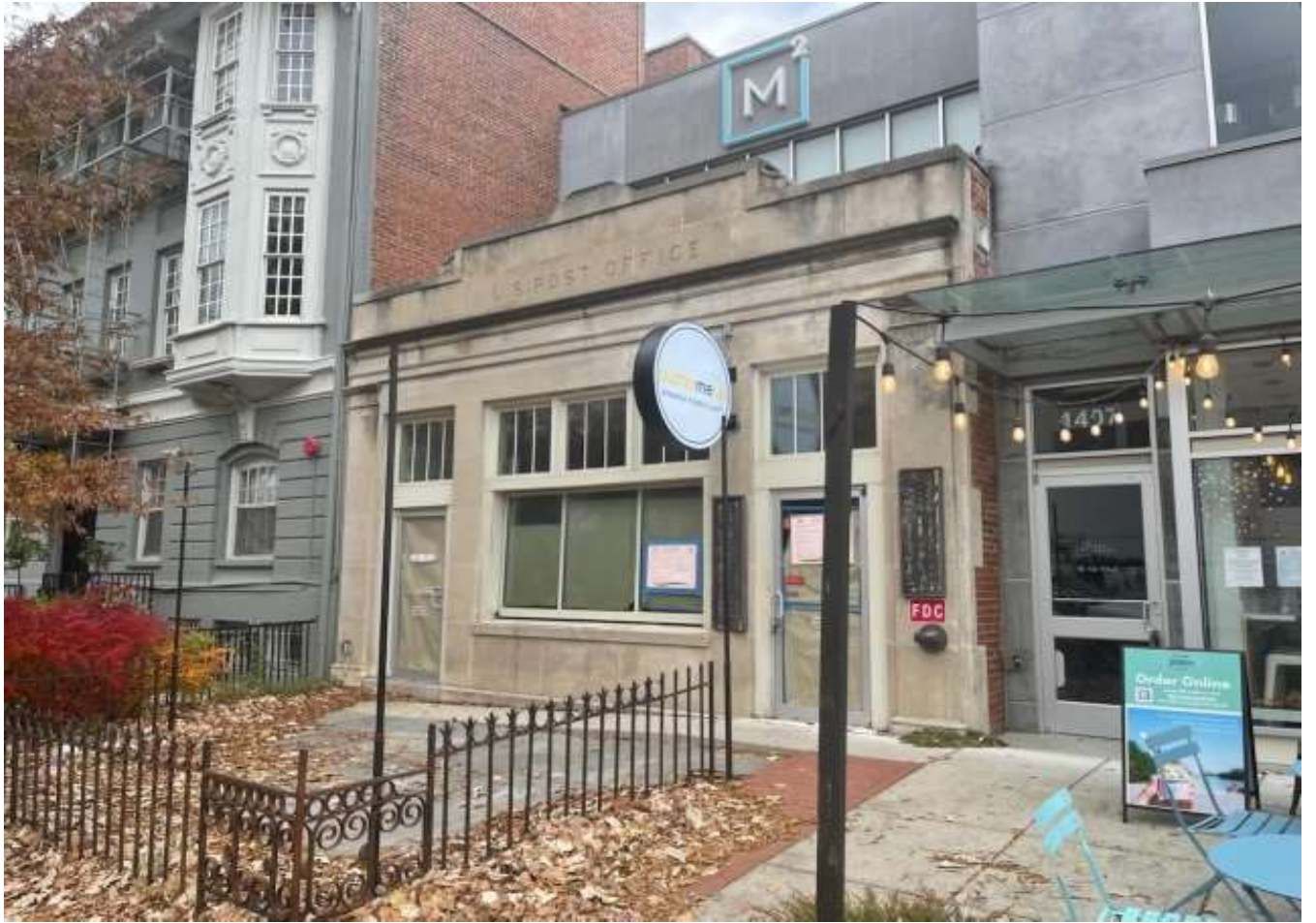
Blade sign installed at 1409 T Street NW
