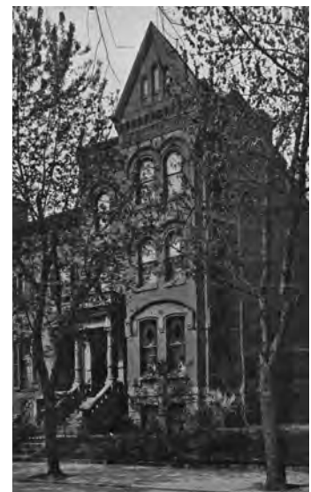
Figure 3-2. Women's Christian Temperance Union headquarters at 522 6th Street NW, demolished (StreetsofWashington).
