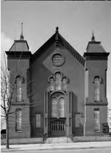
Figure 3-5. Nineteenth Street Baptist Church at 19th and I Streets NW in 1975, demolished (Library of Congress).
