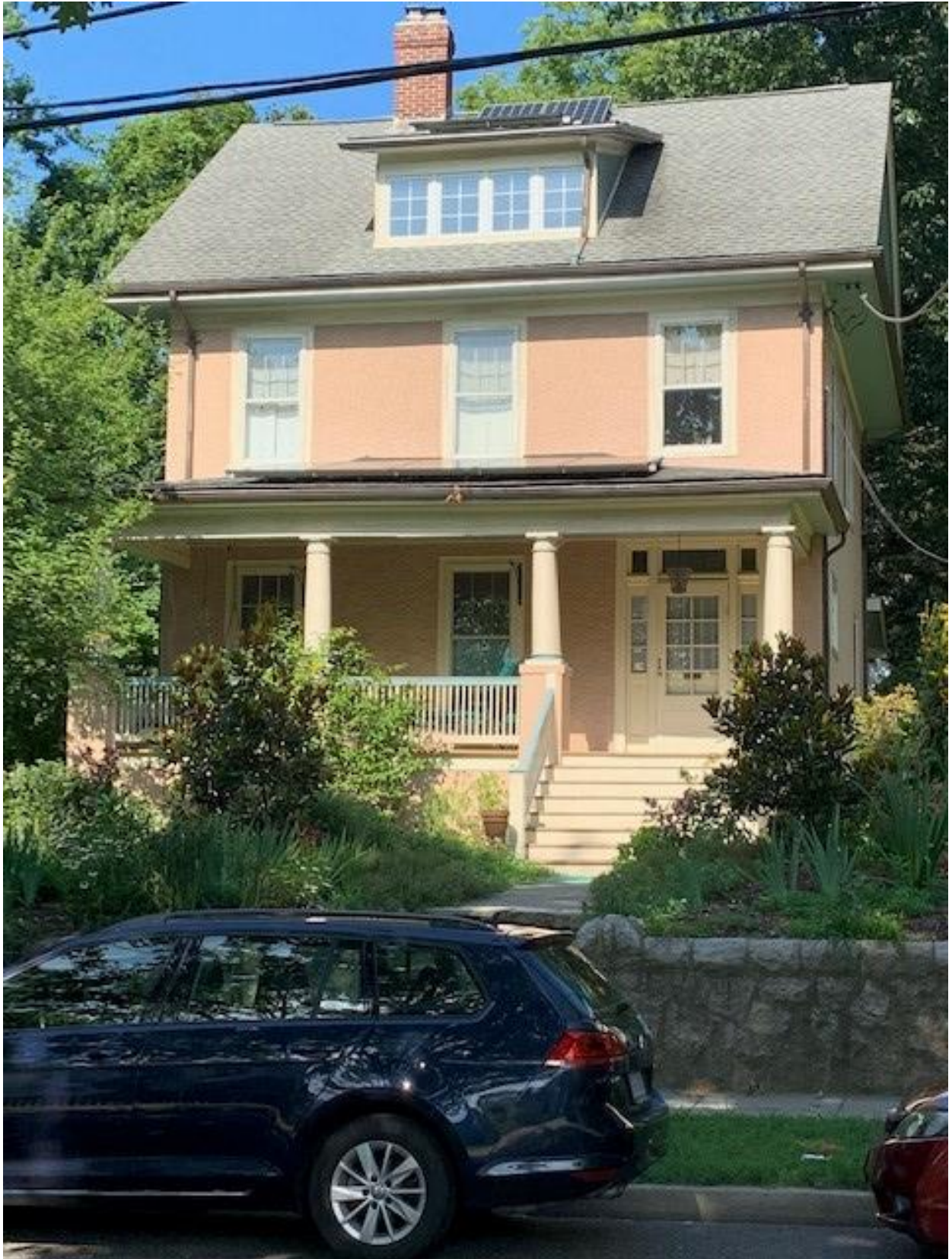
6824 5 th Street NW with panels on porch and dormer roof approved by HPRB in 2018
