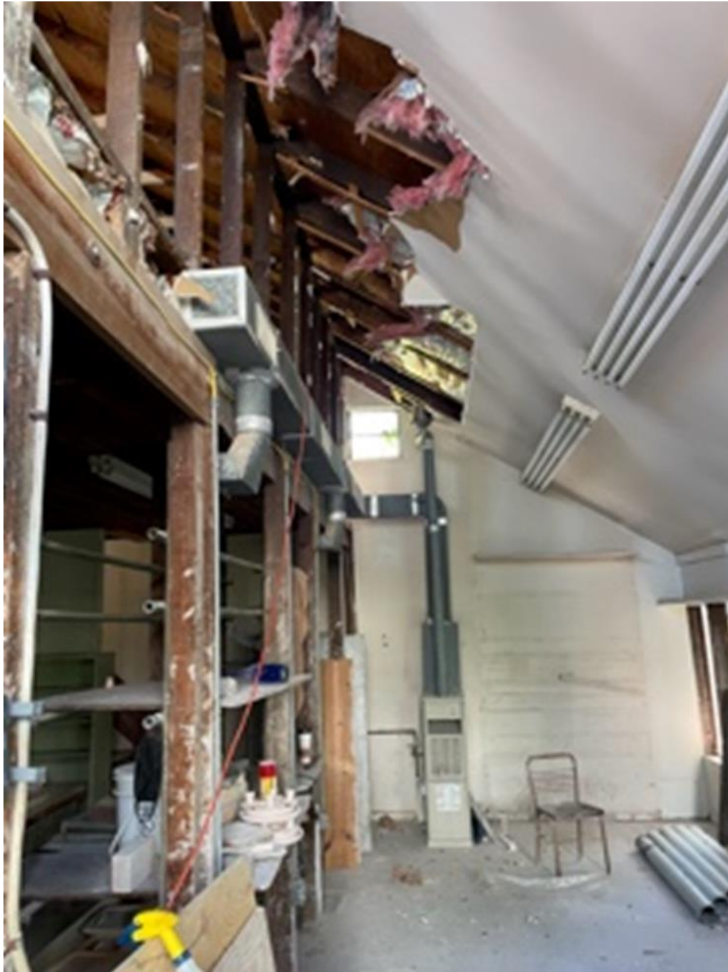
Interior of outbuilding at 515 Cedar showing older wall framing and newer roof framing. The older framing elements are of different sizes, possibly indicating that they were reclaimed and reused.
