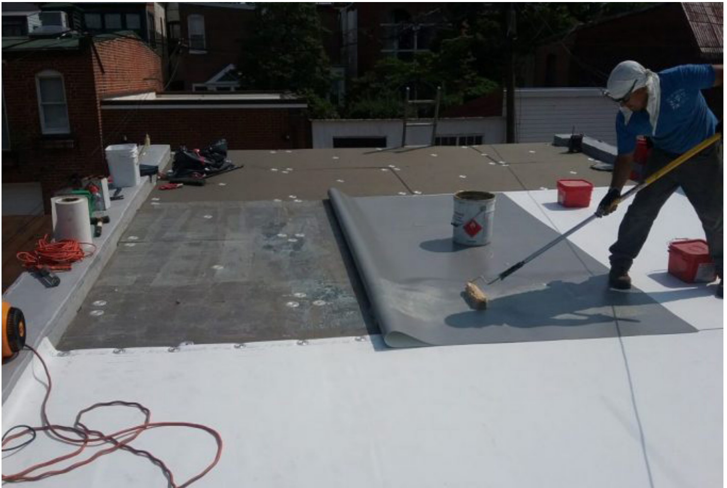
ROOF MEMBRANE REPLACEMENT
