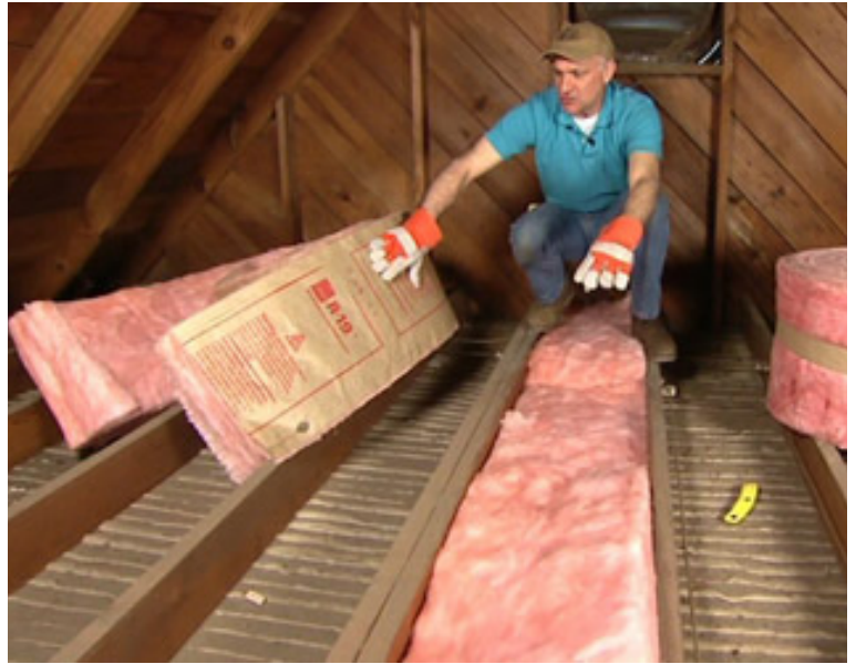
BATT INSULATION BETWEEN THE CEILING JOISTS
