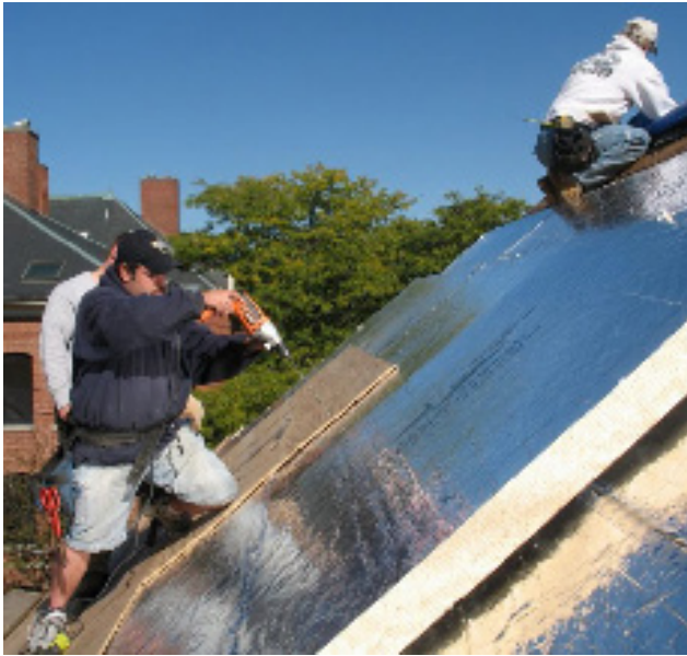
RIGID INSULATION ON A SLOPED ROOF
