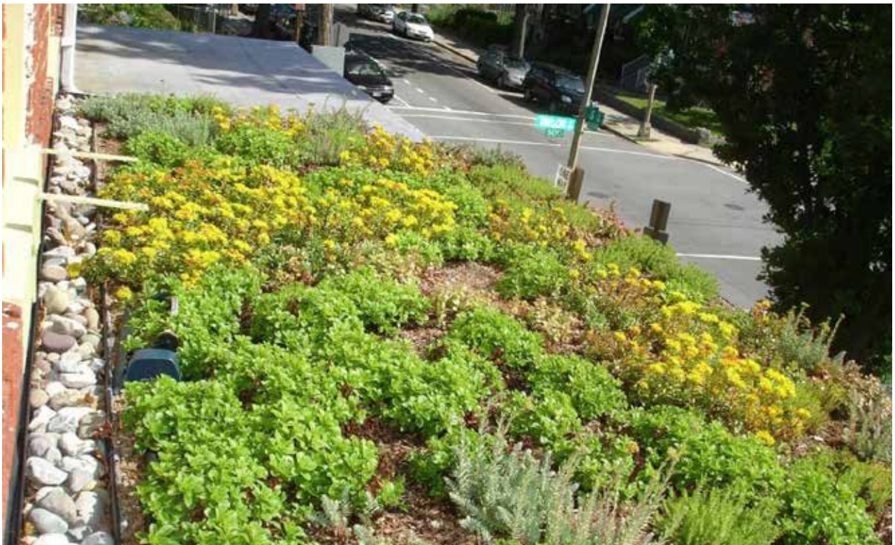
GREEN ROOF ON PORCH ROOF OF ROWHOUSE
