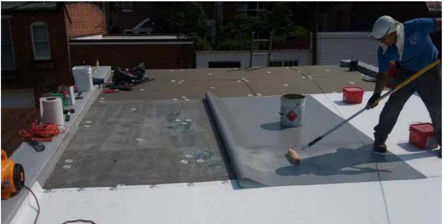
ROOF MEMBRANE REPLACEMENT
