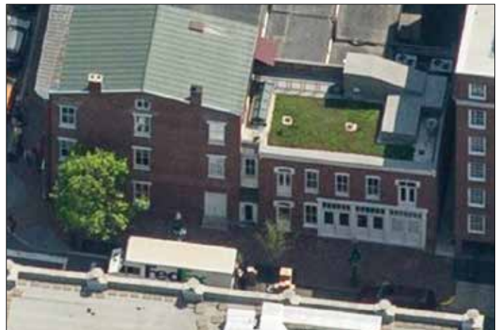
VISIBILITY OF THE GREEN ROOF ON THIS LOW-RISE BUILDING IS MINIMIZED BY A SETBACK FROM ROOF EDGES.
