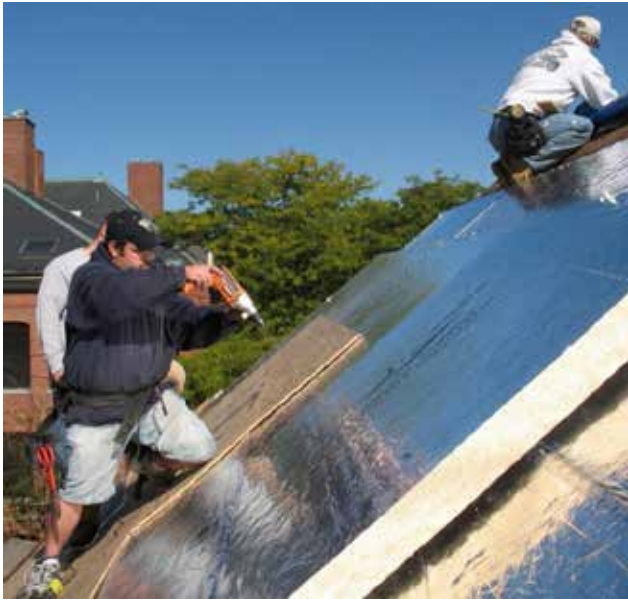
RIGID INSULATION ON A SLOPED ROOF
