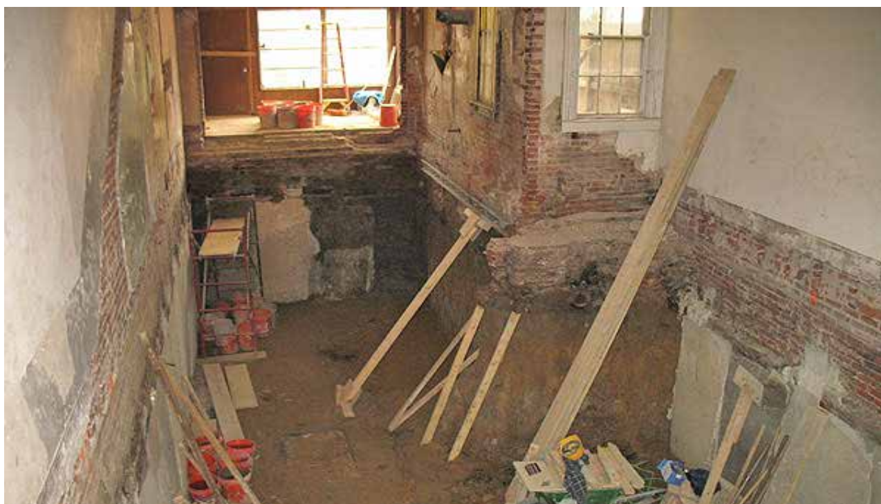
EXCAVATION, SHEETING AND SHORING
