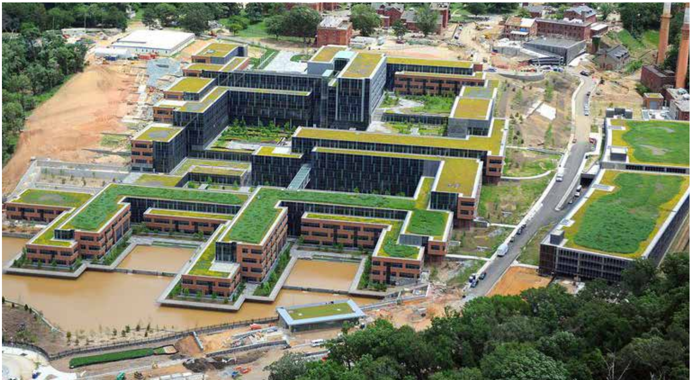
GREEN ROOFS ON US COAST GUARD HEADQUARTERS
