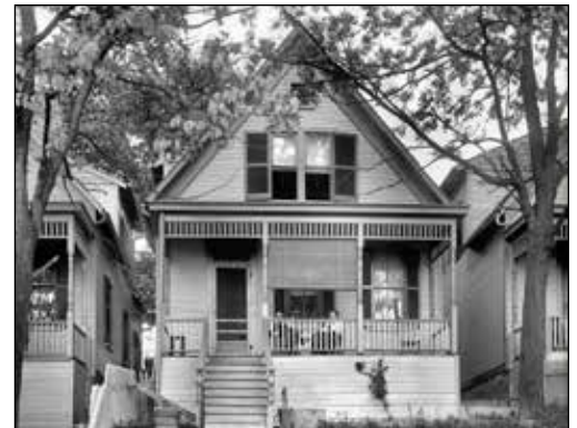
PORCHES PROVIDE SHELTERED OUTDOOR LIVING SPACE, MAXIMIZE CROSS VENTILATION, AND SHADE EXTERIOR WALLS AND WINDOWS. Library of Congress
