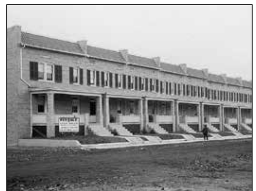
THESE ROWHOUSES HAVE PORCHES, SHUTTERS, AND MASONRY WALLS, ALL OF WHICH IMPROVE PERFORMANCE AND ENERGY-EFFICIENCY. Library of Congress
