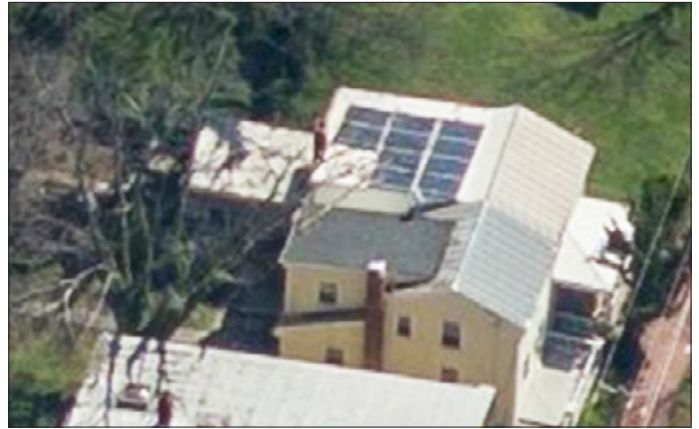
SOLAR PANELS ON THE REAR ROOF SLOPE OF THIS SEMI-DETACHED HOUSE ARE INSTALLED FLUSH TO THE ROOF AND SETBACK FROM EDGES MINIMIZING VISIBILITY FROM THE STREET.
