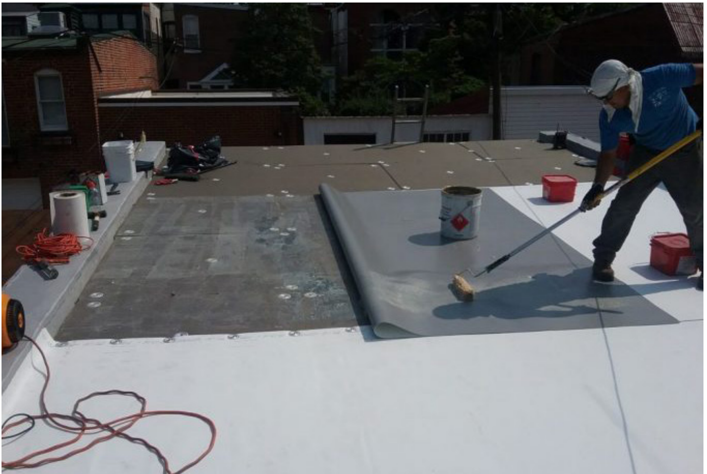
ROOF MEMBRANE REPLACEMENT
