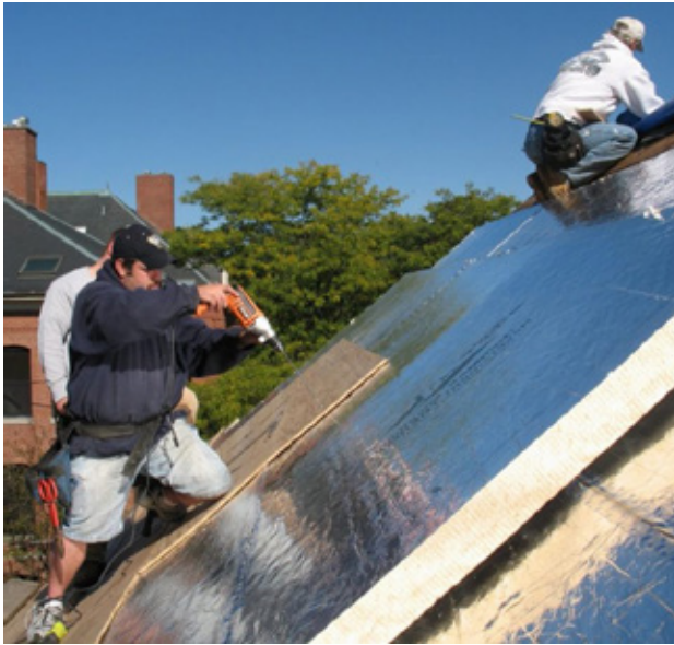
RIGID INSULATION ON A SLOPED ROOF
