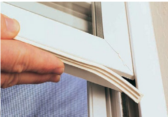
WOOD WINDOW WEATHERSTRIPPING
