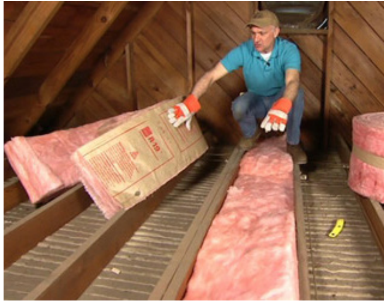
BATT INSULATION BETWEEN THE CEILING JOISTS
