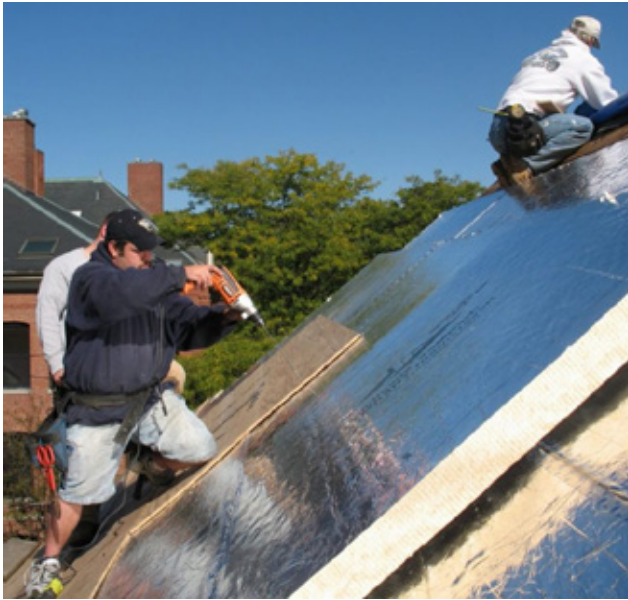
RIGID INSULATION ON A SLOPED ROOF
