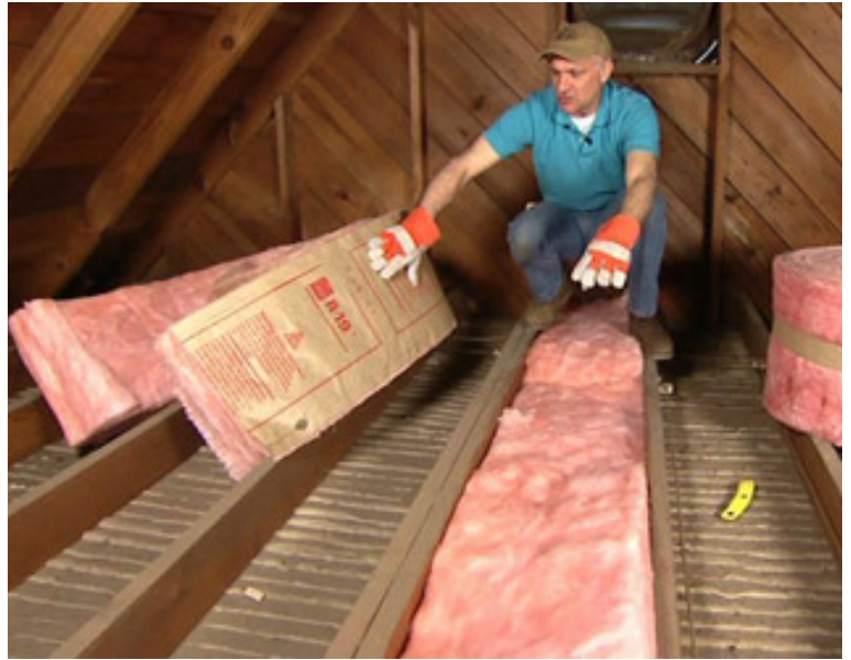
BATT INSULATION BETWEEN THE CEILING JOISTS
