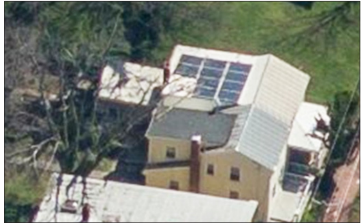
SOLAR PANELS ON THE REAR ROOF SLOPE OF THIS SEMI-DETACHED HOUSE ARE INSTALLED FLUSH TO THE ROOF AND SETBACK FROM EDGES TO MINIMIZE VISIBILITY FROM THE STREET.
