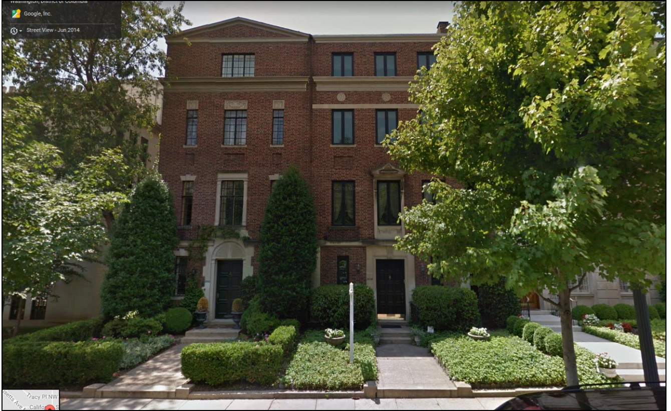
1806 24 th Street (left), prior to unpermitted work
