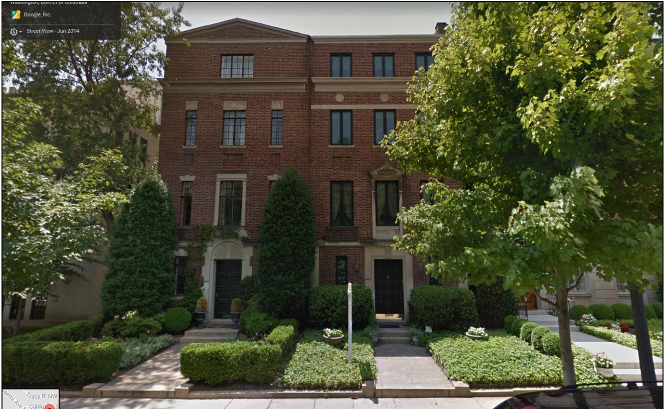
1806 24 th Street (left), prior to unpermitted work
