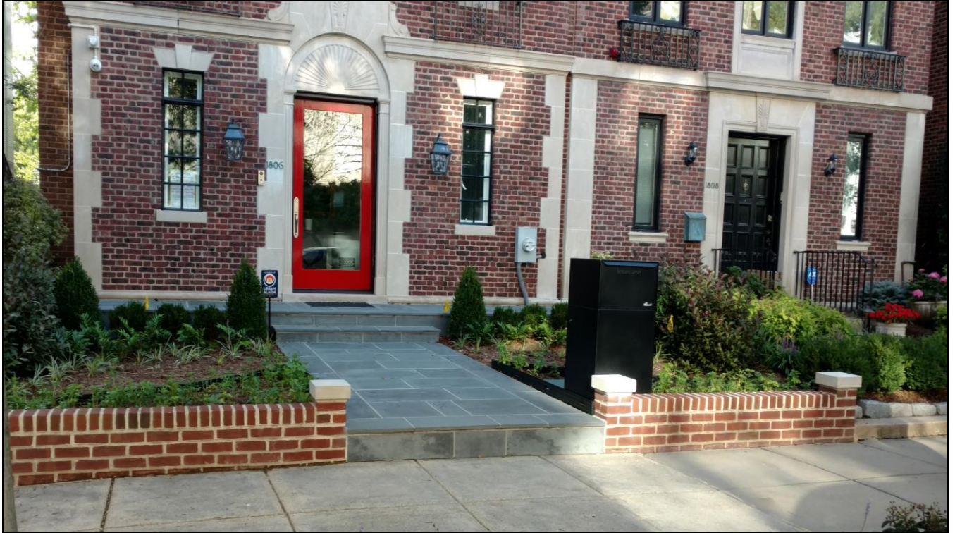
1806 24 th Street (left), after unpermitted work
