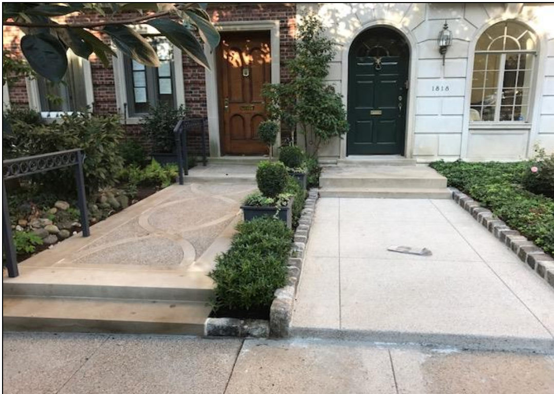
Recently completed replacement walks at 1816 and 1818 24 th Street, constructed after consultation with HPO and obtaining building permits, that replicate the material and coloration of the original walks.
