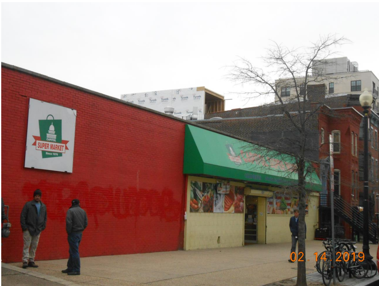
Figure 1. Unpermitted construction, February 14, 2019. Height difference of 8 feet; now removed. Current concept would produce a 2'-8" height difference.
