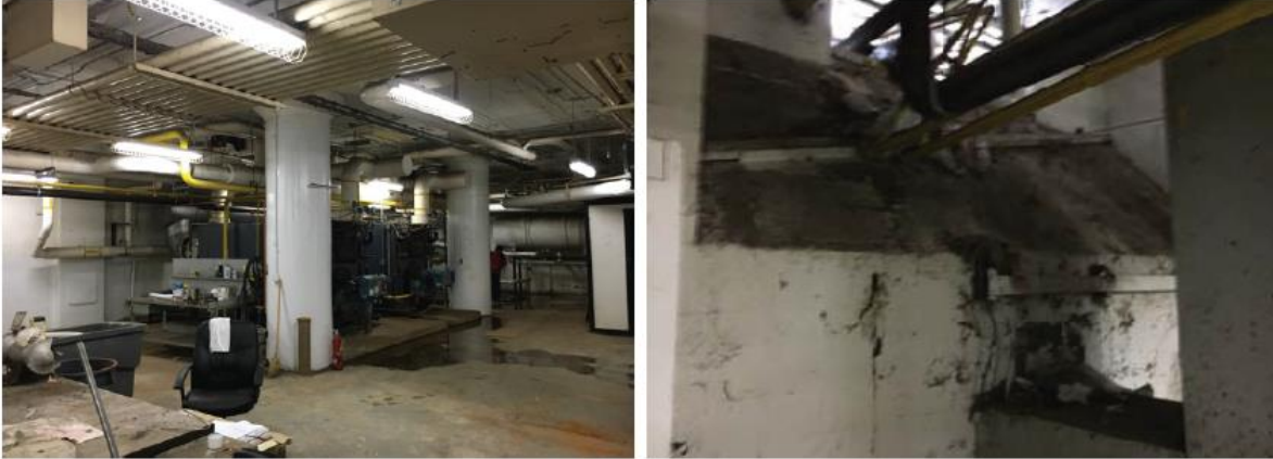
Figure 3.15 Existing Substructure Conditions, National Geographic Society Warehouse
