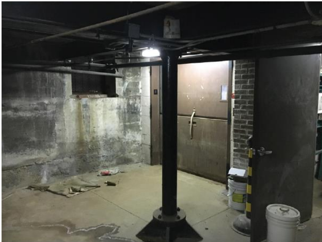
Figure 3.29 Steel Column at Basement of Schlitz Building
