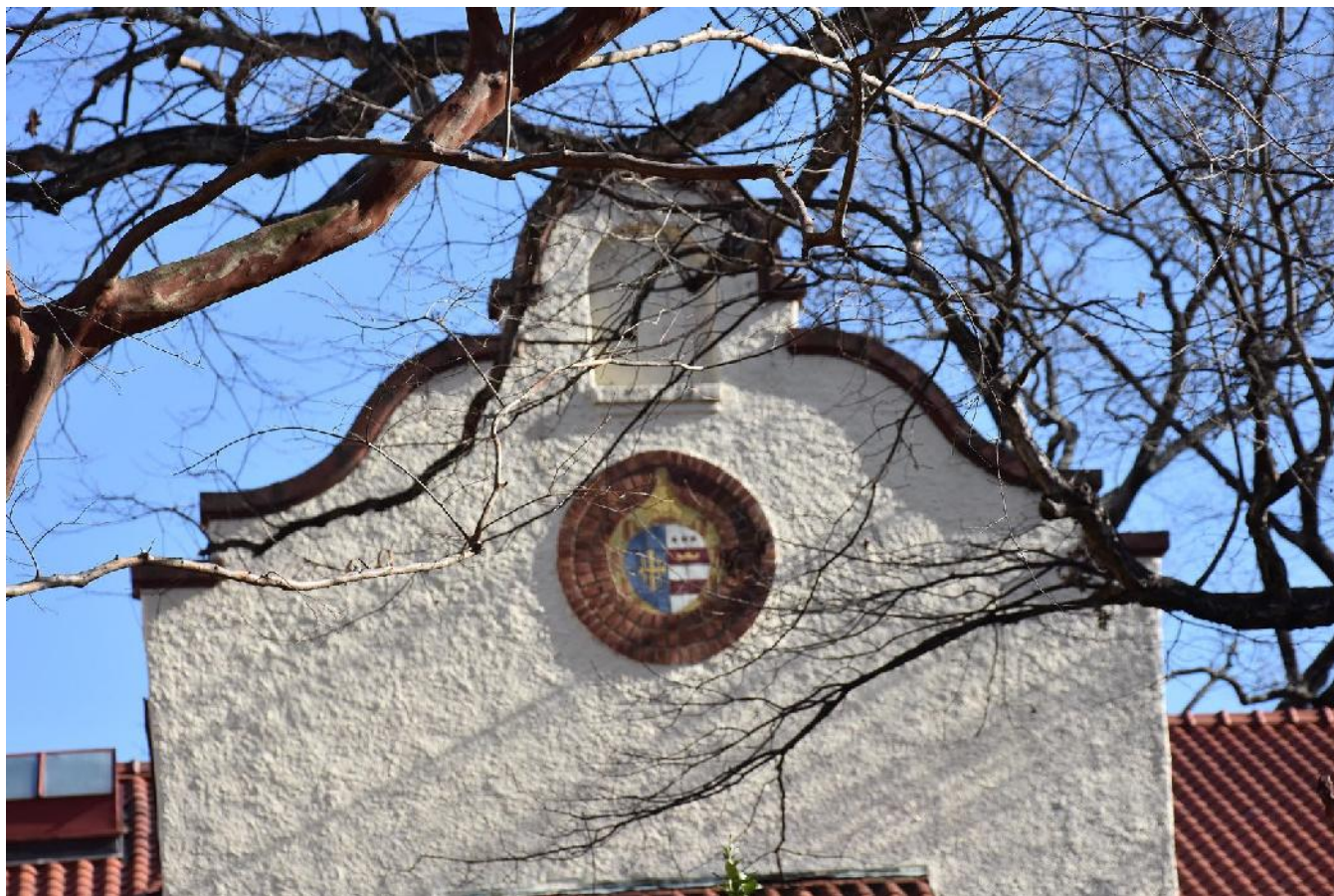
Photo 14: Rosemount Center, Main Block Rear Façade, Parapet detail (D.P. Sefton).
