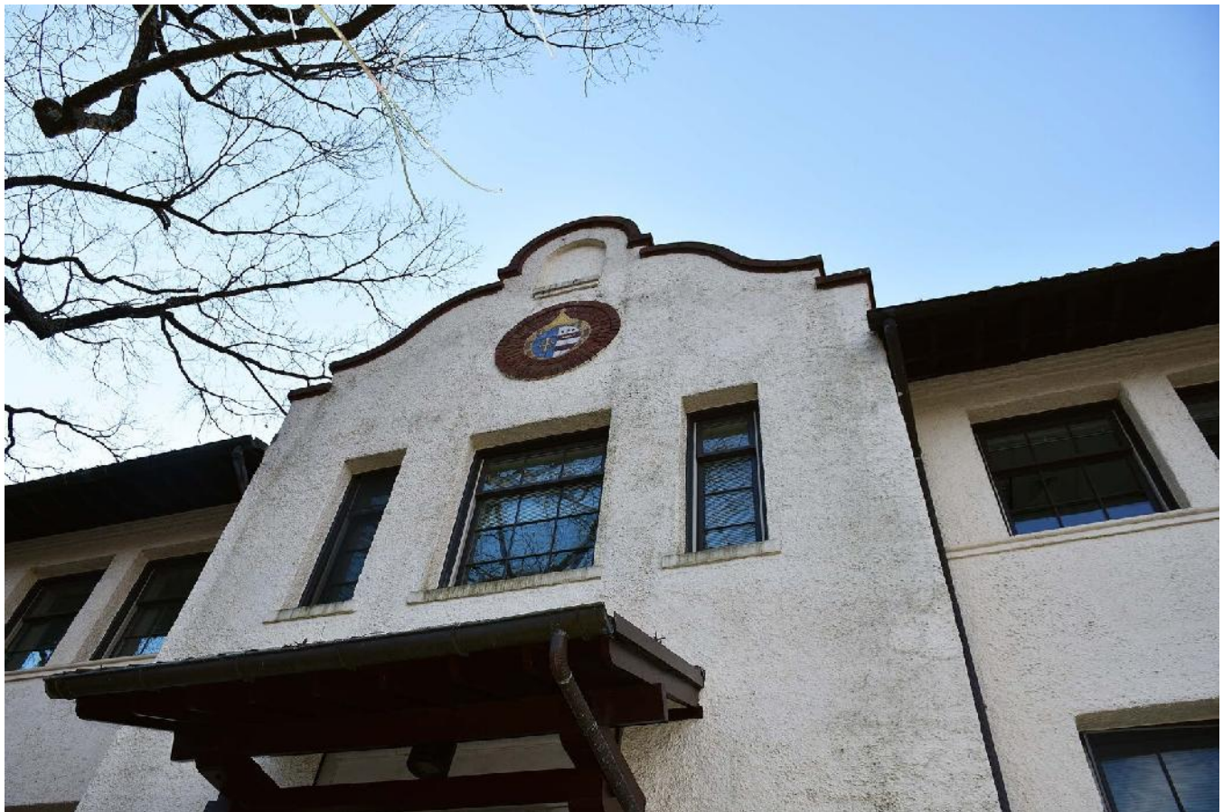
Photo 6: Rosemount Center, Front Façade Parapet detail (D.P. Sefton).
