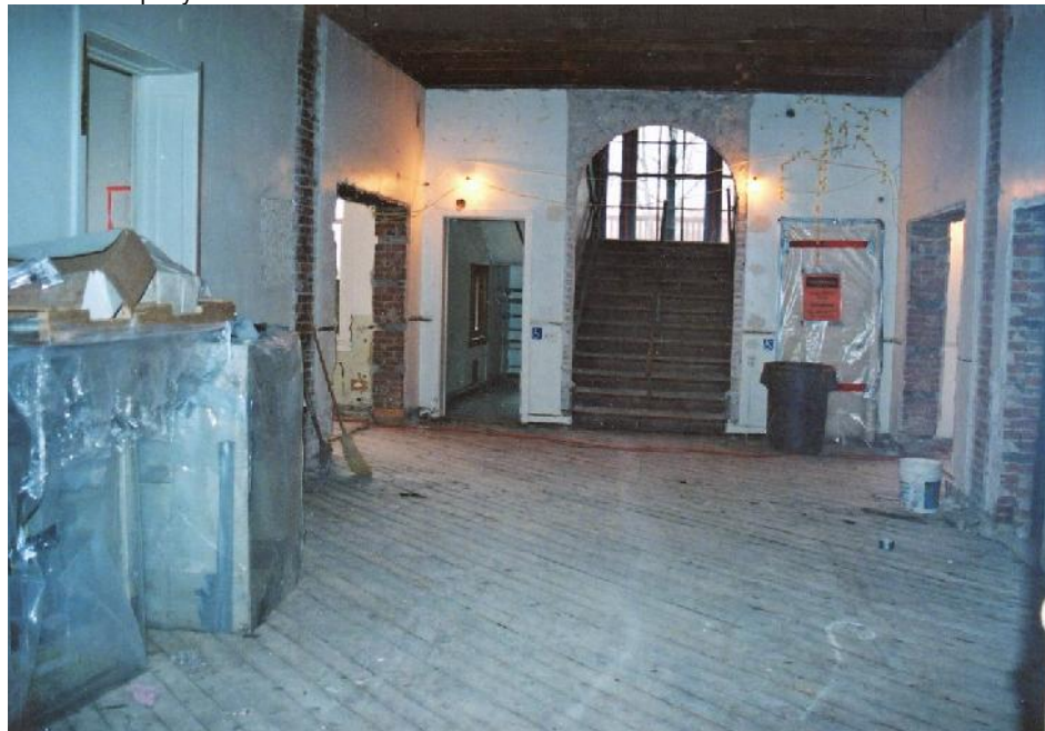
Figure 6: The entrance foyer during renovation in 2005 (Rosemount Center archives).
