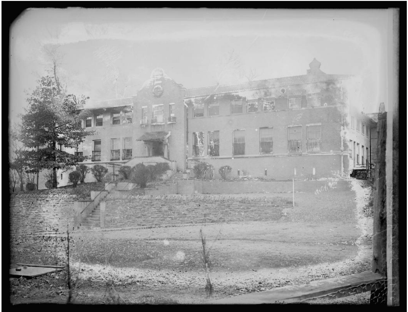
Photo 1: Undated, damaged early photo of the House of Mercy, Front (East) Façade from Rosemount Avenue, showing the original staircase to the main entrance. (Library of Congress).
