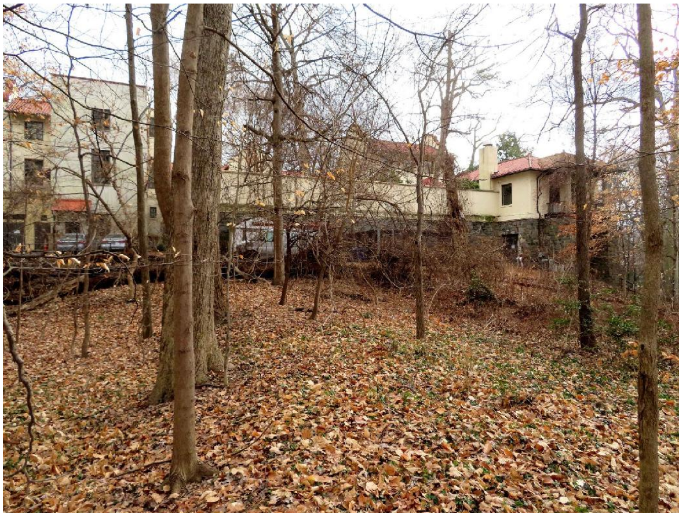
Photo 8: Rosemount Center, West Side from Rock Creek Park, Showing Retaining Wall and Rear Extension of North Wing (J. DeFerrari).
