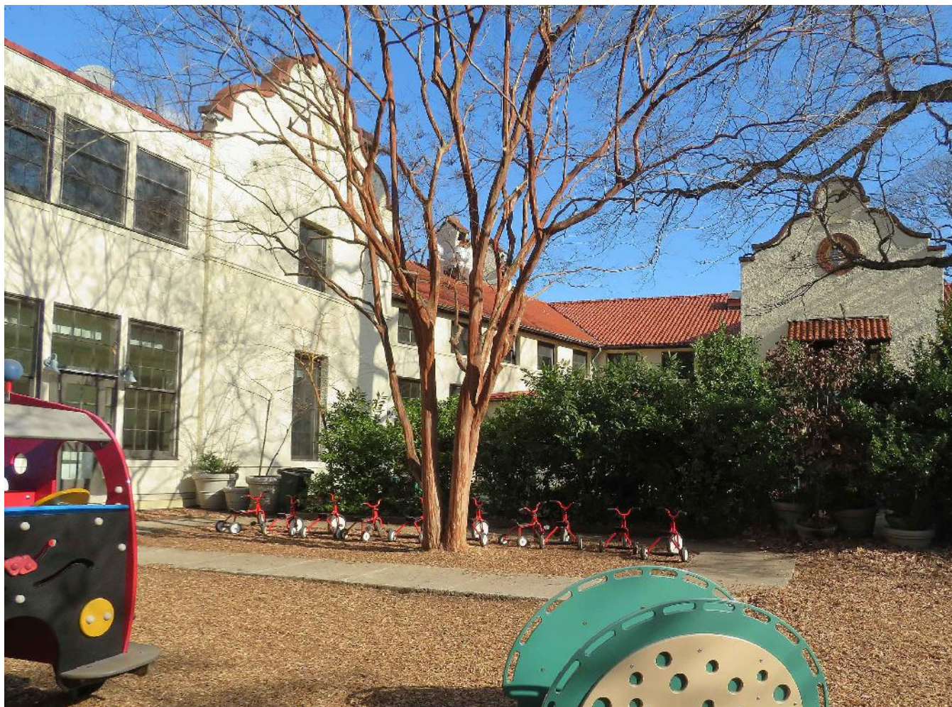
Photo 10: South Side of North Wing showing Rear Extension (J. DeFerrari).
