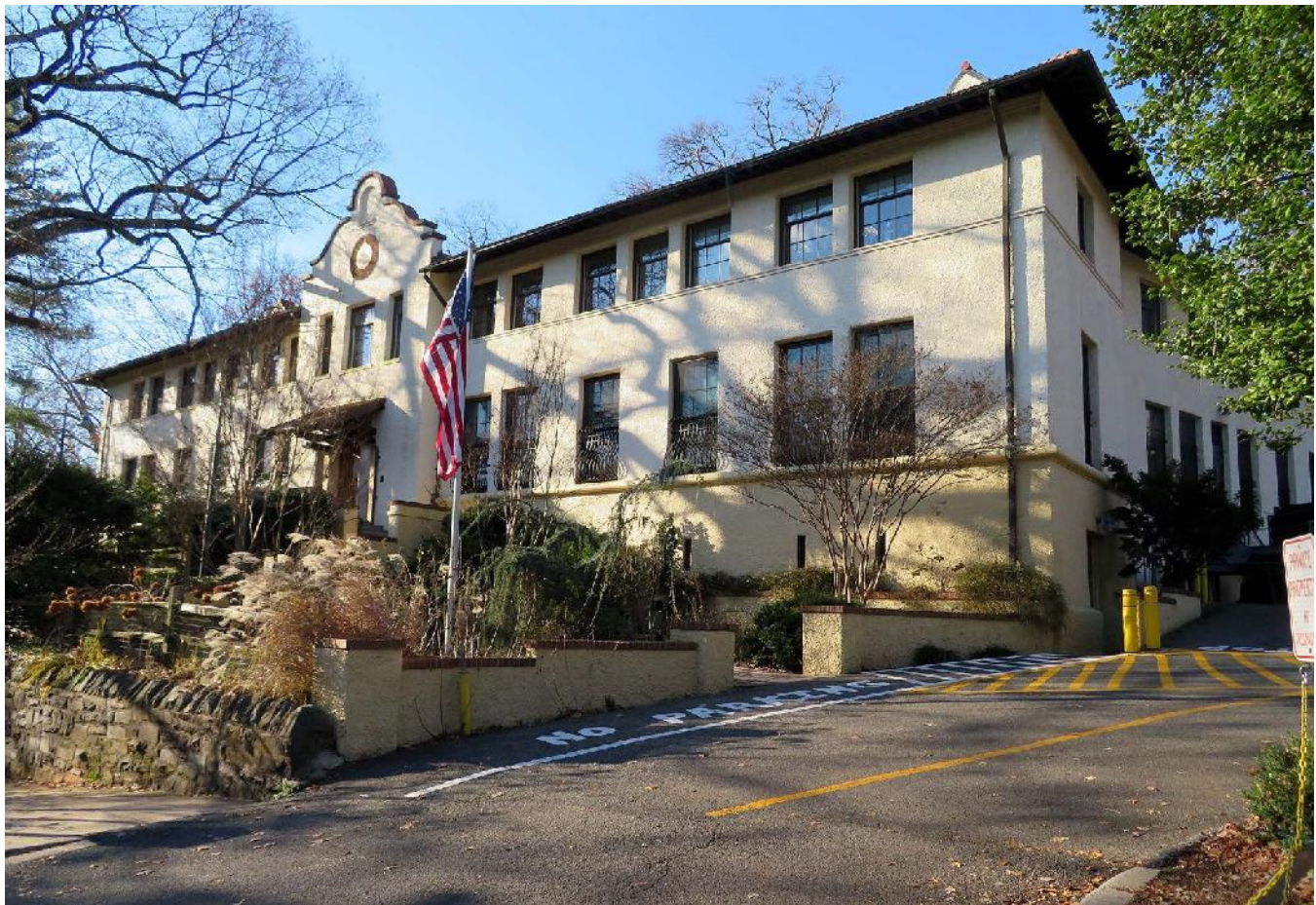
Photo 5: Rosemount Center, Front (East) Façade from Rosemount Avenue NW (J. DeFerrari).
