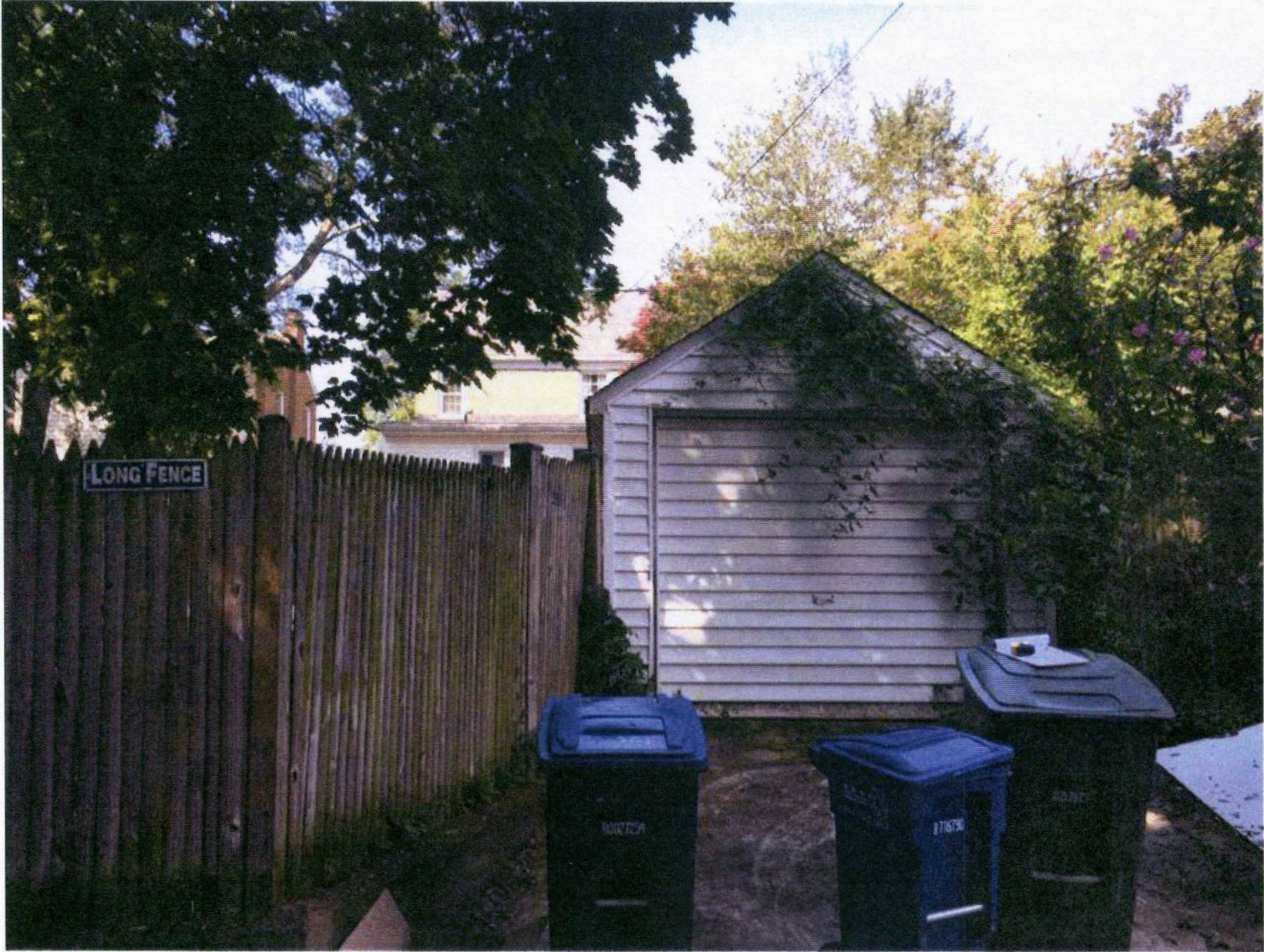
VIEW OF EXISTING GARAGE
