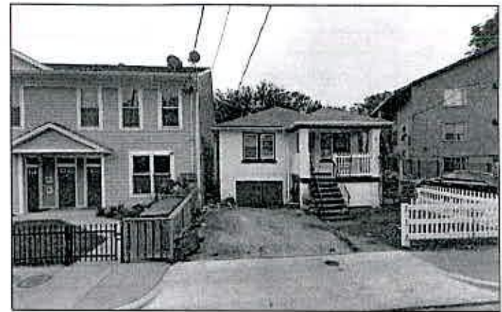
PICTURE BEFORE DEMOLITION STARTED IN MAY 2019.
