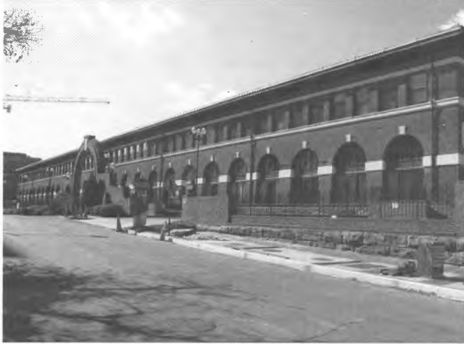
East elevation (looking south) – View 1
