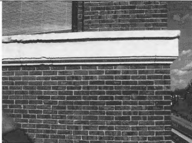
Detail of limestone banding beneath second-story windows
