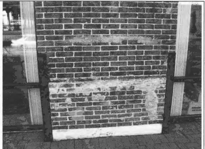
Detail of metal stripping on ground-floor arch openings
