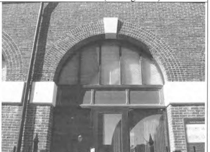
Detail of arch opening, showing keystone and impost blocks
