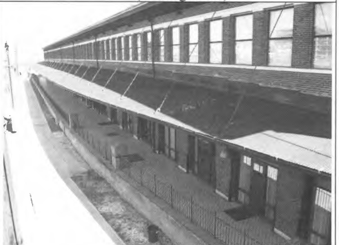
West elevation (looking north)
