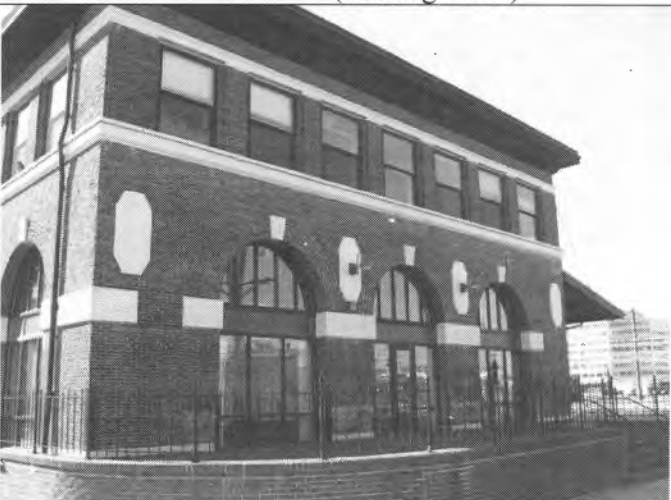
North elevation (looking south)
