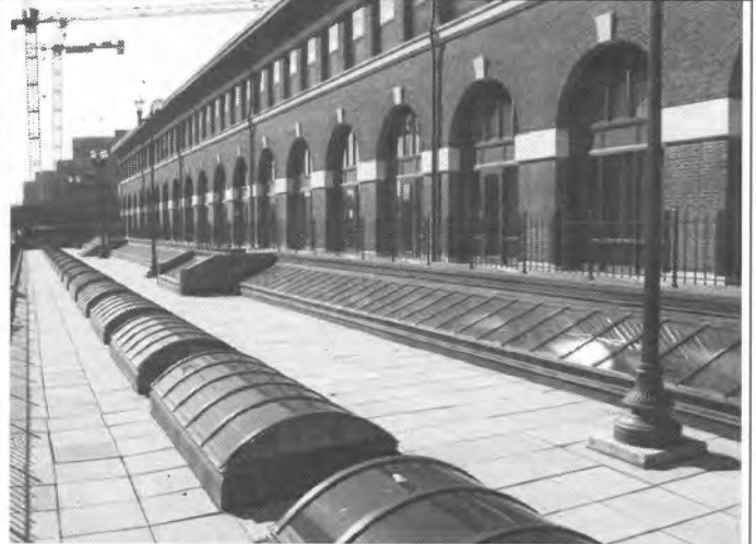
East elevation (looking south) – View 2
