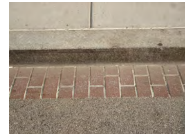
Granite curb with brick gutter
