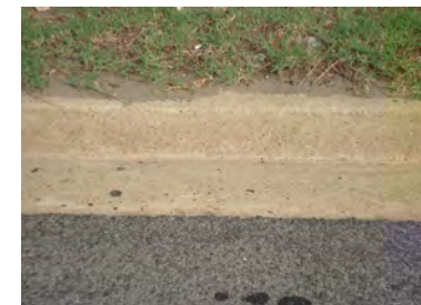
Concrete curb with concrete gutter
