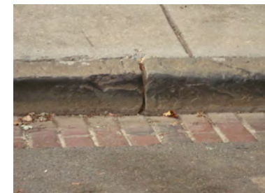
Bluestone curb with brick gutter
