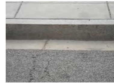
Granite curb with concrete gutter
