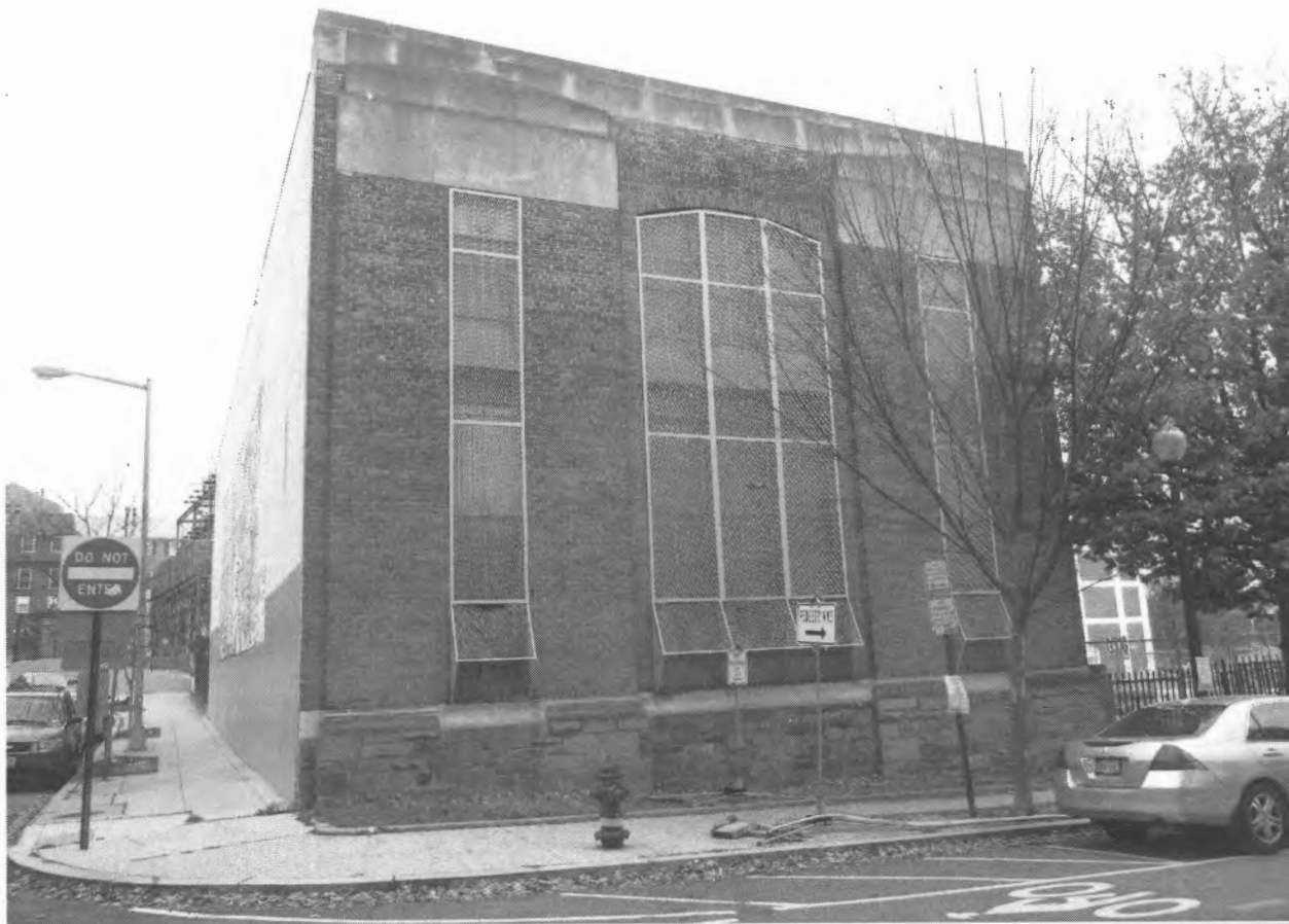
Pepco Substation No. 25
