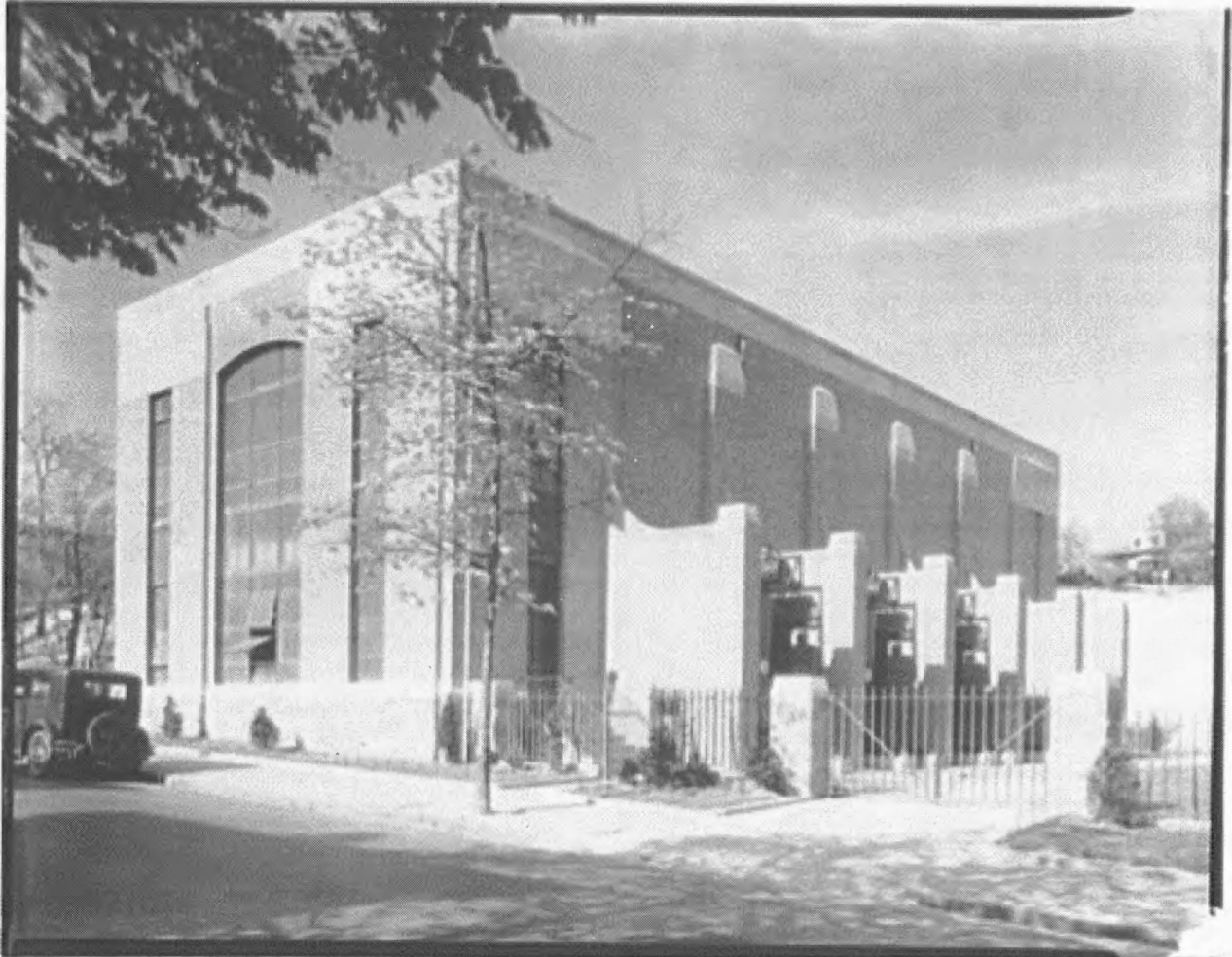
Potomac Electric Power Company Substation No. 25 from the southwest on Champlain Street, NW, ca. 1931. (Photo from Library of Congress)
