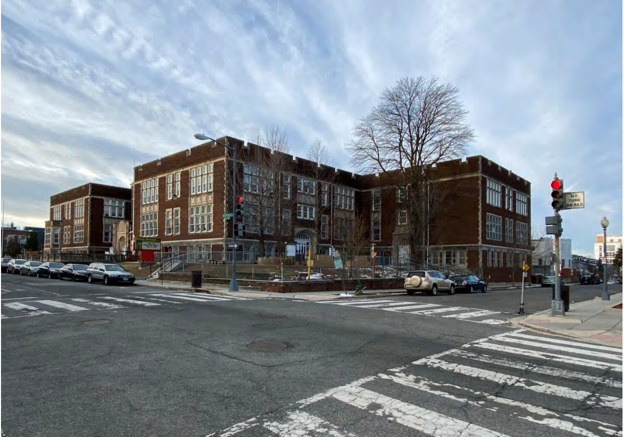
Photo 22 of 23: DC Park View Historic District 020.jpeg Park View School, facing southwest
