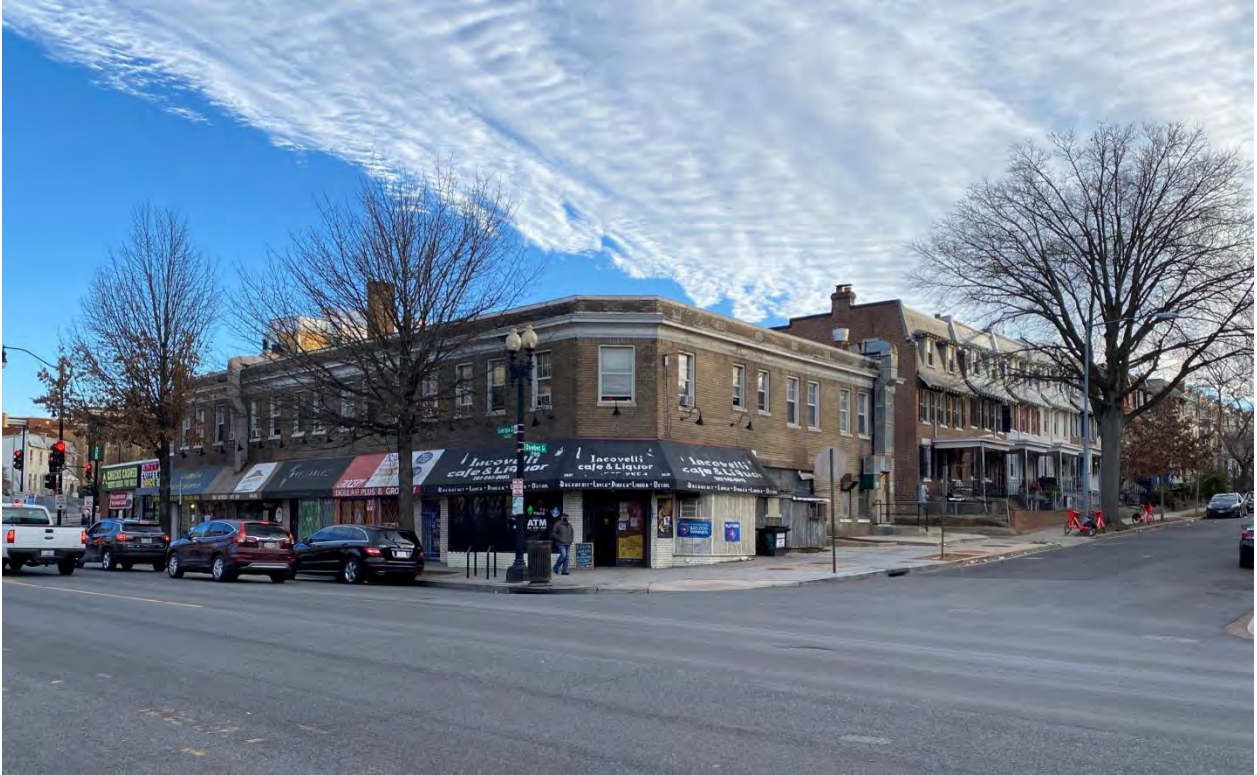
Photo 2 of 23: DC Park View Historic District 002.jpeg 3651 Georgia Avenue, facing northeast
