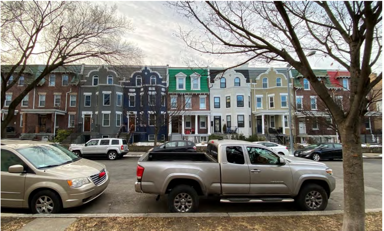
Photo 5 of 23: DC Park View Historic District 006.jpeg 612-626 Rock Creek Church Rd., NW (even), facing south
