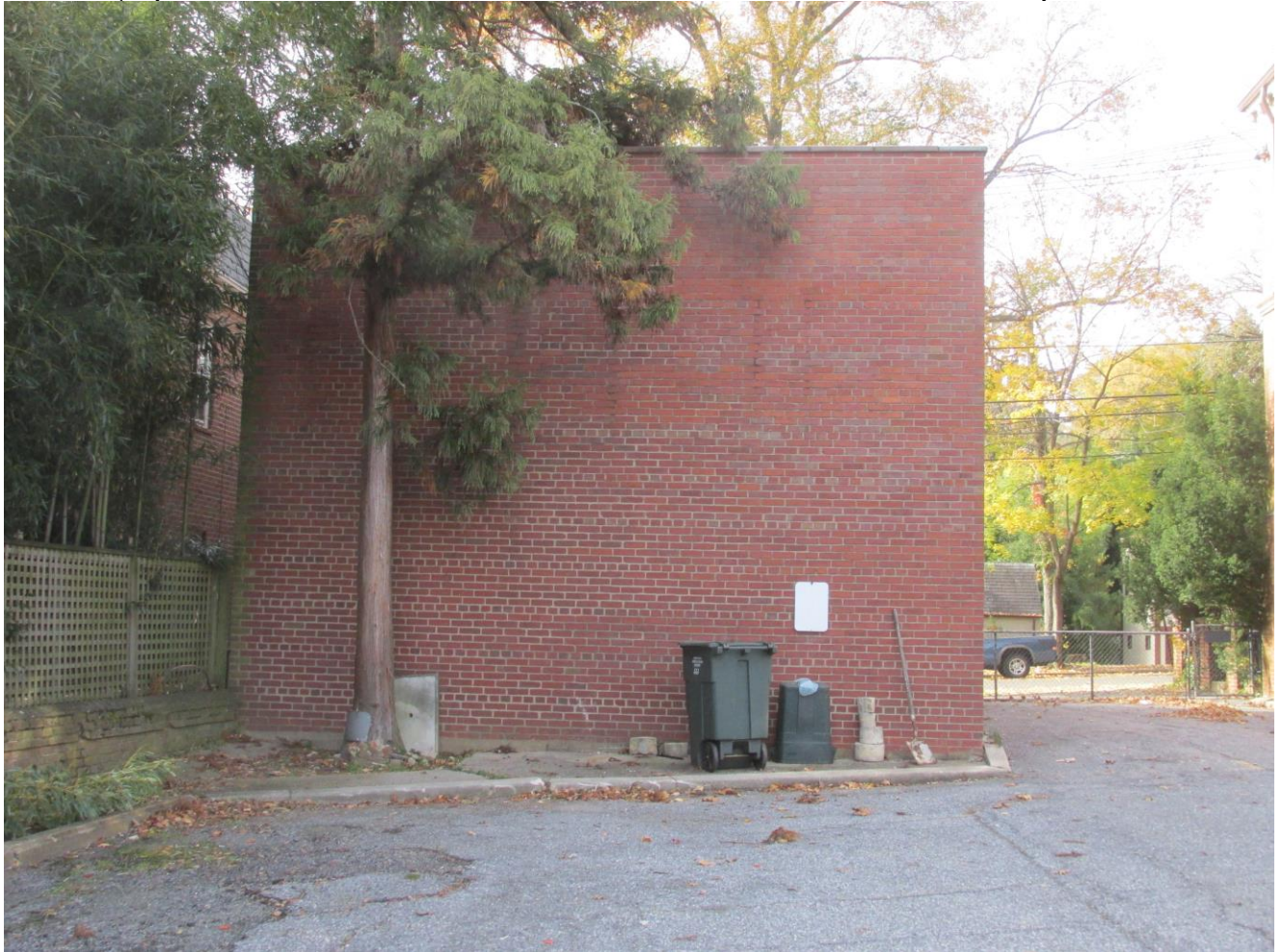
Pepco Substation No. 61
