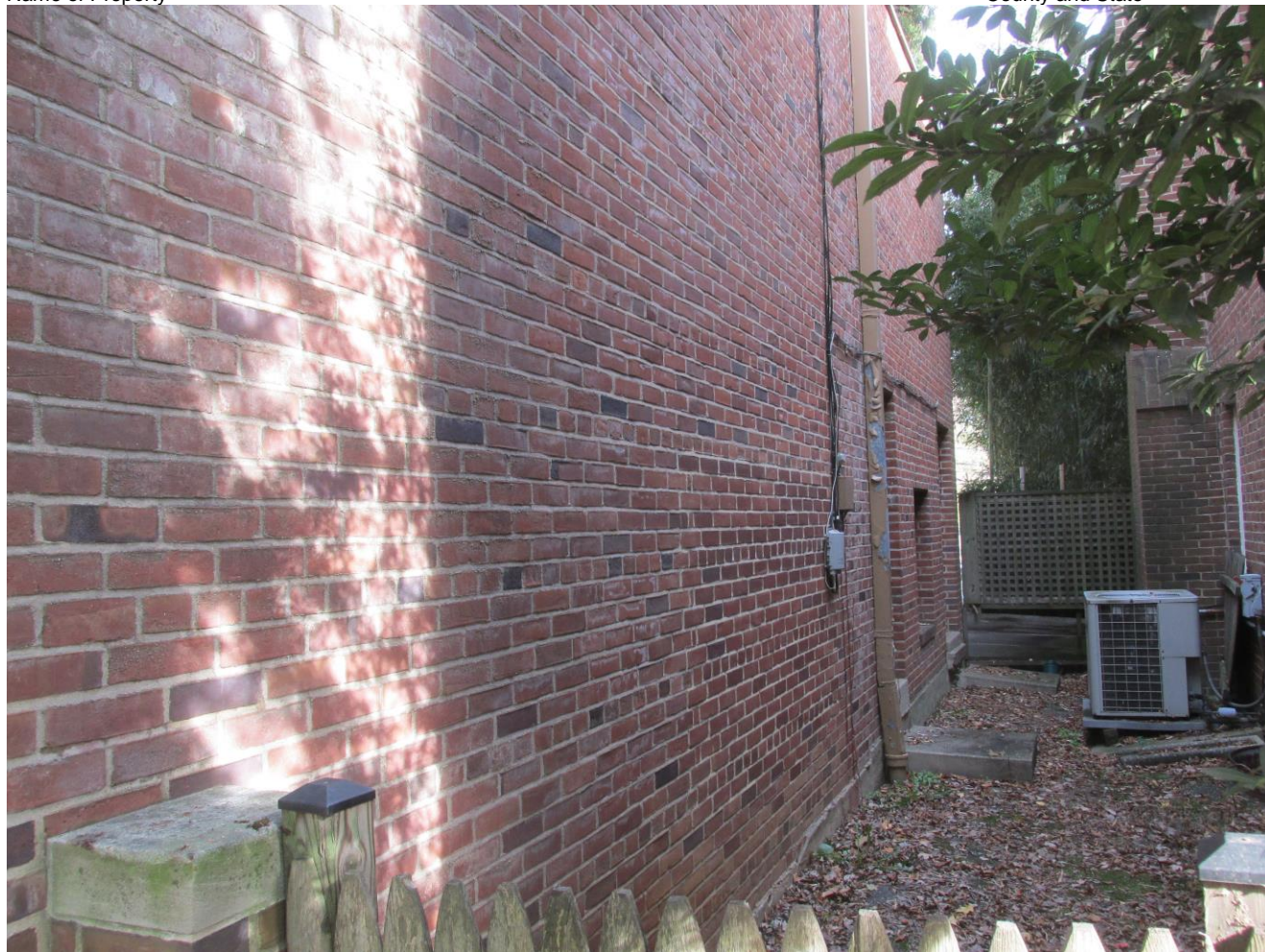
Pepeco Substation No. 61
