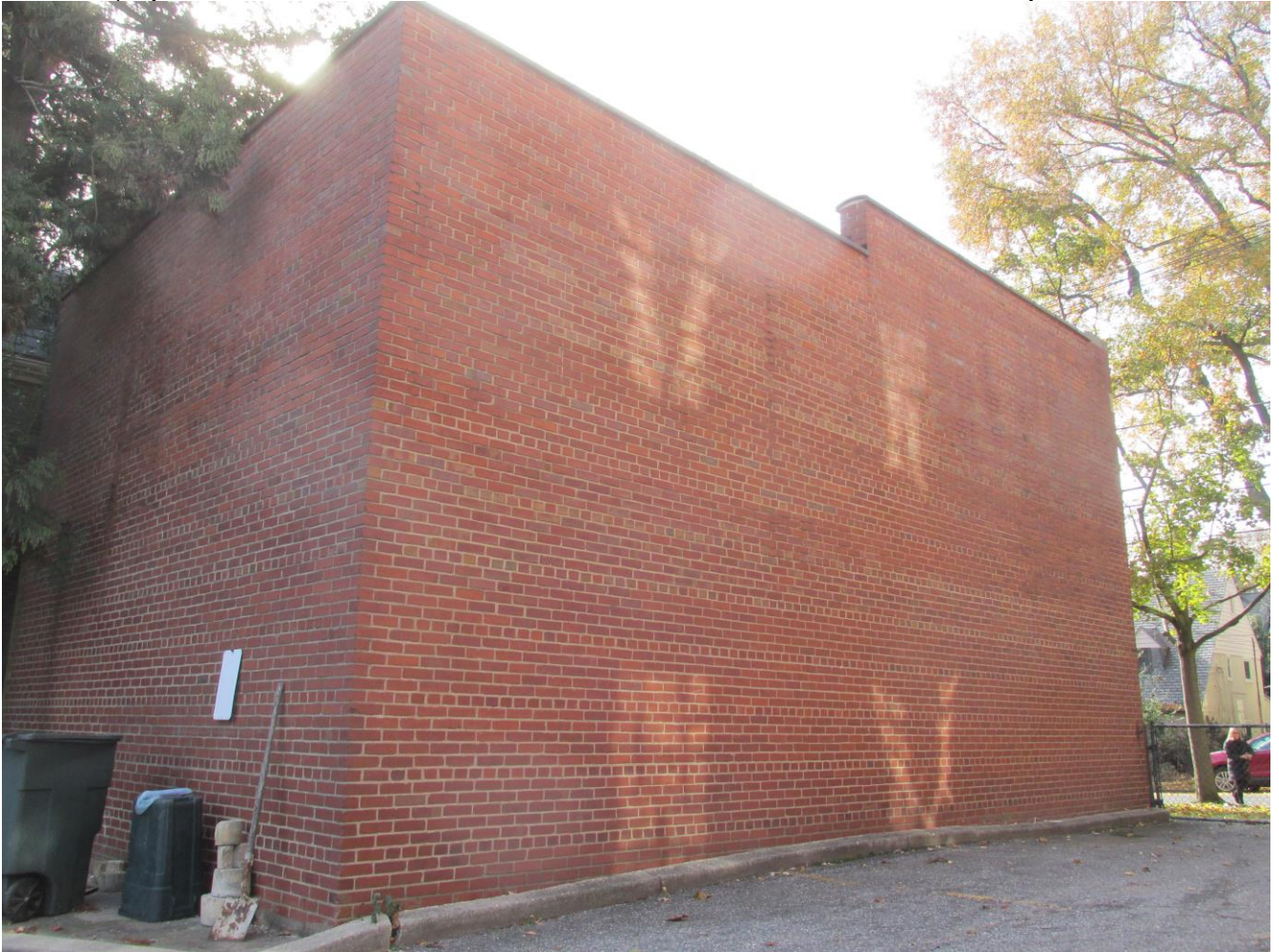
Pepeco Substation No. 61
