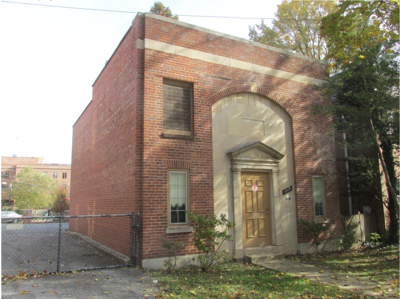
Pepeco Substation No. 61
