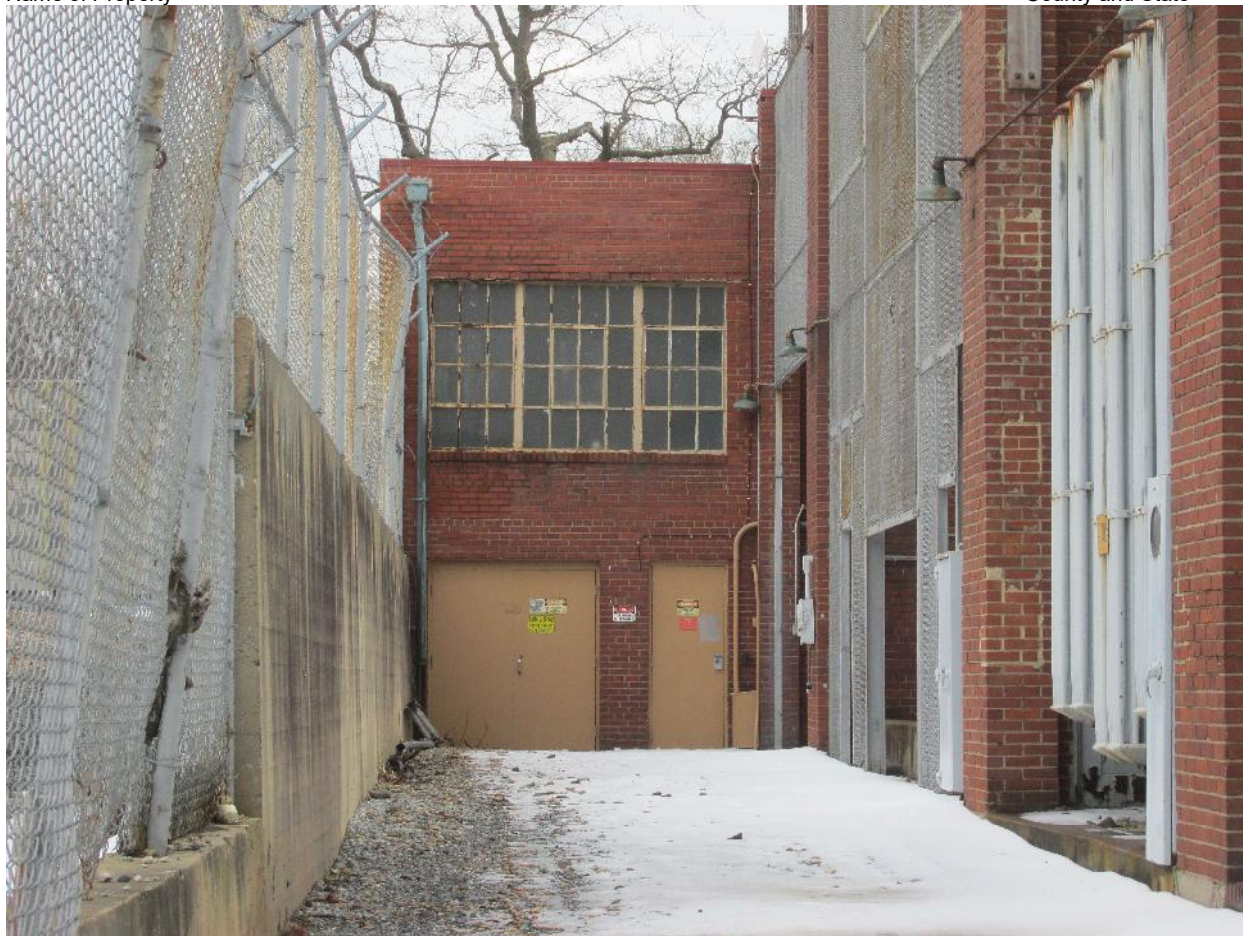
Pepco Harrison Street Substation
