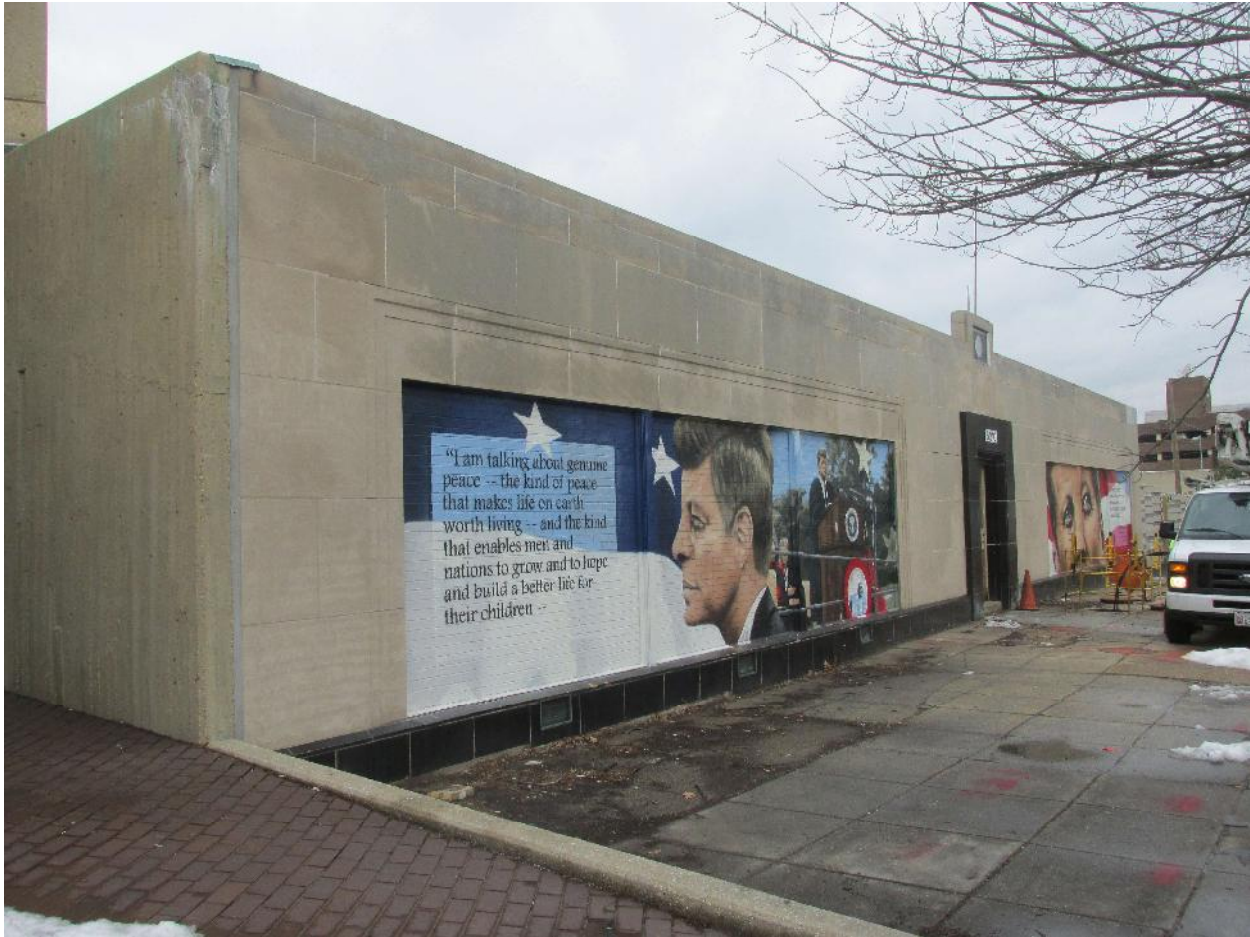
Pepco Harrison Street Substation Washington, DC March 18, 2017 Kent Boese General View looking north from Wisconsin Avenue, NW 2/8
