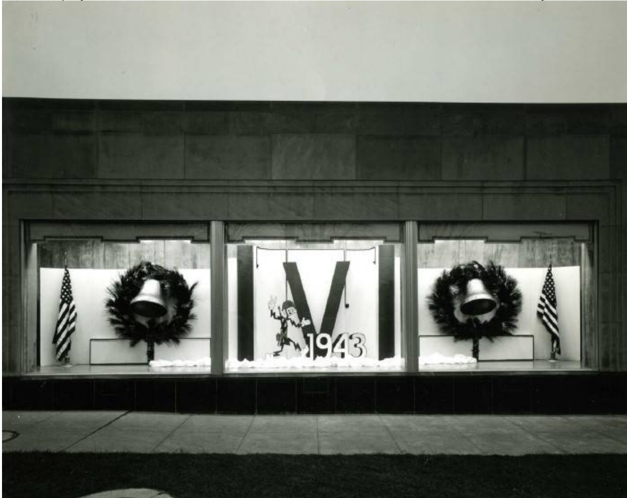
Potomac Electric Power Company Harrison Substation showing window display from December 1943. (Photo from PEPCO)
