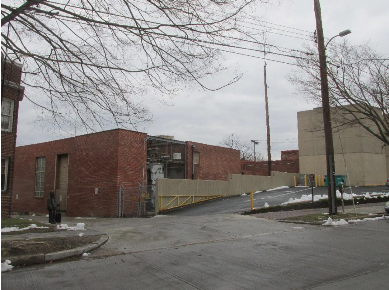
Pepco Harrison Street Substation
