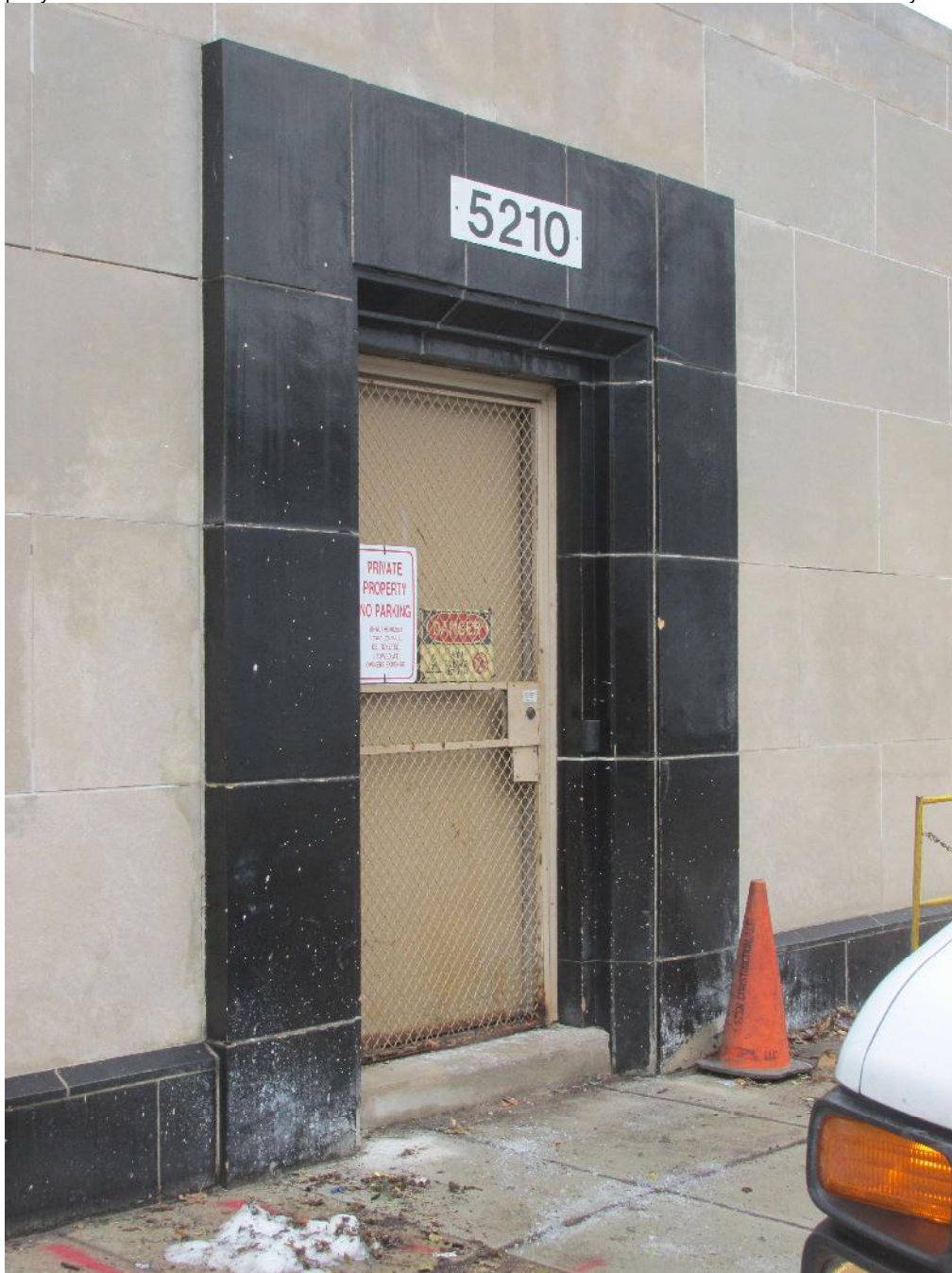
Pepco Harrison Street Substation
