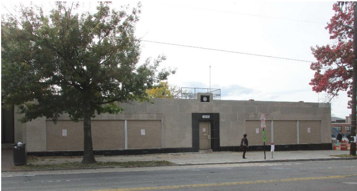
Pepco Harrison Street Substation
