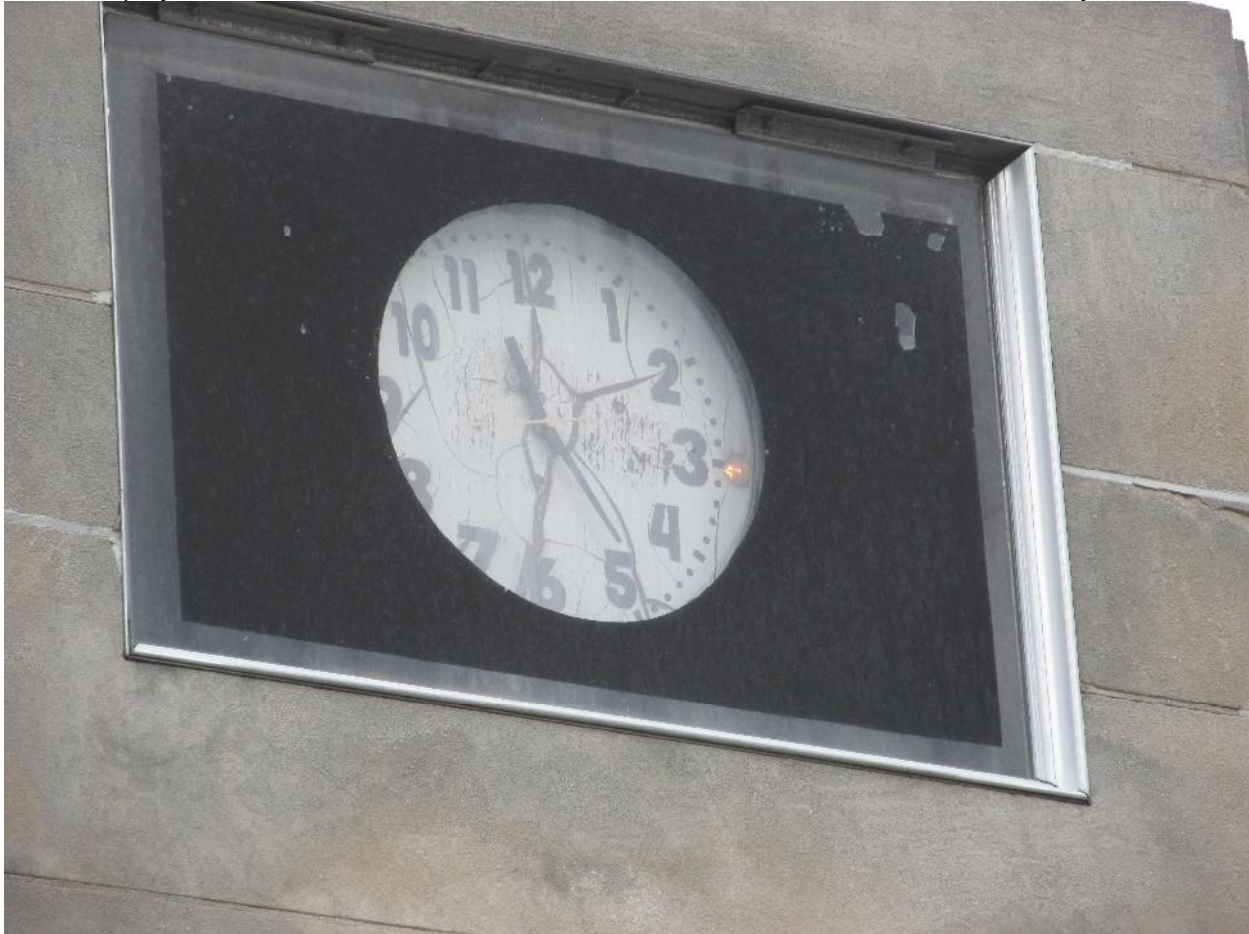
Pepco Harrison Street Substation Washington, DC March 18, 2017 Kent Boese Detail of clock on Wisconsin Avenue Façade 3/8
