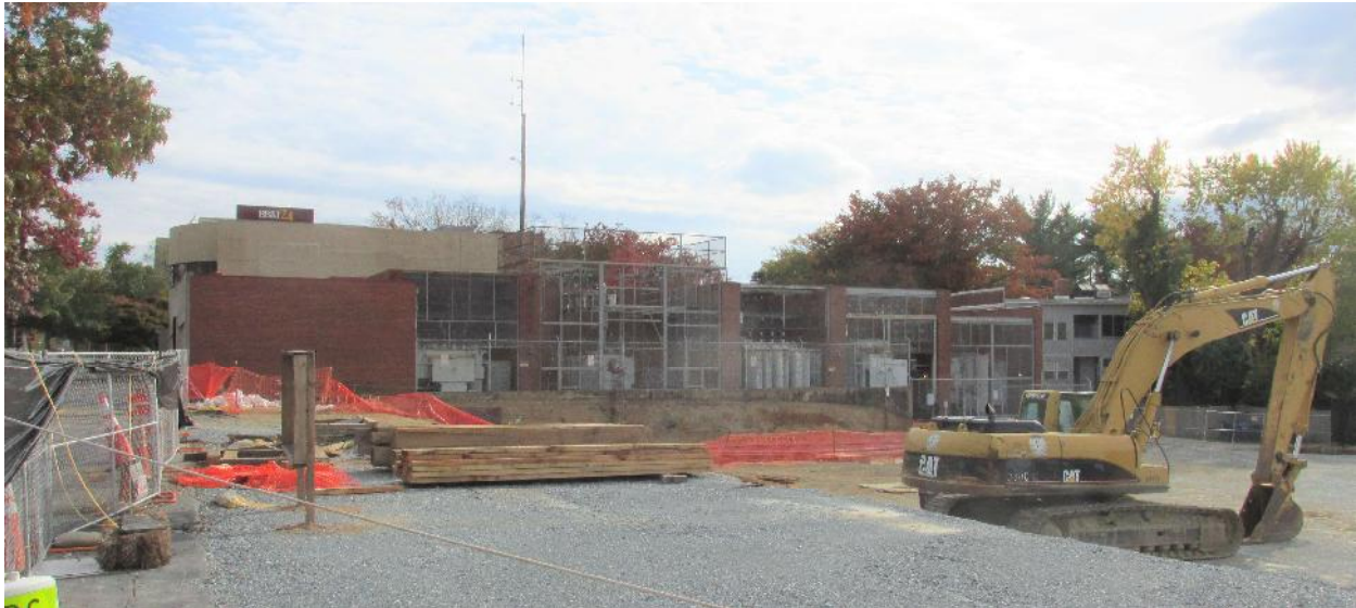
Pepco Harrison Street Substation
