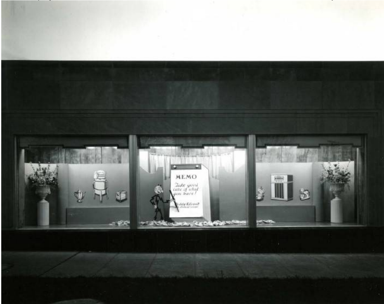
Potomac Electric Power Company Harrison Substation showing window displays ca. 1940s. (Photo from PEPCO)
