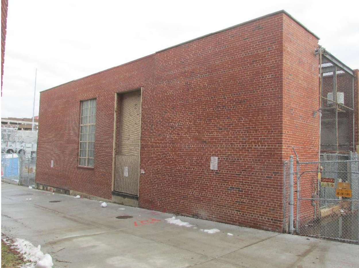
Pepco Harrison Street Substation
