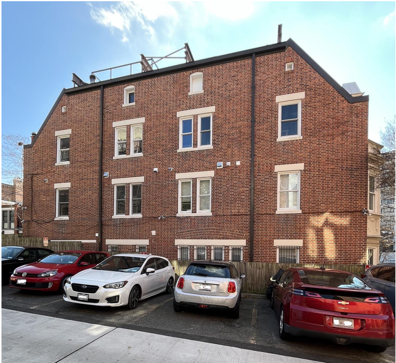
Photo 13: North elevation view from alley (J. DeFerrari).
