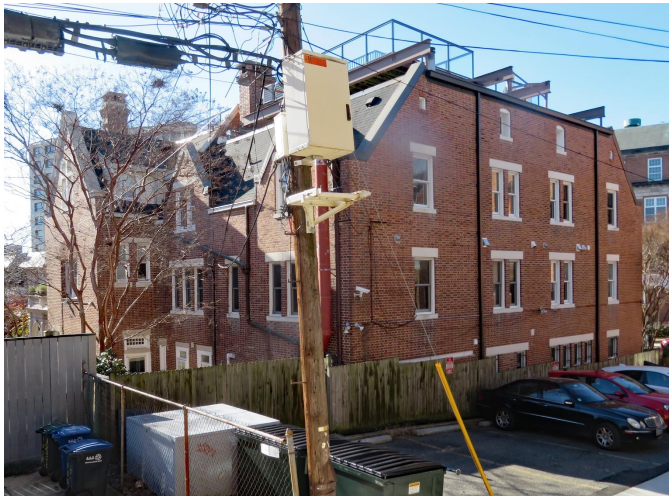
Photo 14: North and east elevations, view from alley (J. DeFerrari).
