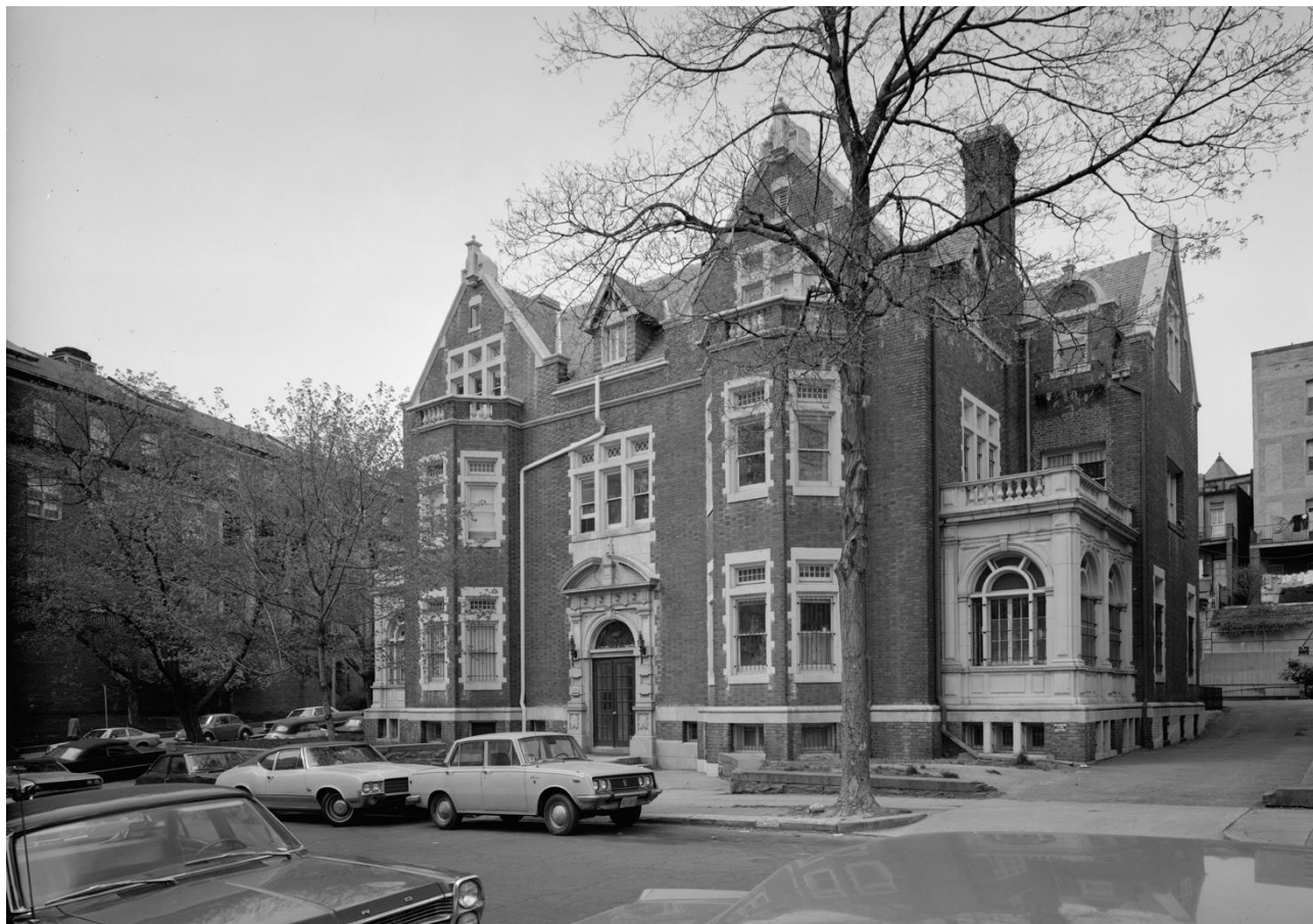
Photo 2: Old Chinese Legation, Front (south) Elevation from Vernon Street NW (Jack E. Boucher, HABS).
