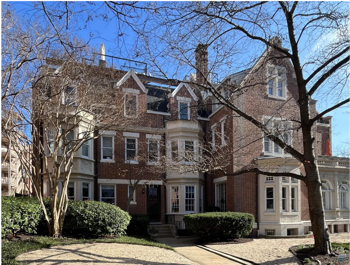
Photo 12: West elevation view from 19 th Street NW (J. DeFerrari).
