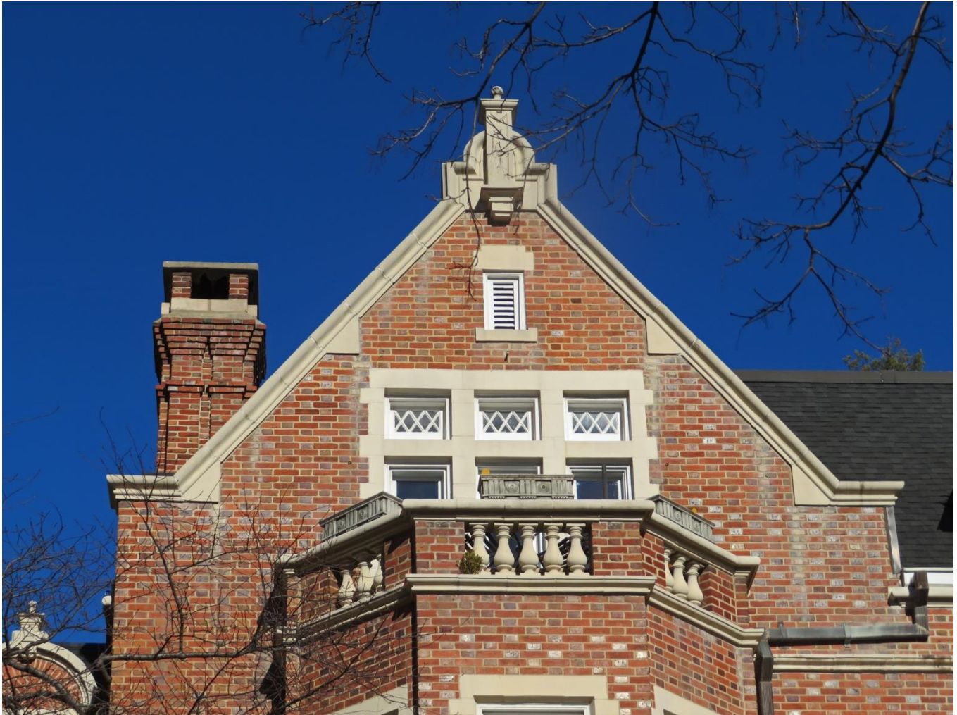
Photo 8: Detail of west gable parapet and balcony, front (south) elevation from Vernon Street NW (J. DeFerrari).
