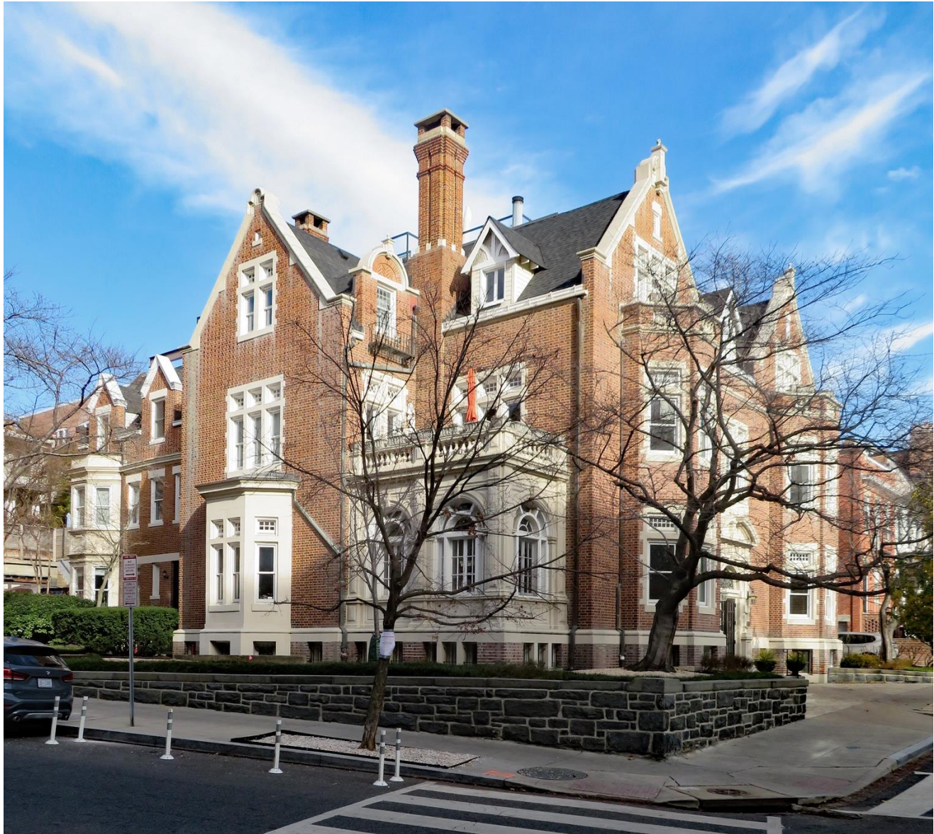
Photo 10: West elevation view from 19 th Street NW (J. DeFerrari).
