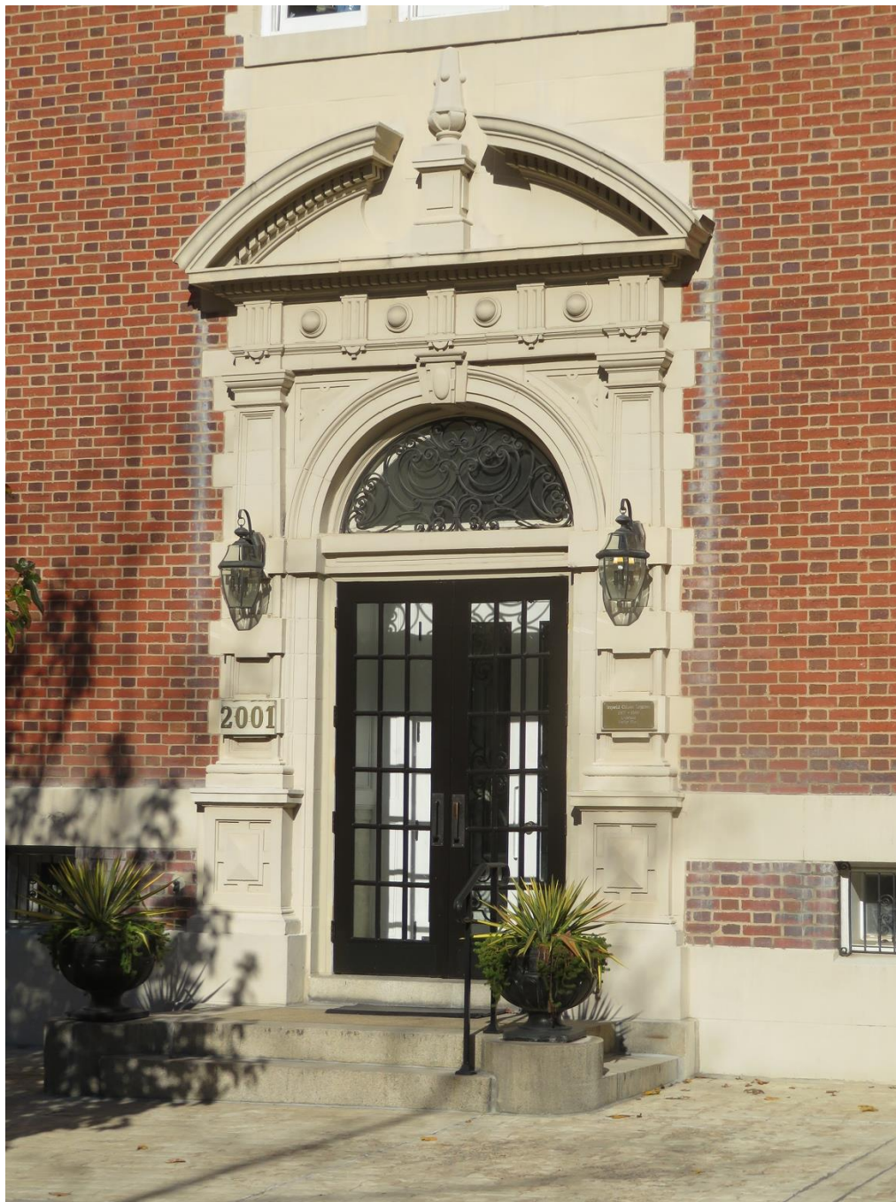
Photo 7: Main entrance on Vernon Street NW (J. DeFerrari).
