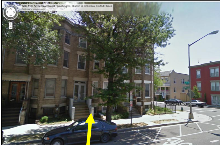
View of the subject block looking east across 11 th Street (Property identified); Google Streetview (2009 image)
