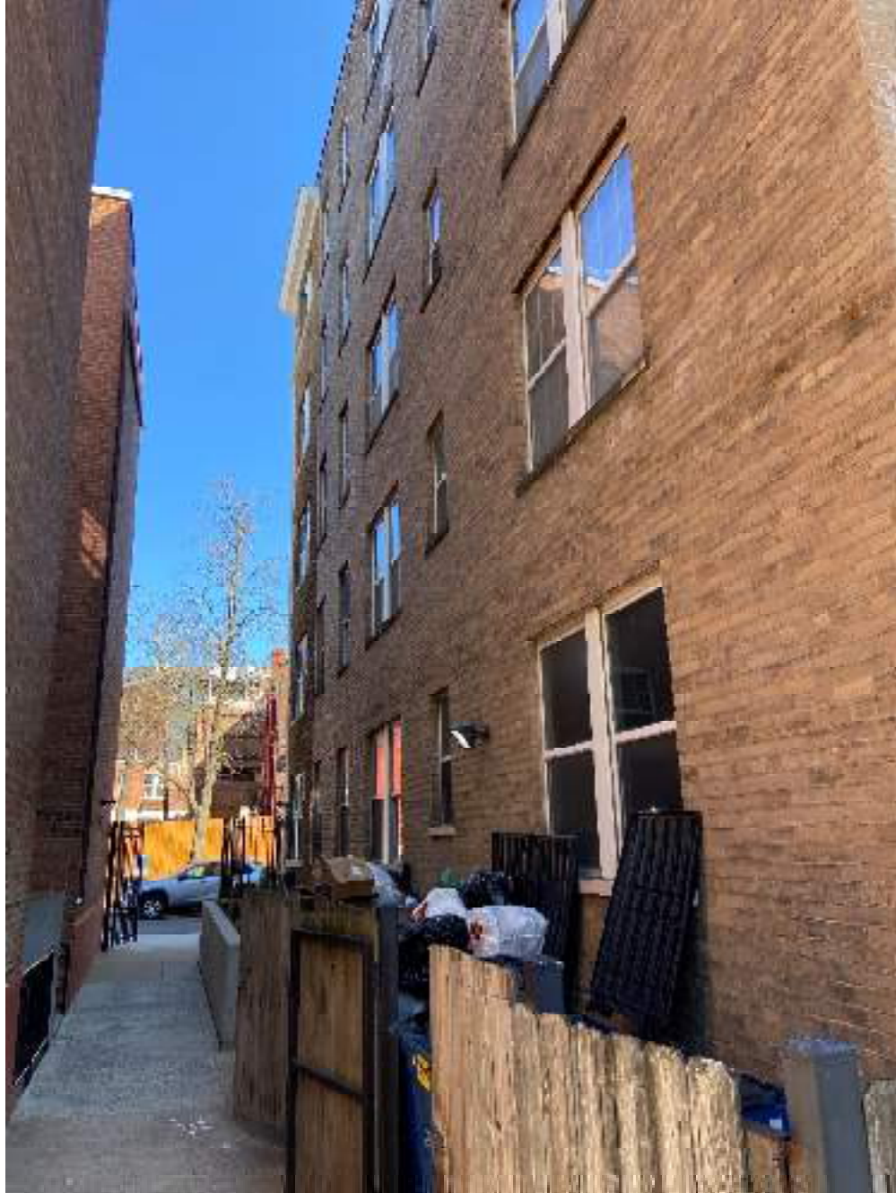
Photo #15 D.C._Washington_Mozart Apartments_0015 view of west elevation and gate, looking north
