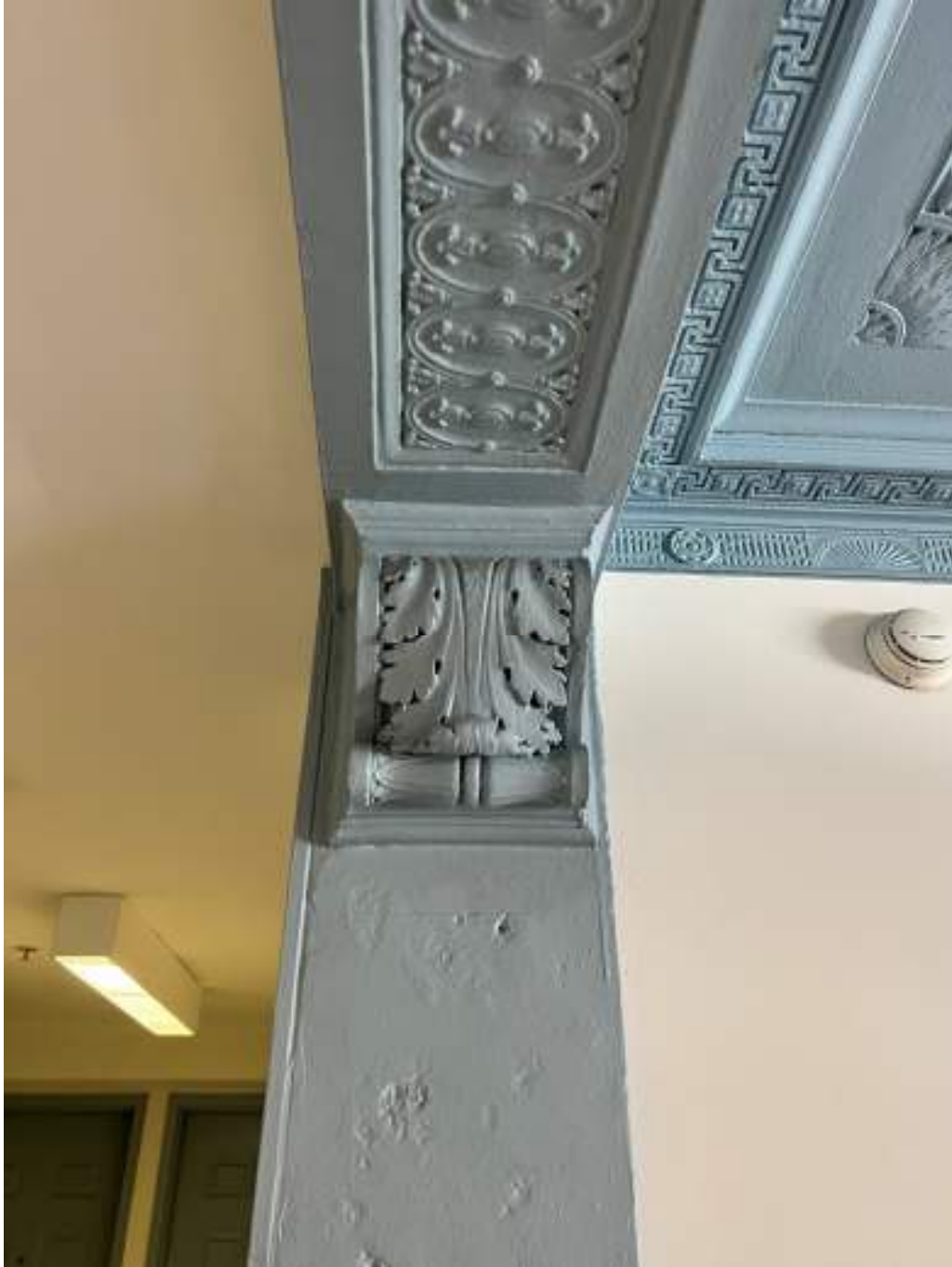
Photo #17 D.C._Washington_Mozart Apartments_0017 detail of lobby molding, looking west
