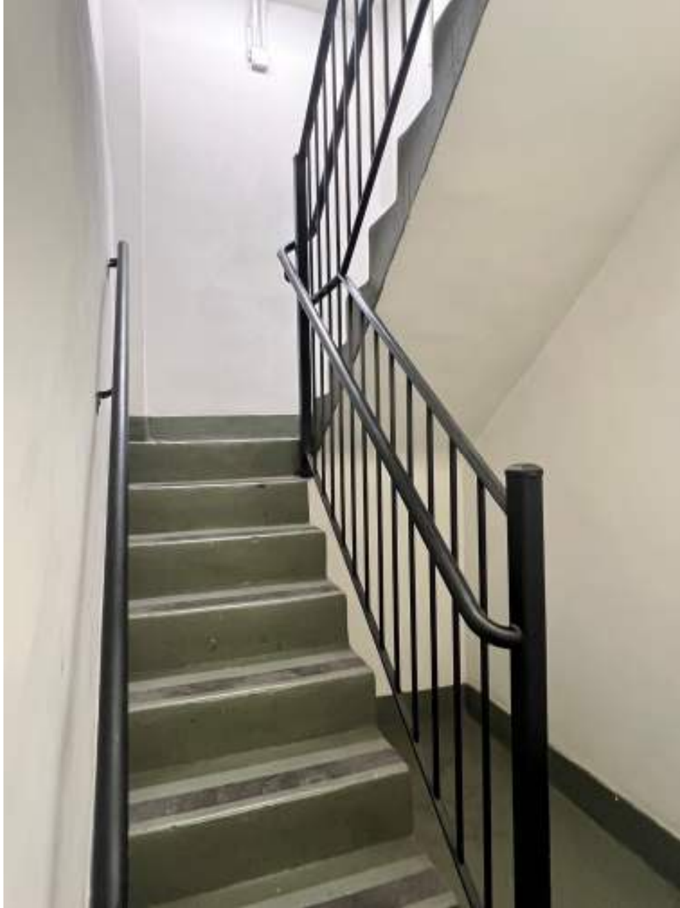
Photo #18 D.C._Washington_Mozart Apartments_0018 view of stairwell (typical), looking east
