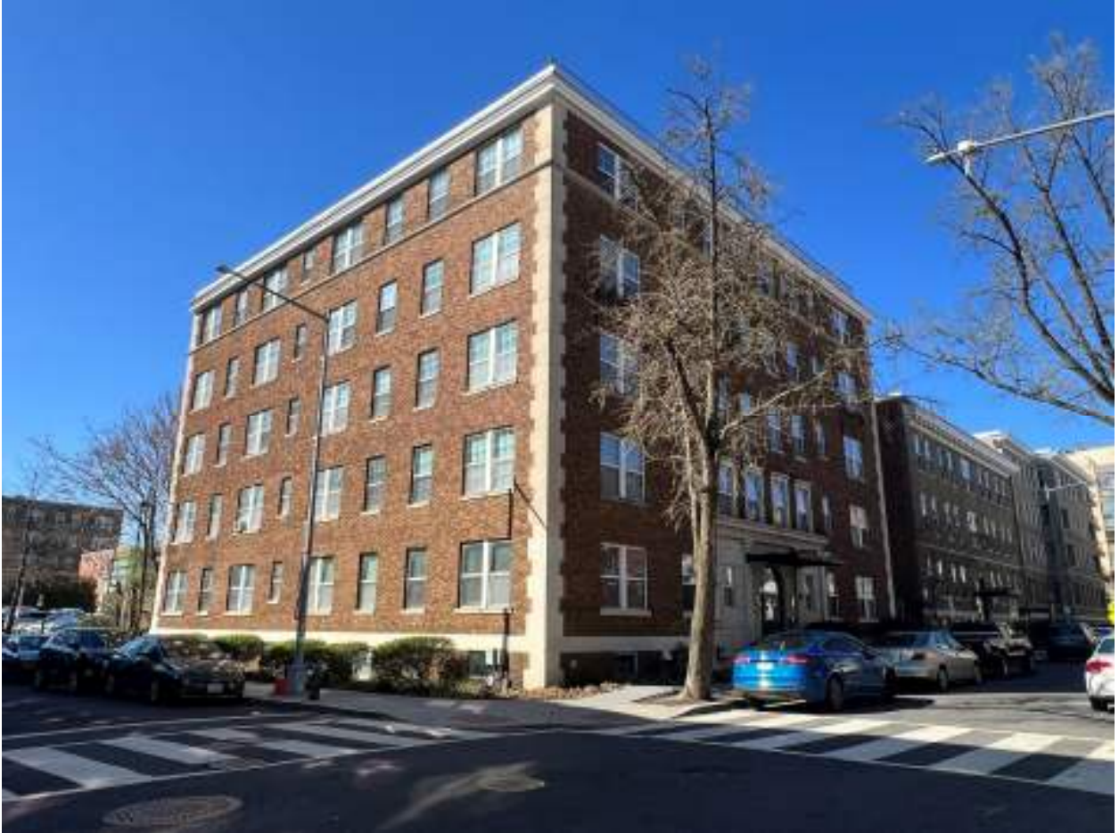
Photo #2 D.C._Washington_Mozart Apartments_0002 view of façade and elevation, looking southwest
