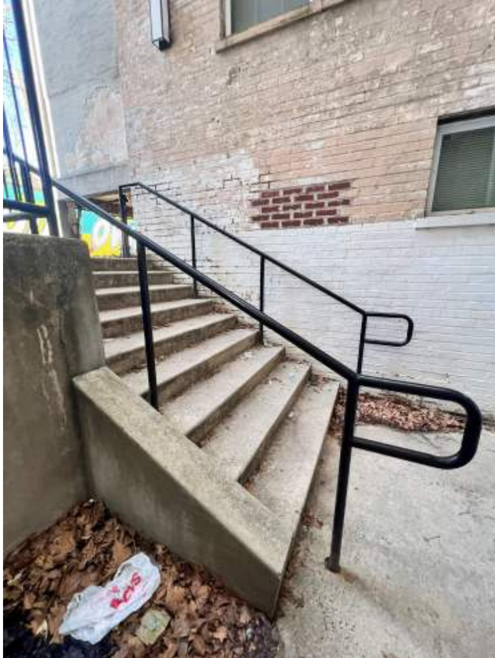
Photo #11 D.C._Washington_Mozart Apartments_0011 view of courtyard stair, looking southwest
