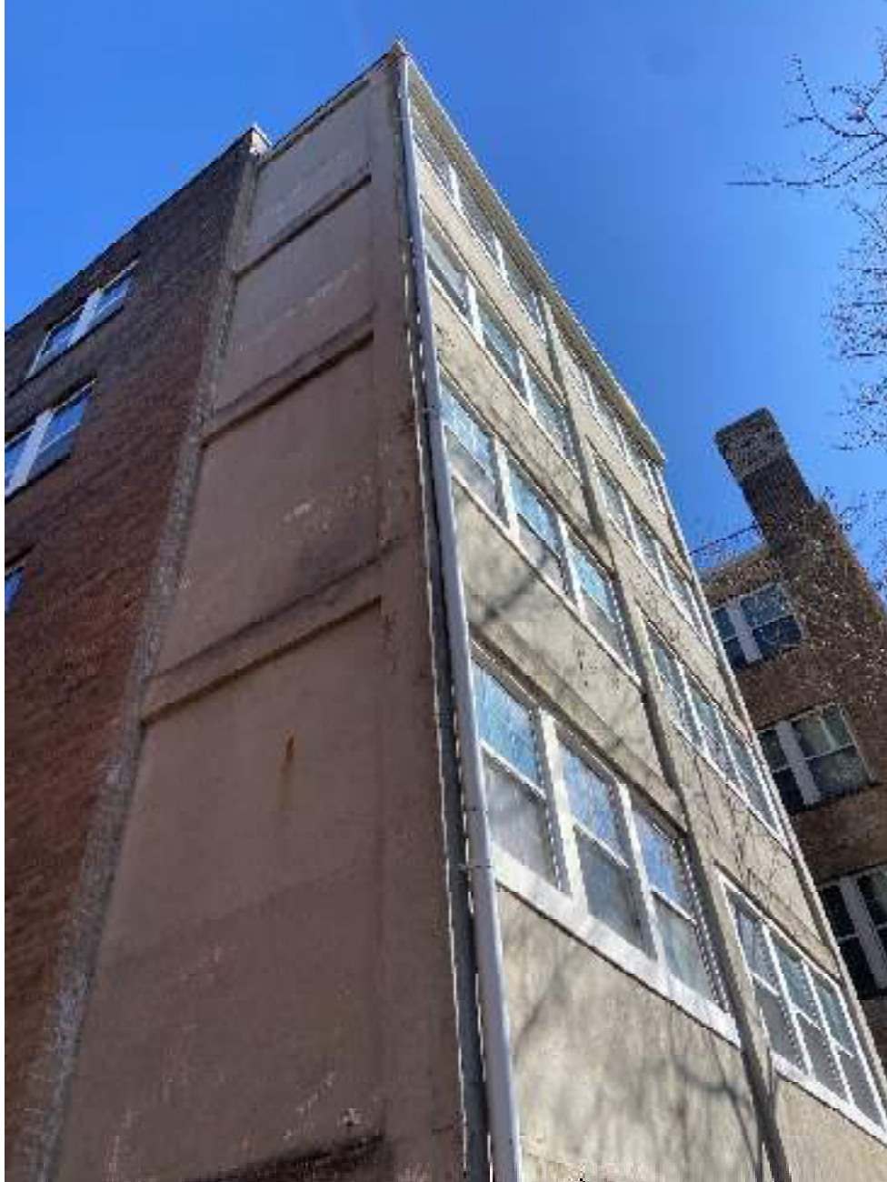
Photo #12 D.C._Washington_Mozart Apartments_0012 view of concrete historic porch enclosure, looking northeast
