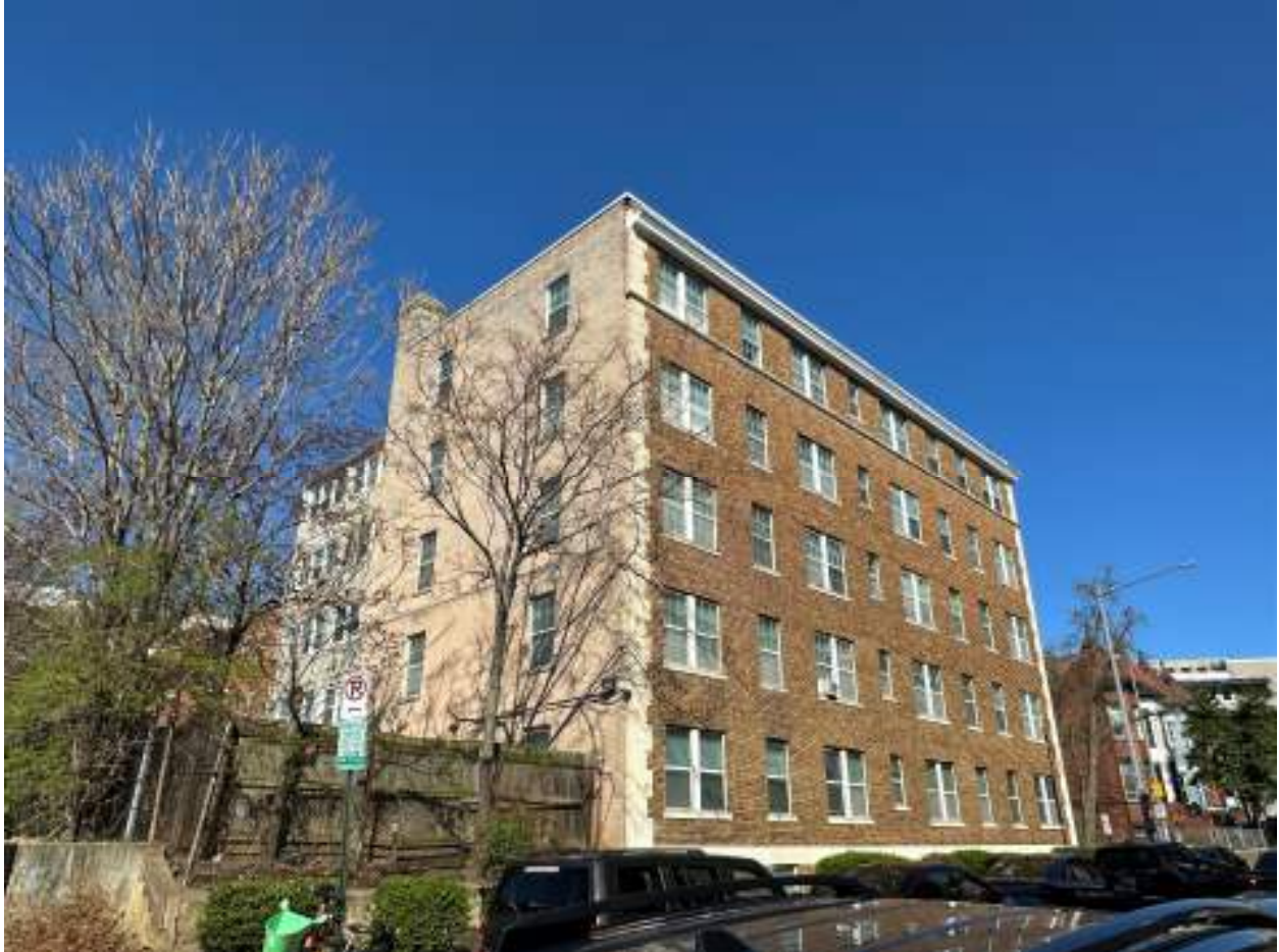
Photo #4 D.C._ Washington_ Mozart Apartments_0004 view of east and south elevations, looking northwest
