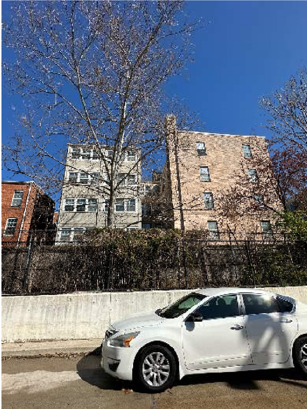
Photo #5 D.C. _Washington_Mozart Apartments_0005 view of south elevation, looking north
