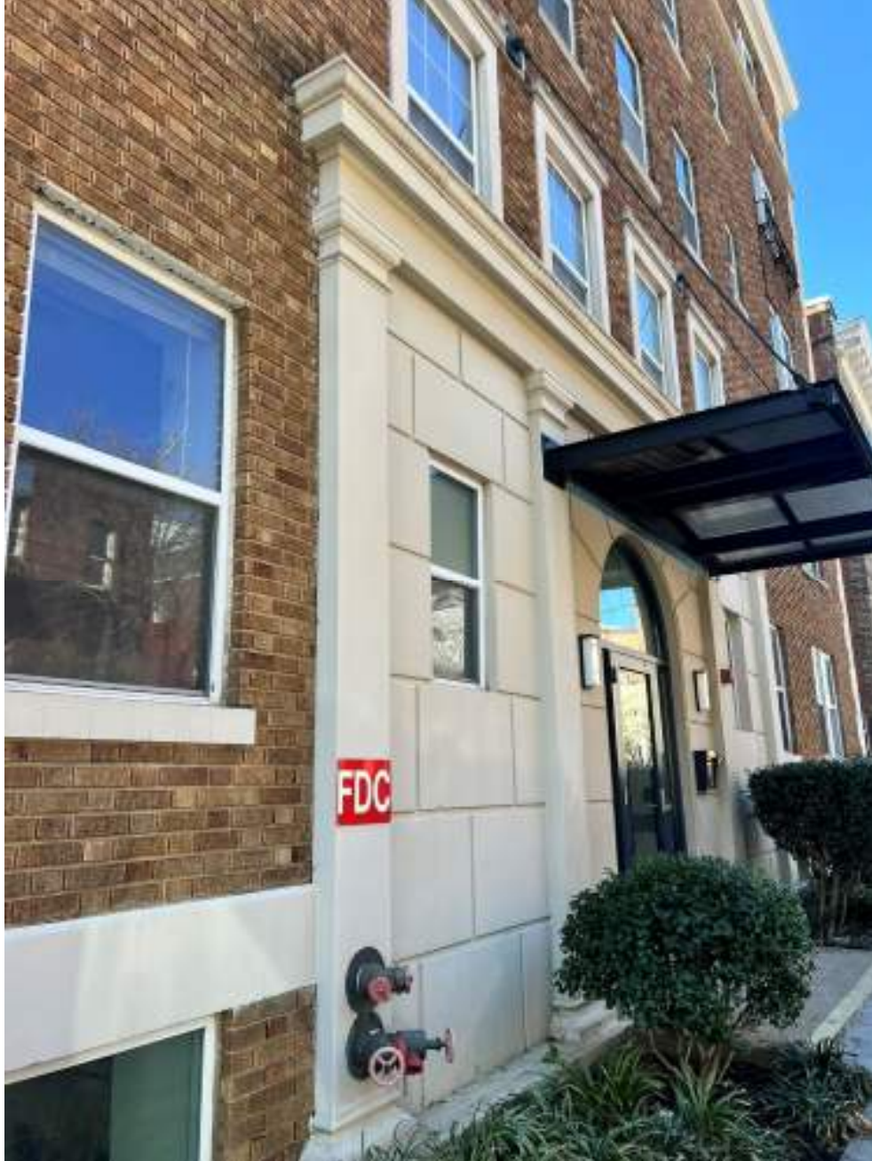
Photo #8 D.C._Washington_Mozart Apartments_0008 view of primary entrance and façade windows, looking west
