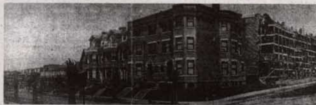
17th and Kilbourne Streets (1906). Construction scaffolding for row at right in place. Courtesy Martin Luther King, Jr. Library, Washingtoniana Collection.
