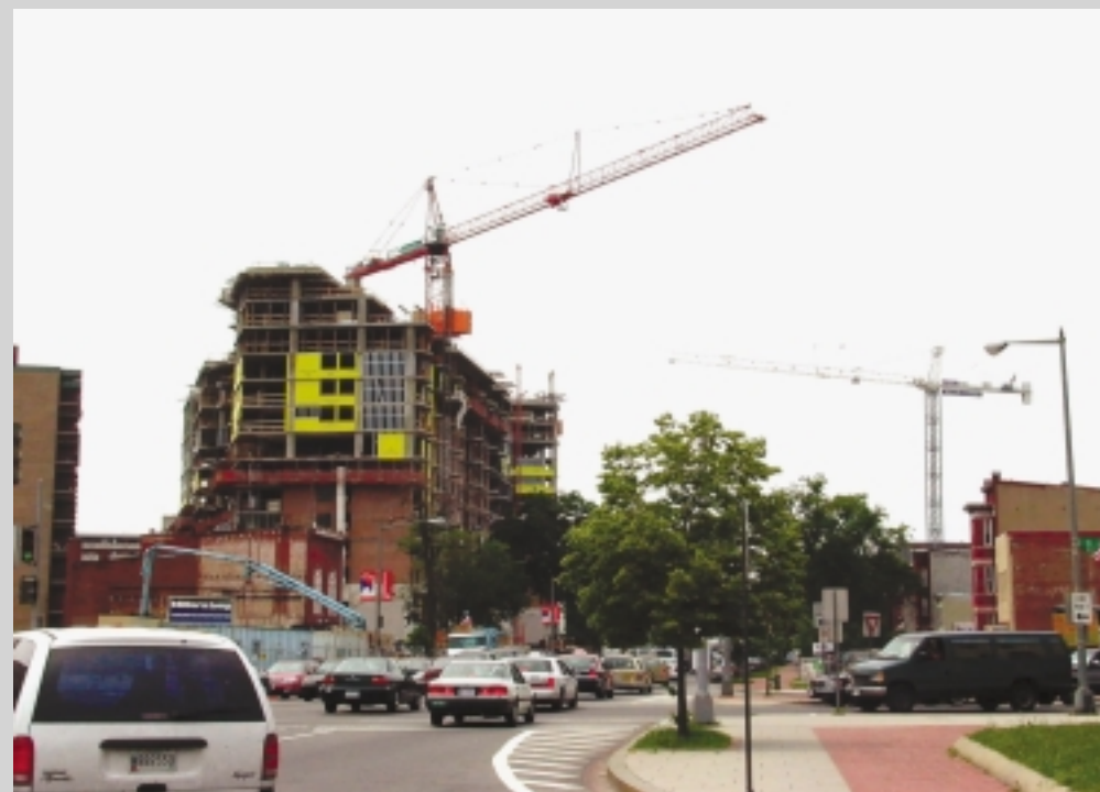
Additional residential construction on Massachusetts Avenue
