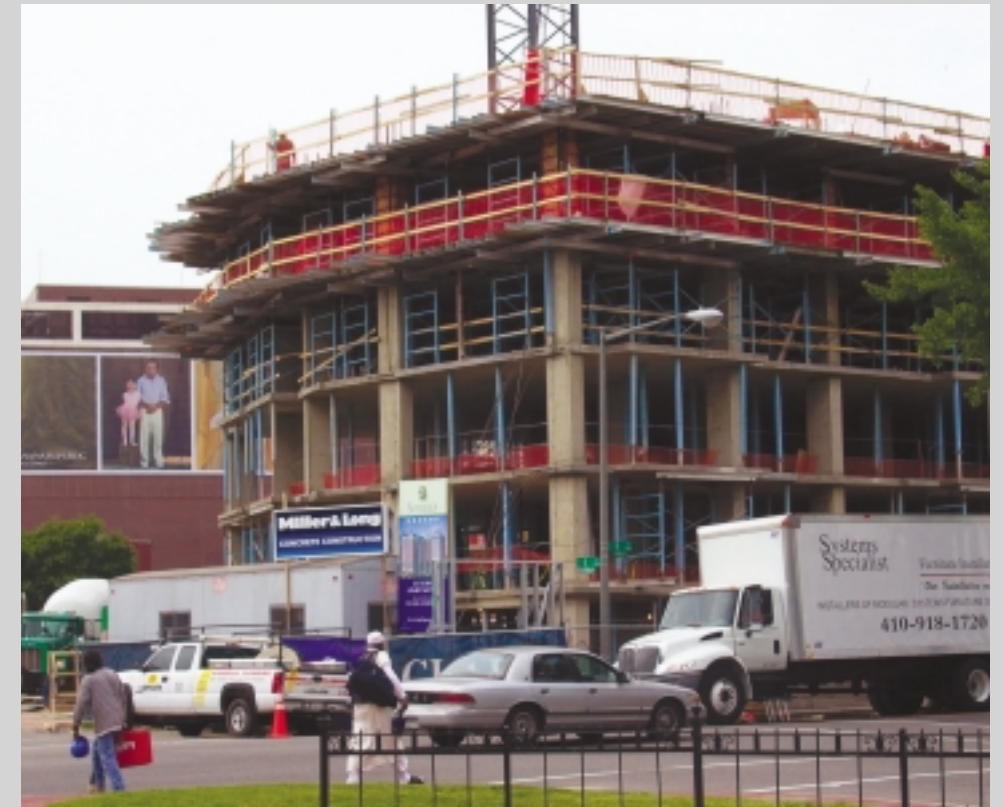
Sovereign Square, 246 apartments under construction at 5th Street and Massachusetts Avenue
