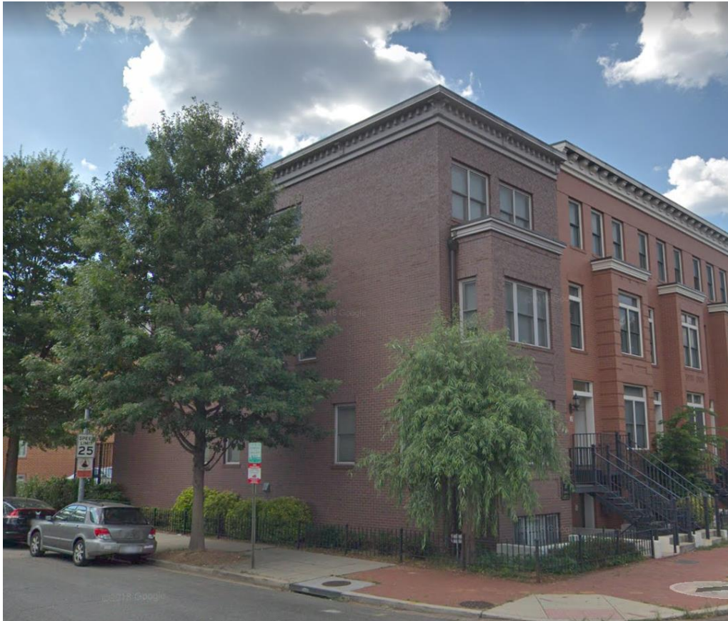
Figure 1. 1220 4 th Street NW (2010)
