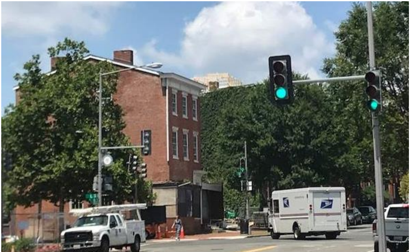
Photo 1: View of mock-up of roof addition from south
