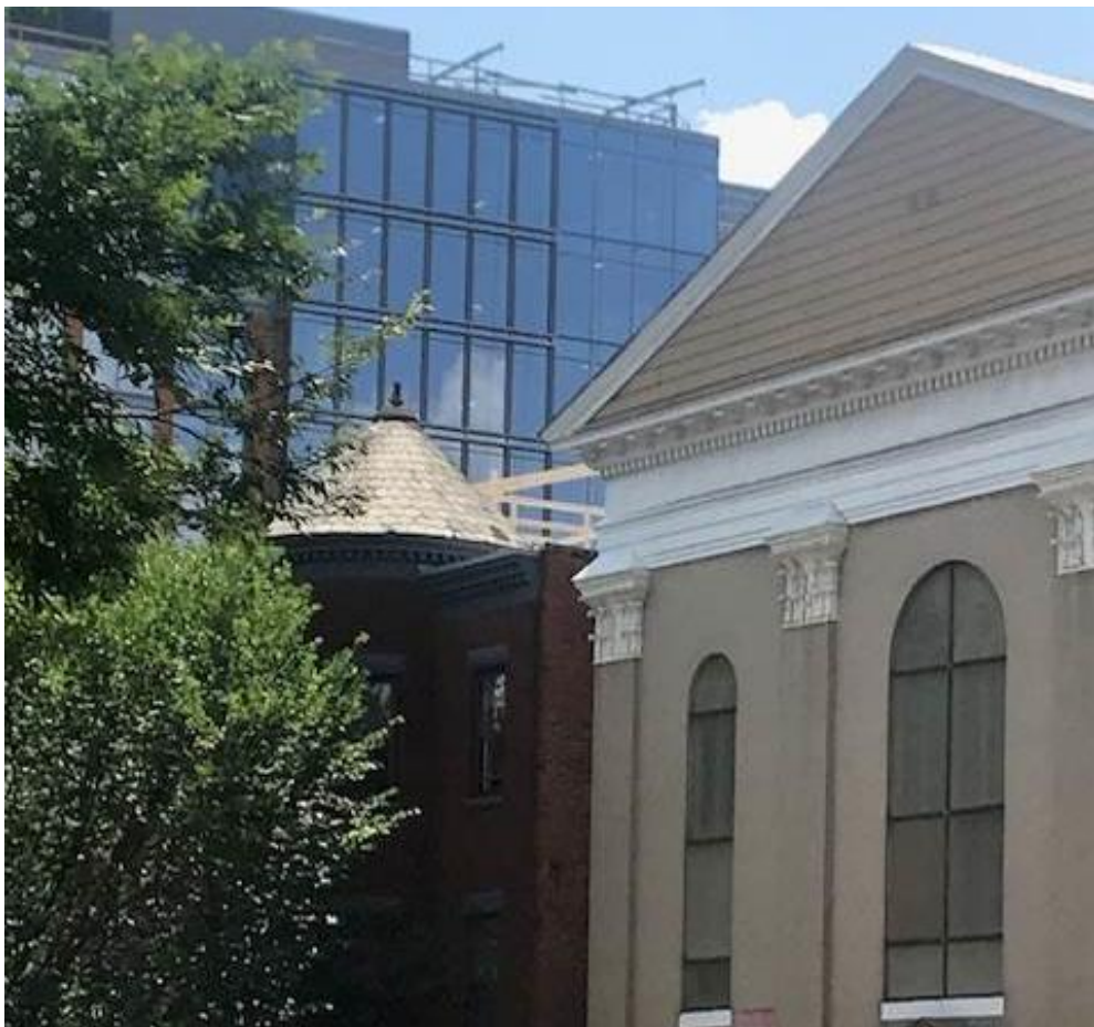
Photo 2: View of mock-up of roof addition from north
