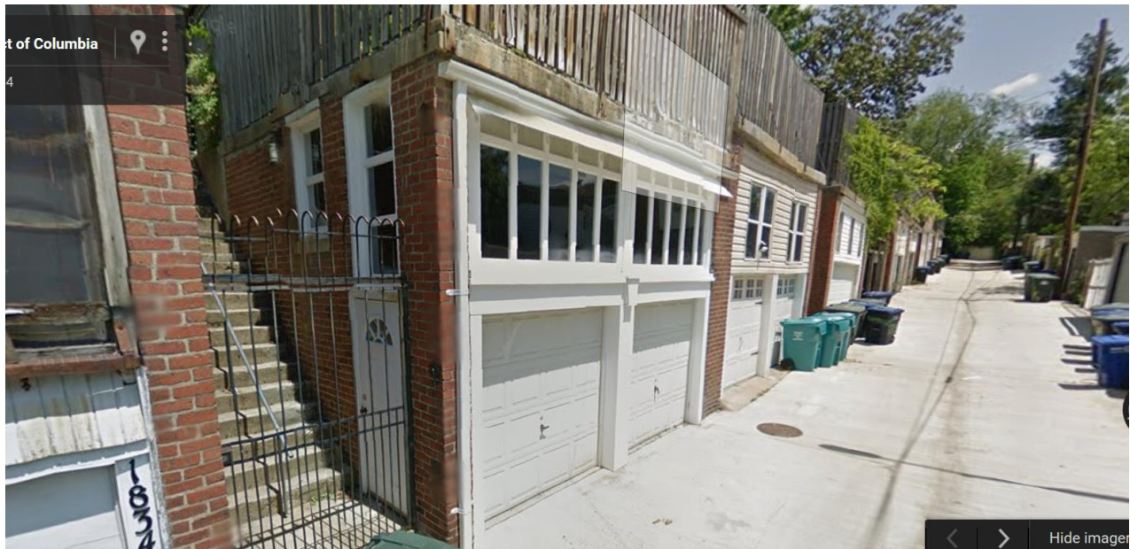
A Google Streetview photo of garages on the south side of the 1800 block of Lamont Street.
