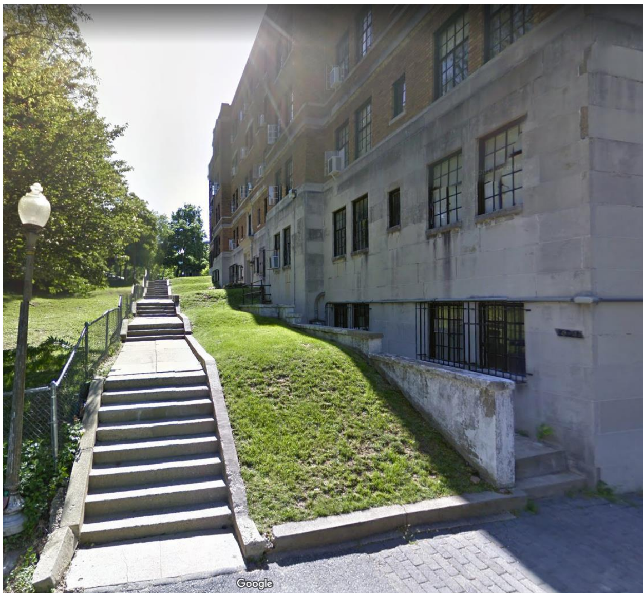
The cabinet would be located in the space between the two sets of basement windows seen here. The four conduits into the building would penetrate the masonry at about the height of the single existing one, seen at the inside corner of the building's projecting pavilion at the end of the areaway.
