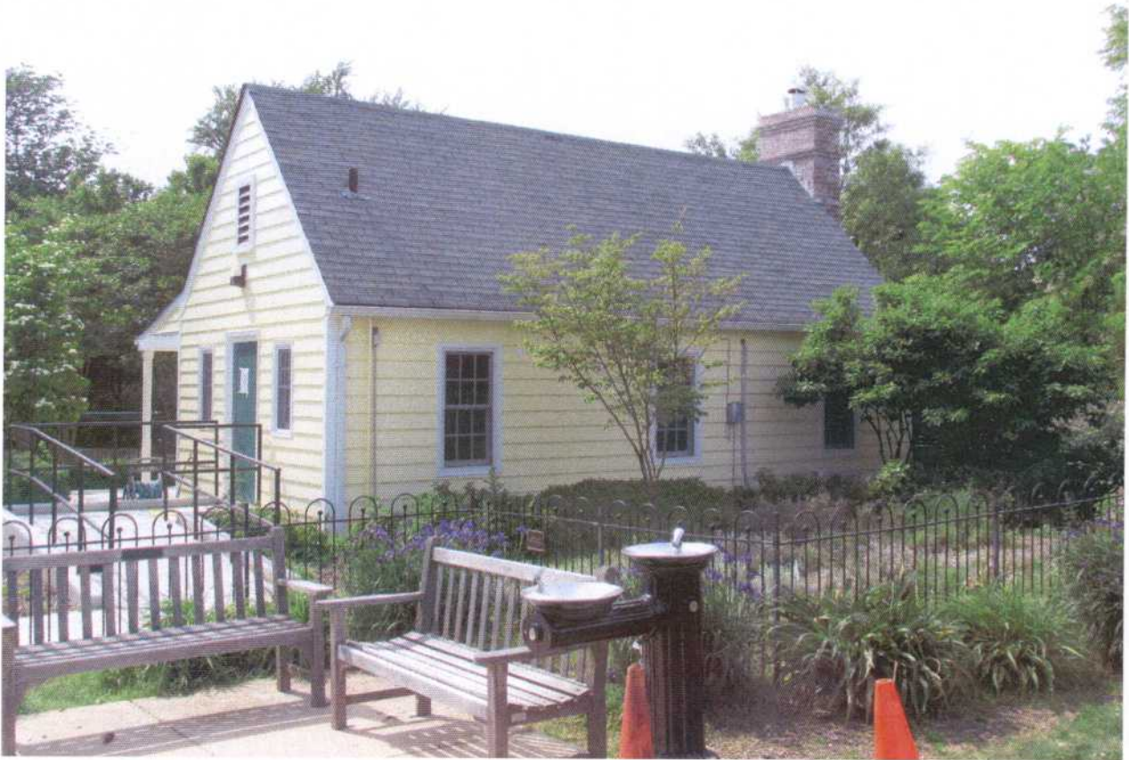
Mitchell Park Field House Washington, DC May 16, 2015 Kent Boese Field House, view from southeast 4/4
