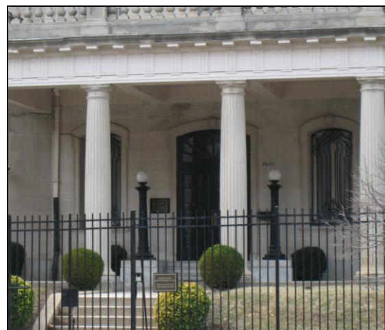
Distinctive light fixtures should be retained and repaired. While new fixtures do not have to replicate originals, they should be in proportional in scale and appropriate in coloration with the building.
