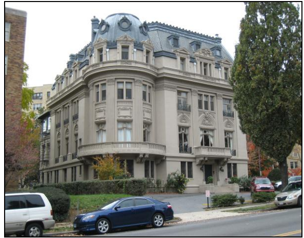
The mansard roof on the former French Embassy at 2460 16 th Street includes slate shingles, copper cresting and a metal-clad tower with oculus windows.
