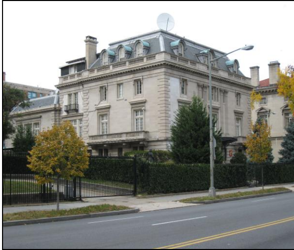
Locating this satellite dish further back from the street, or on the rear wing, would have minimized its visual impact and not interfered with the profile and appearance of the building's roofline.
