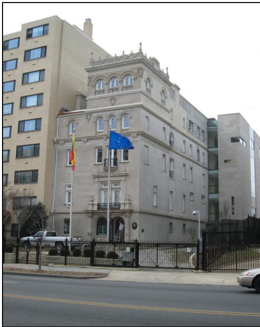
The modern apartment building abutting this mansion overwhelms the historic building. In contrast, the rear addition, although clearly contemporary, is appropriately scaled, subordinate in size, and compatible in coloration and materials.
