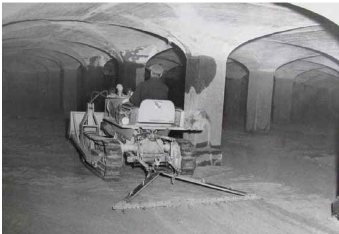
Tractor and filter rake pulverizing the filter sand surface and filter operation (c. 1944)
