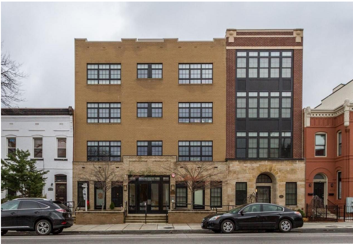
Three-story roof additions, 1511 and 1515 11 th Street NW
