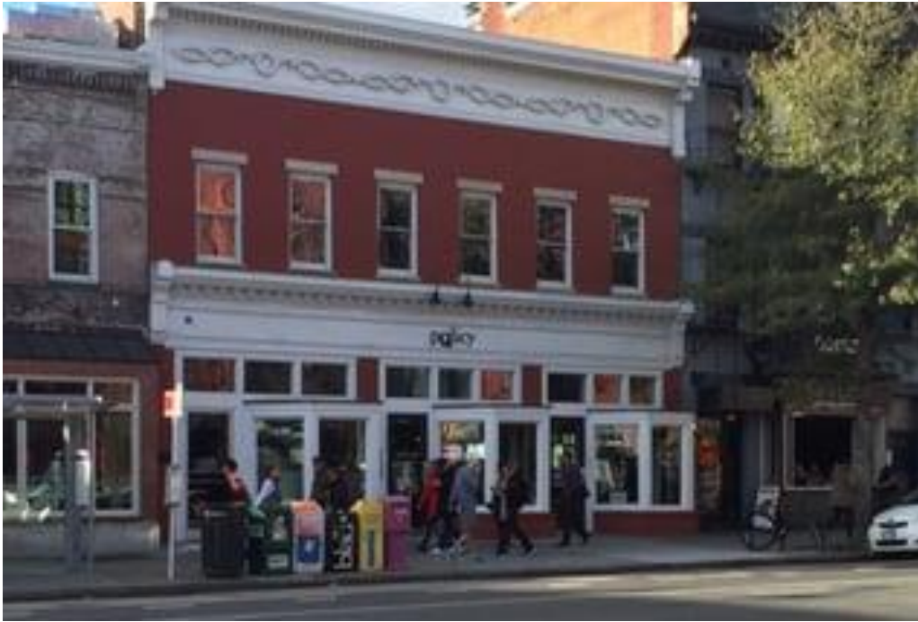
One-story roof addition, 1902-1906 14 th Street NW
