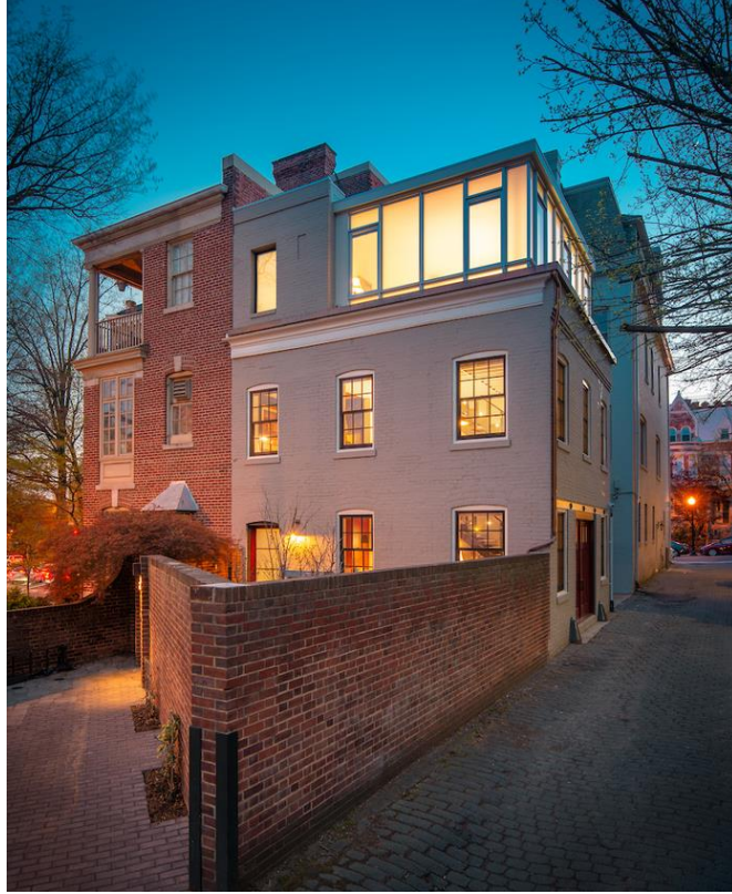
One-story roof addition, 2161 Florida Avenue NW
