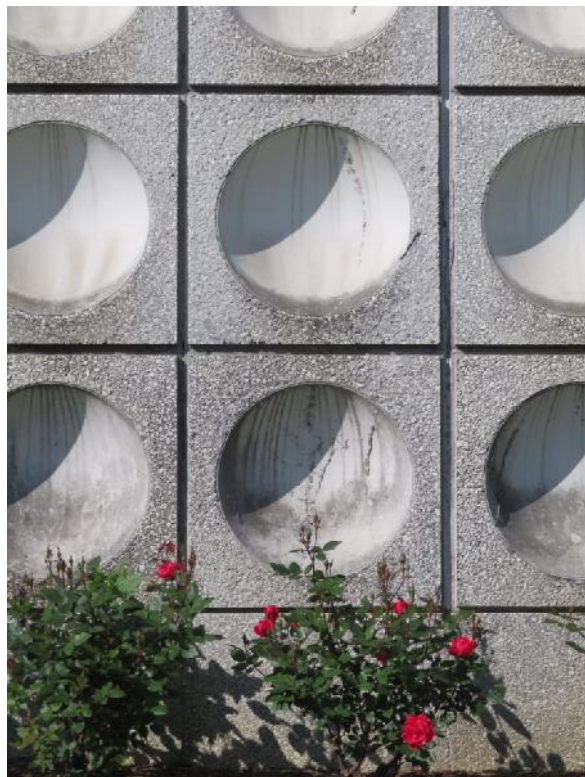
Detail of an array of sculpted concrete dimples from the building's north elevation.
