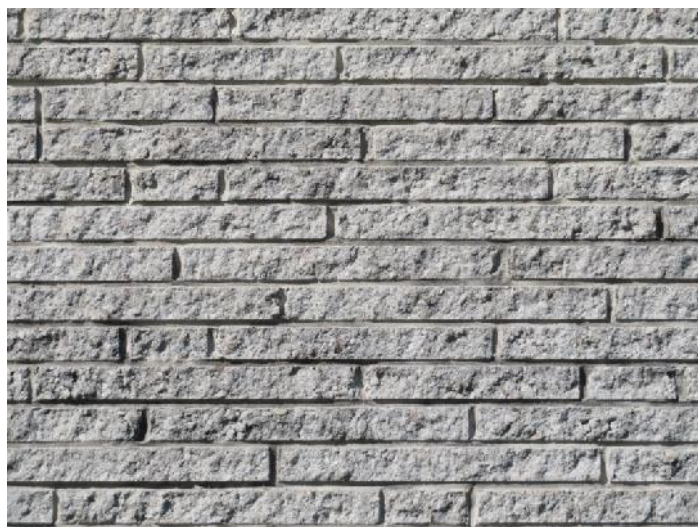
Detail of the rusticated roman brick used on the building's principal elevations.
