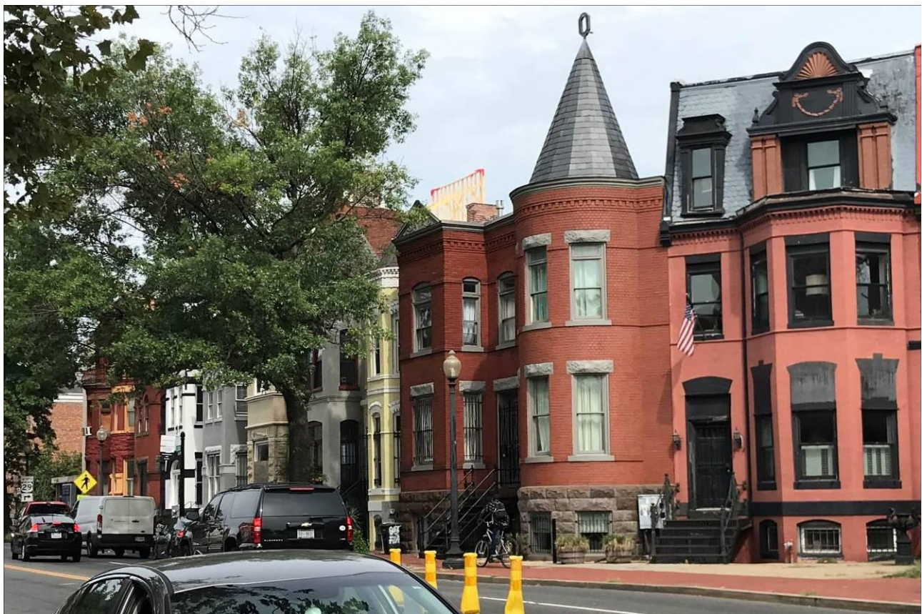
Figure 1. Flag test mock-up of front façade of proposed fourth floor, August 31, 2021.
